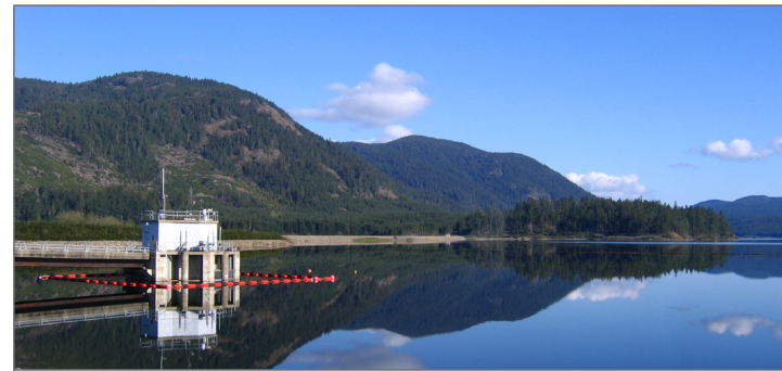
Water Supply Intake at Sooke Lake Reservoir
