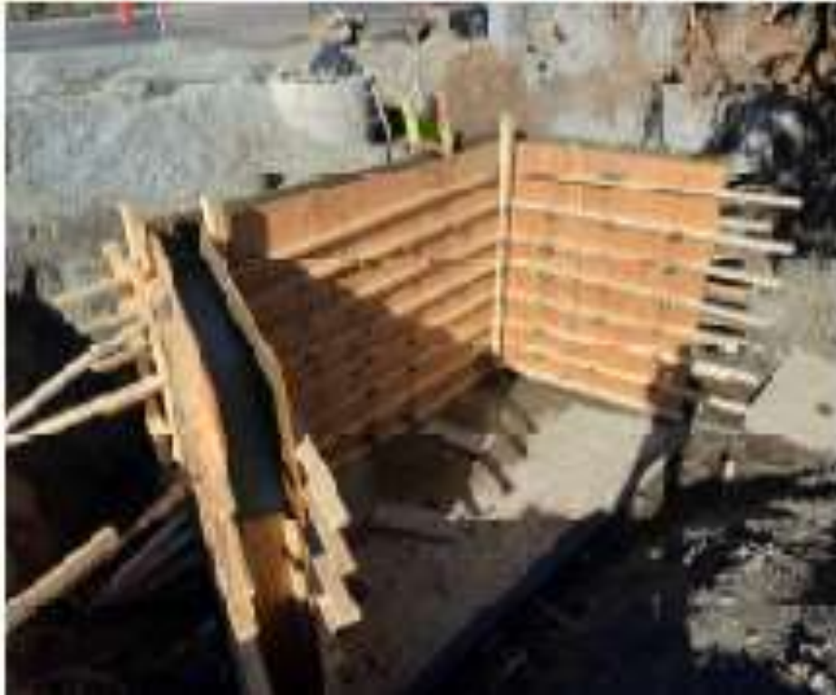
Figure 15–Residual Solids Pipes – Peers Creek – Forming east side headwall.
