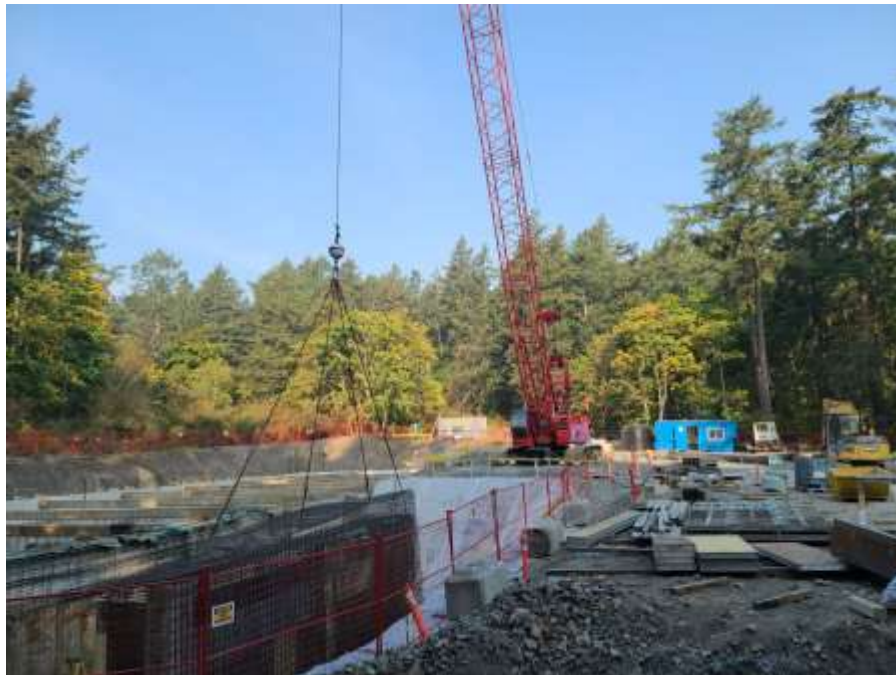
Figure 19–Arbutus Attenuation Tank- Valve chamber wall reinforcing steel installation.
