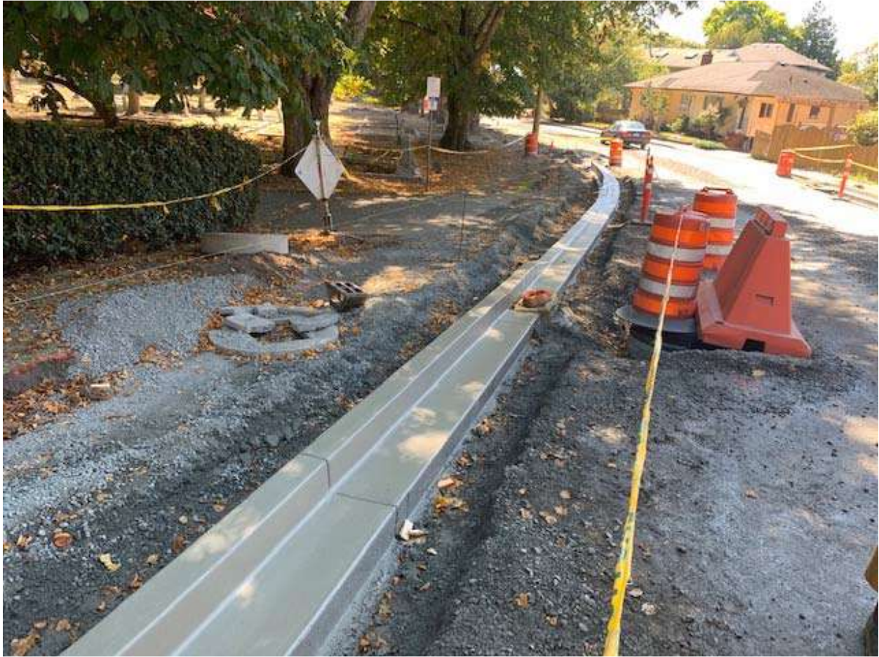
Figure 20–Trent Forcemain- Curb work completed on Memorial Crescent.
