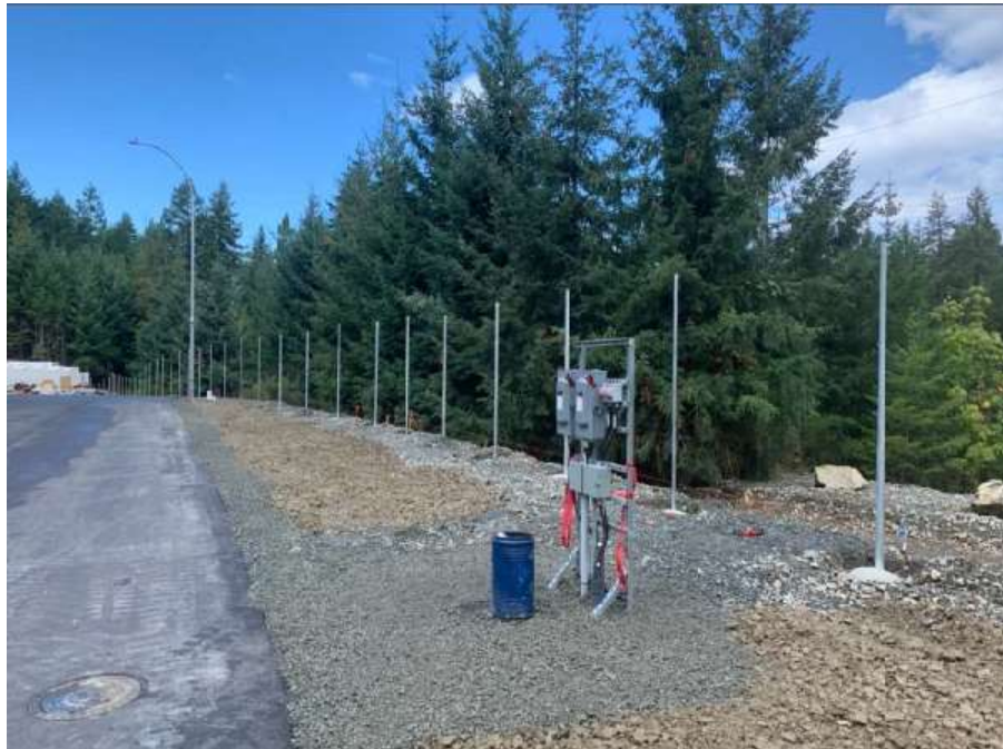
Figure 7- Residuals Treatment Facility- Ongoing installation of site perimeter fencing.
