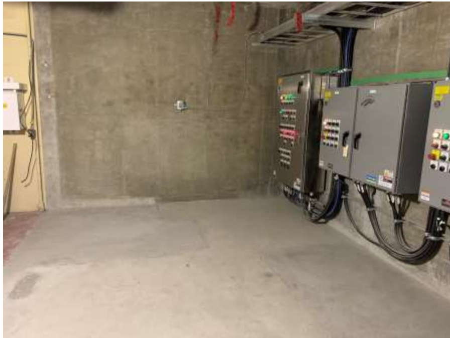
Figure 10- Clover Point Pump Station – Control room concrete slab infills.
