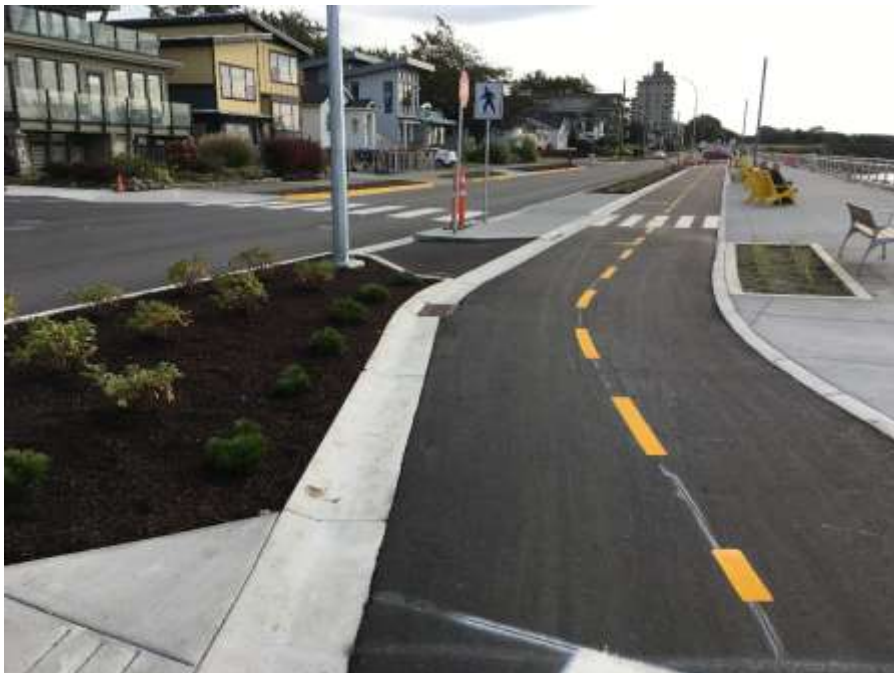
Figure 13–Clover Forcemain- Cycle track and Dallas Road paving complete.
