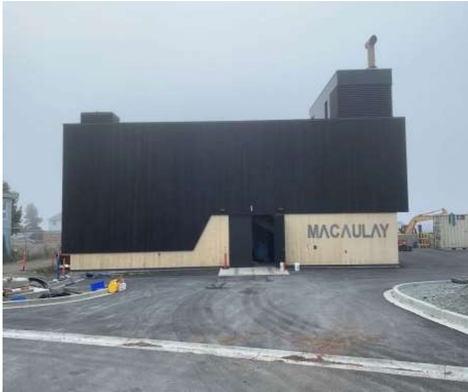
Figure 11—Macaulay Point Pump Station- Macaulay signage installed.
