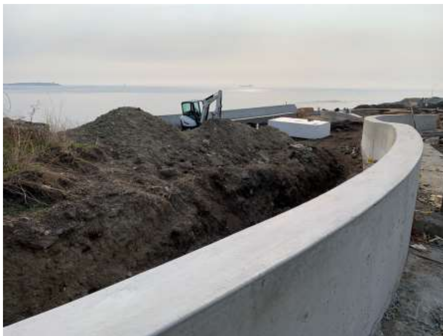
Figure 9–Clover Point Pump Station- Concrete pour of north retaining wall.
