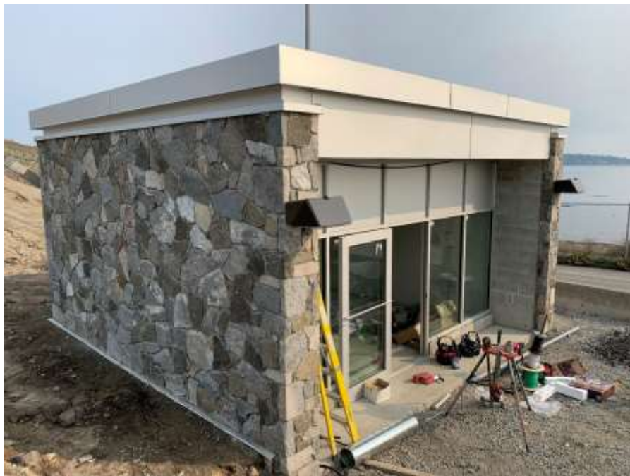
Figure 8–Clover Point Pump Station- Exterior of public washroom.
