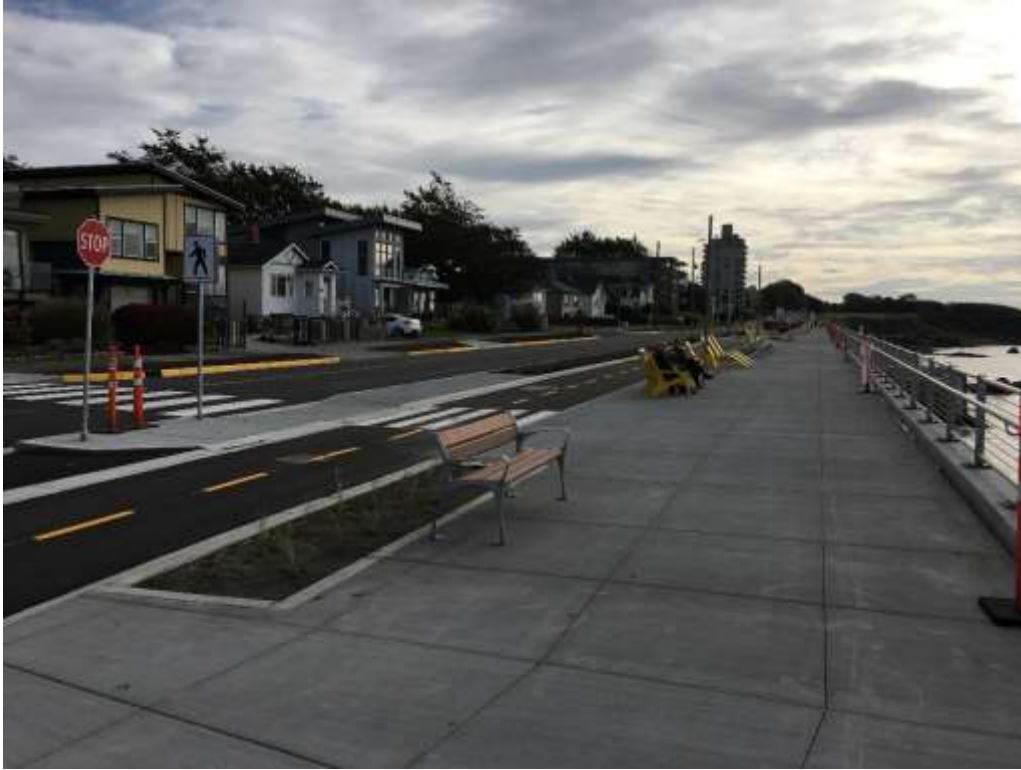
Figure 14–Clover Forcemain- Sidewalk complete with benches and lounge chairs.
