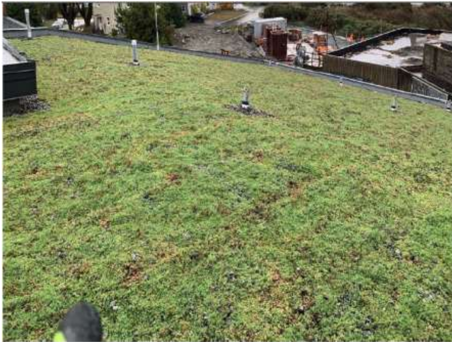
Figure 12—Macaulay Point Pump Station- Green roof complete.
