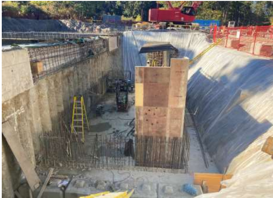
Figure 18–Arbutus Attenuation Tank- Valve chamber wall formwork installed.
