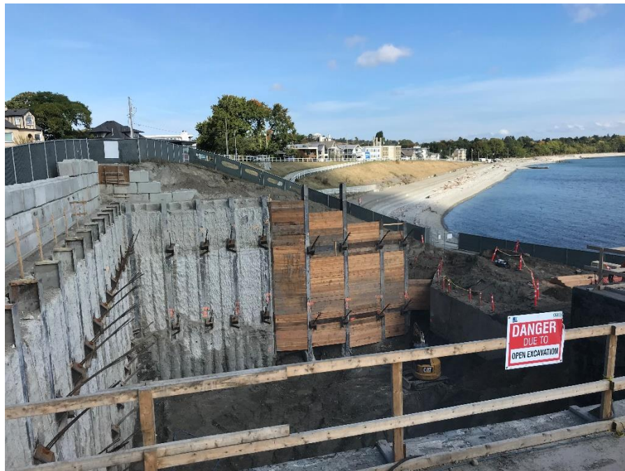
Figure 11 – Clover Point Pump Station: Completed tie-back installation.
