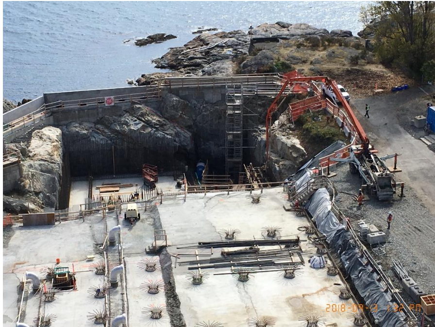
Figure 4 - McLoughlin Point Wastewater Treatment Plant: Placing concrete in tertiary wall.
