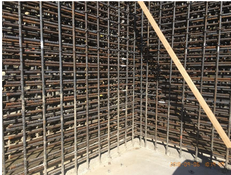
Figure 2 – McLoughlin Point Wastewater Treatment Plant: Installation of tertiary wall reinforcing steel.
