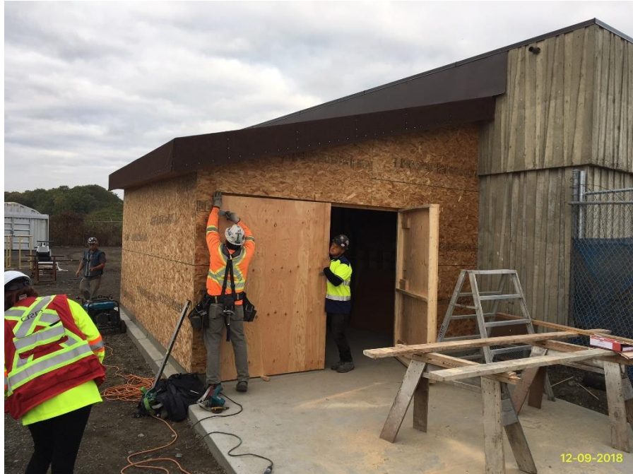
Figure 14 – Macaulay Point Pump Station: Construction of temporary bin room.
