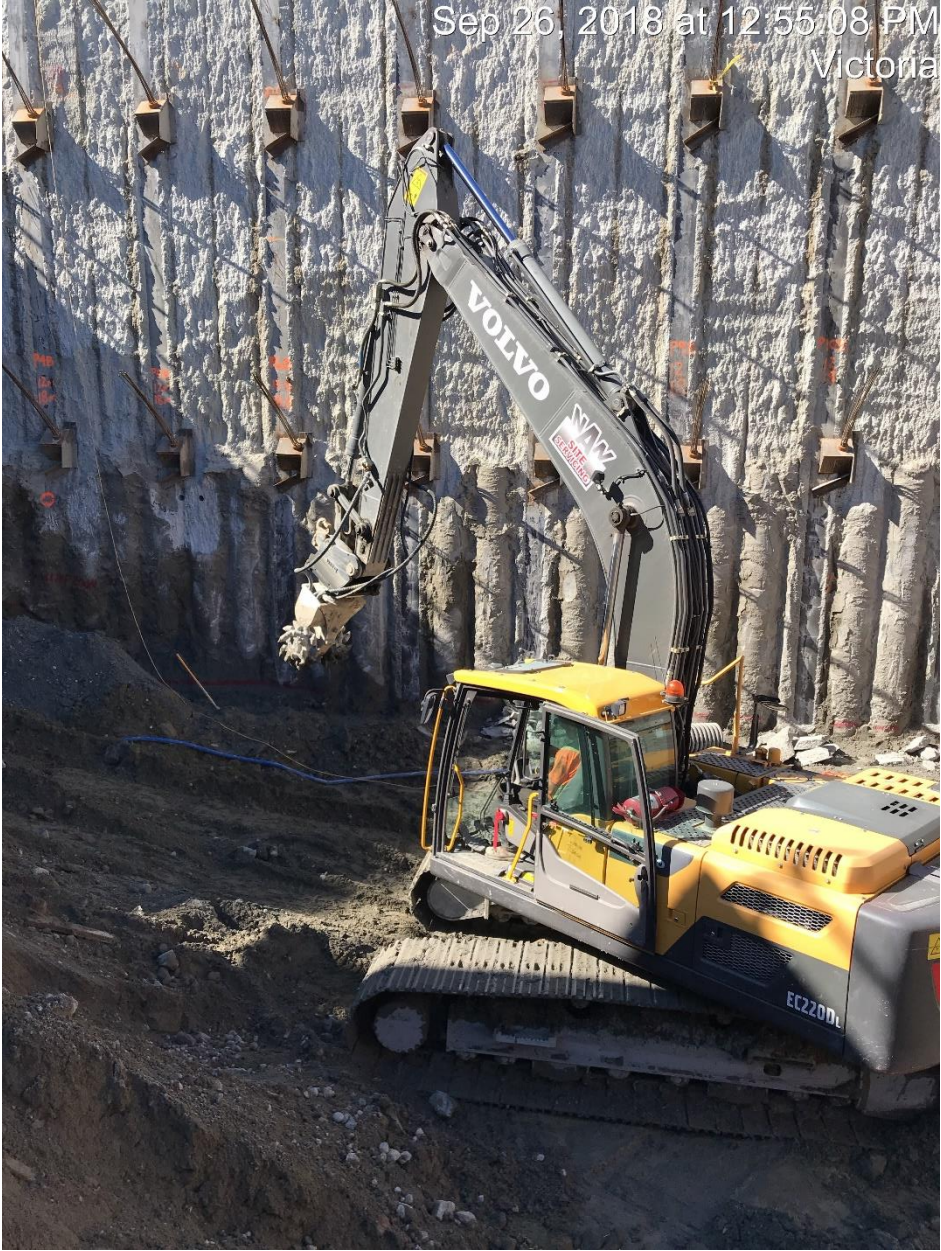
Figure 13 – Clover Point Pump Station: Grinding concrete flush at caisson wall.
