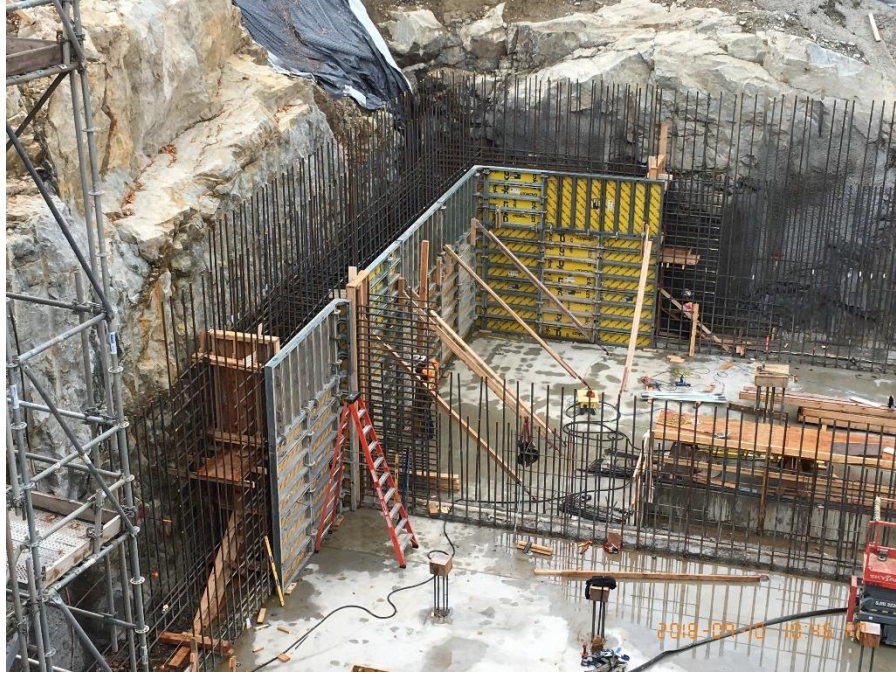
Figure 3 - McLoughlin Point Wastewater Treatment Plant: Installation of tertiary wall formwork.
