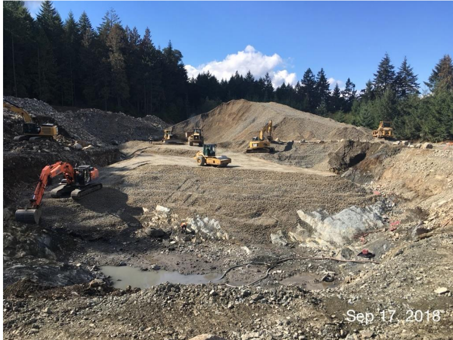
Figure 10 – Residuals Treatment Facility: Placing, spreading and compacting aggregate.
