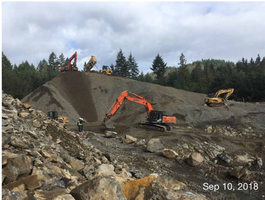
Figure 9 – Residuals Treatment Facility: Stockpiling crushed aggregate.
