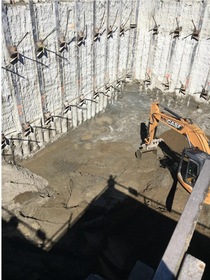
Figure 12 – Clover Point Pump Station: Excavating to base slab elevation.
