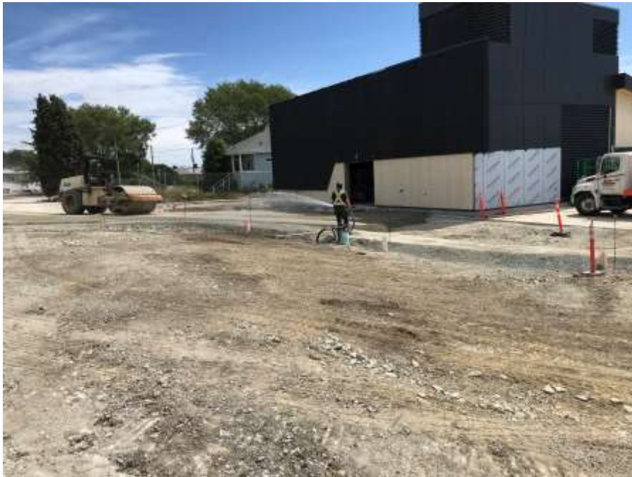
Figure 12—Macaulay Point Pump Station- Grading and prep for concrete curbs.
