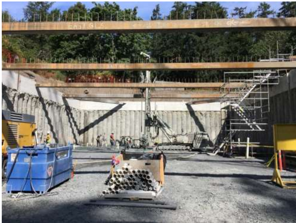
Figure 20–Arbutus Attenuation Tank- Inside the tank excavation looking north.
