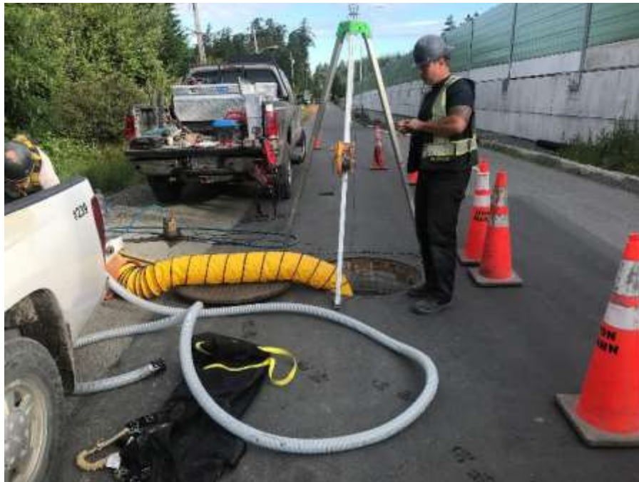
Figure 16- Residual Solids Pipes- Grouting low point drain valve at Portage Road.
