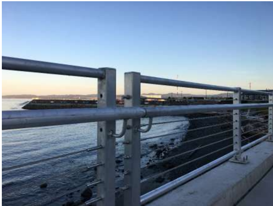
Figure 15–Clover Forcemain- New aluminium railing looking west from Oswego Street.
