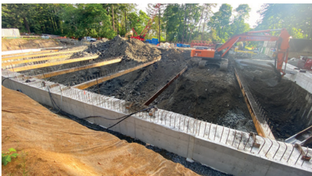
Excavation at the Arbutus Attenuation Tank.
