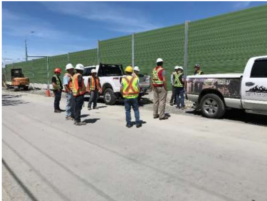
Figure 17-Residual Solids Pipes - Pre-paving meeting at Portage Road.
