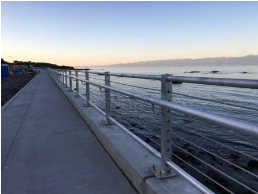
Figure 14–Clover Forcemain- New aluminium railing installed looking east from Oswego Street.
