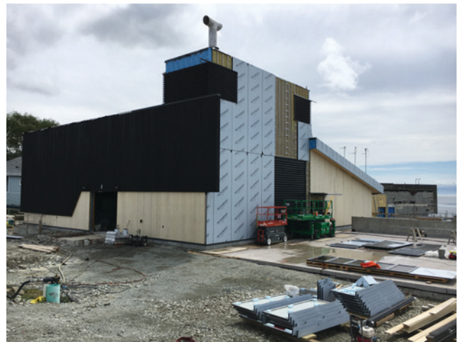
Siding being installed on the new Macaulay Point Pump Station.
