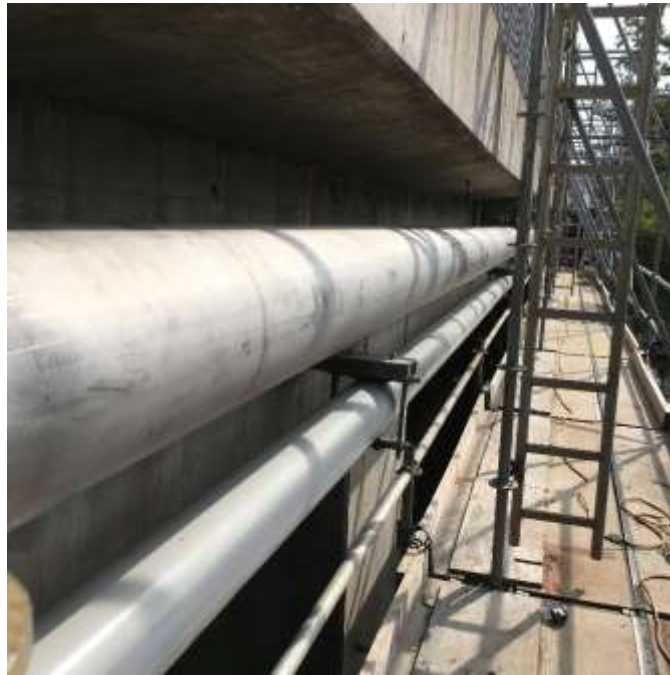
Figure 18–Residual Solids Pump Stations– Admirals Bridge –Installing pipe under Admirals Bridge
