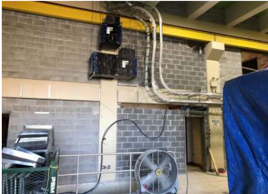
Figure 9–Clover Point Pump Station- New masonry walls in the generator room.
