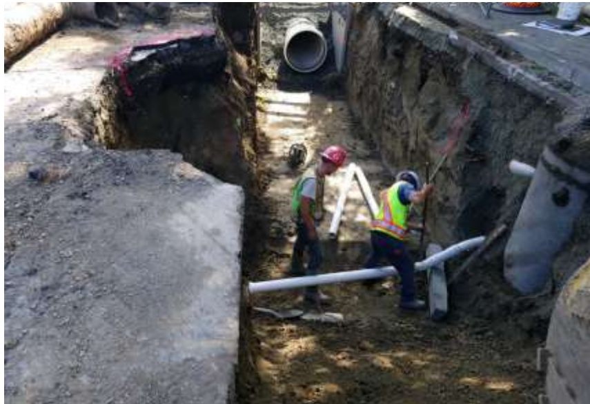
Figure 21- Trent Forcemain – Stannard Avenue – Realignment of sanitary service at Fairfield Road.
