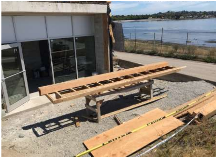
Figure 11- Clover Point Pump Station – Public washroom roof formwork installation.
