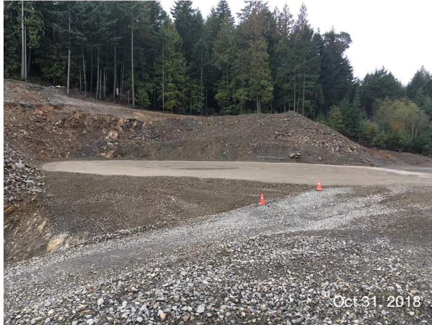
Figure 9 – Residuals Treatment Facility: Filling, grading and compacting complete at digester #2 site.
