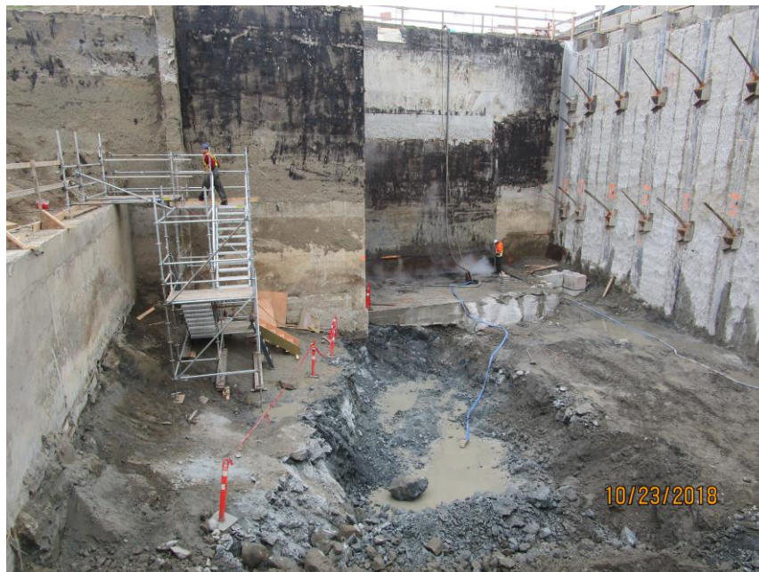
Figure 17 – Clover Point Pump Station: Installation of scaffolding access tower.
