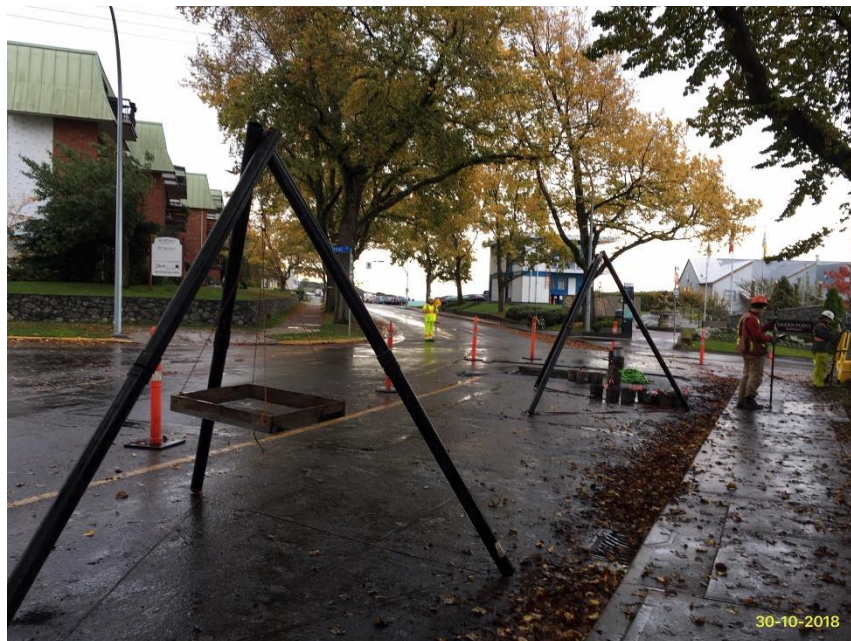
Figure 21 – Clover Forcemain: Pre-construction archaeological test dig.
