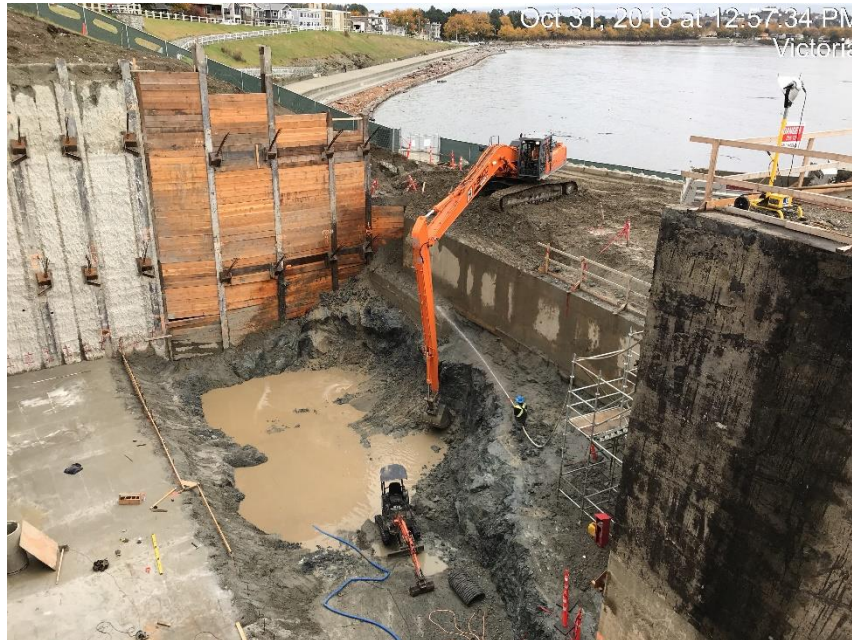
Figure 13 – Clover Point Pump Station: Excavation to final grade.
