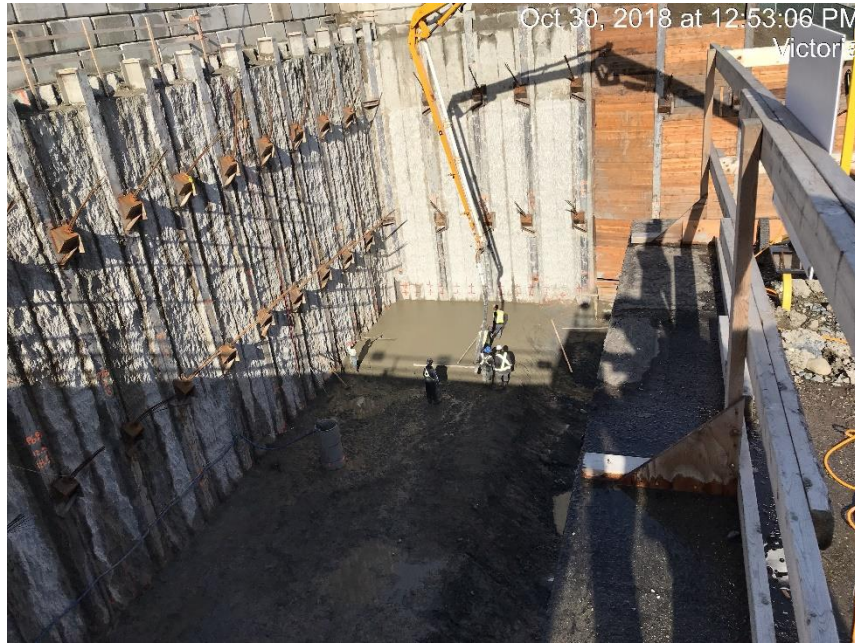
Figure 14 – Clover Point Pump Station: Placing mass concrete levelling pad 8.
