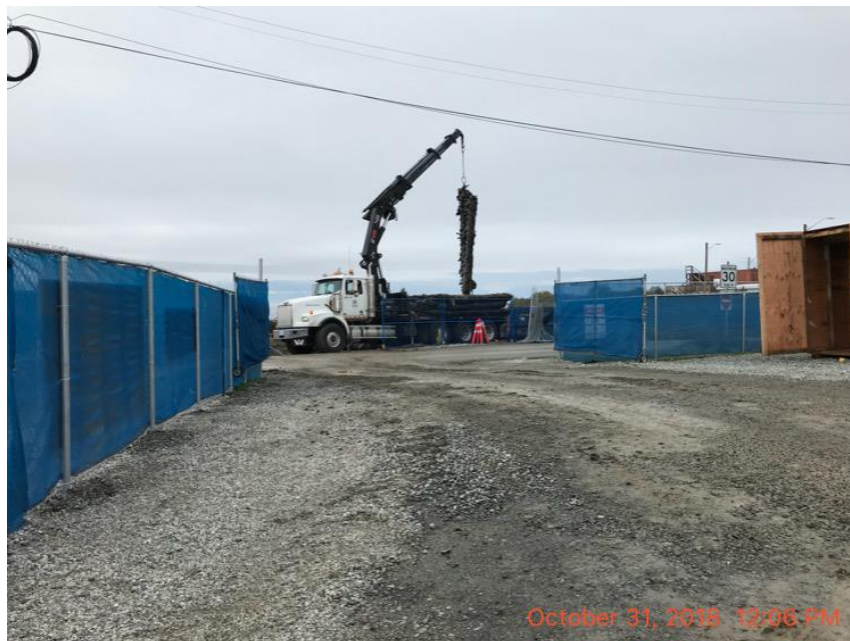
Figure 18 – Macaulay Point Pump Station: Additional blasting mats being delivered to site.
