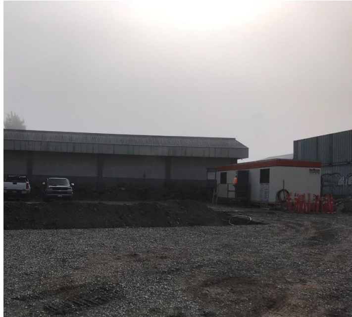
Figure 22 – Clover Forcemain: Mobilization of office trailer at Ogden Point.
