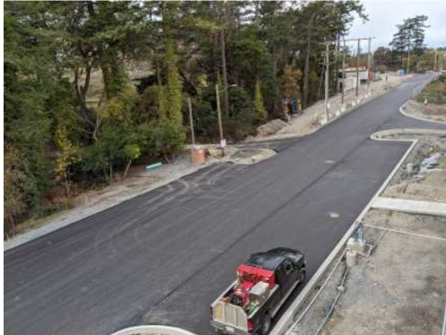
Figure 5– McLoughlin Point Wastewater Treatment Plant- Asphalt paving on Victoria View Road.
