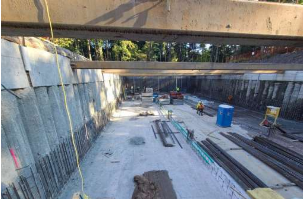
Figure 20—Arbutus Attenuation Tank- Main tank overview.
