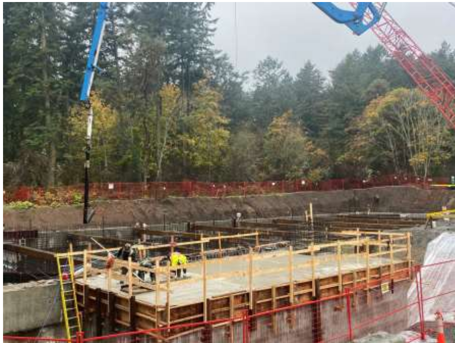
Figure 21—Arbutus Attenuation Tank- Valve chamber suspended slab pour.
