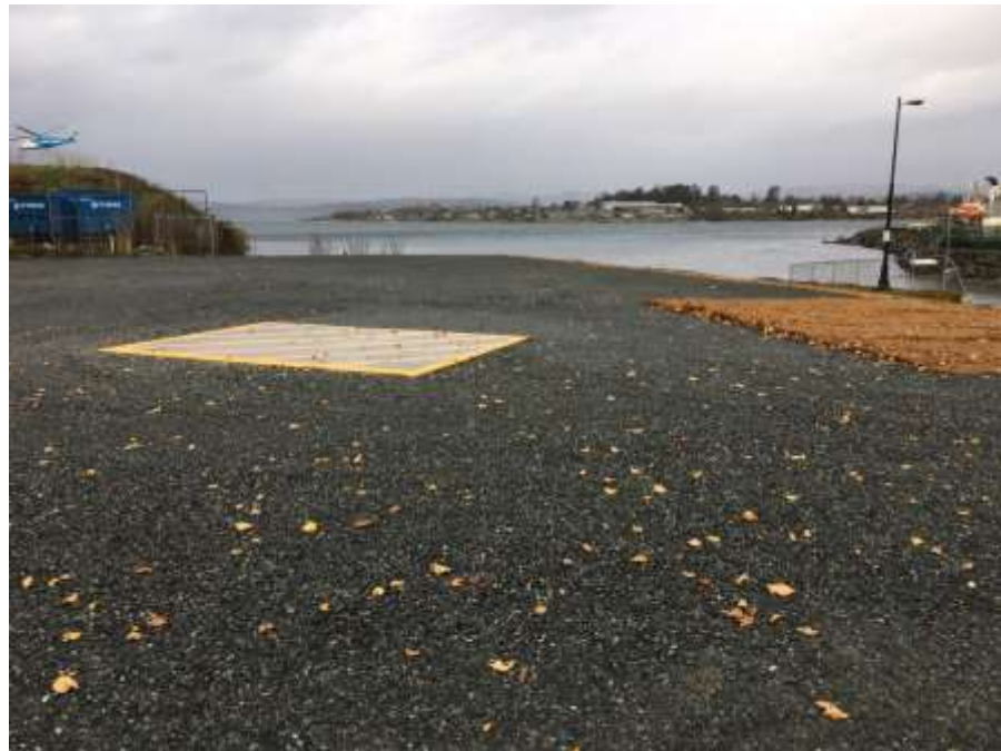
Figure 16–Clover Forcemain- Ogden Point restoration.
