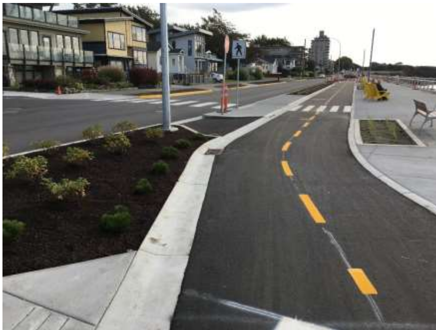
Figure 14–Clover Forcemain- Landscaping complete and lounge chairs installed.
