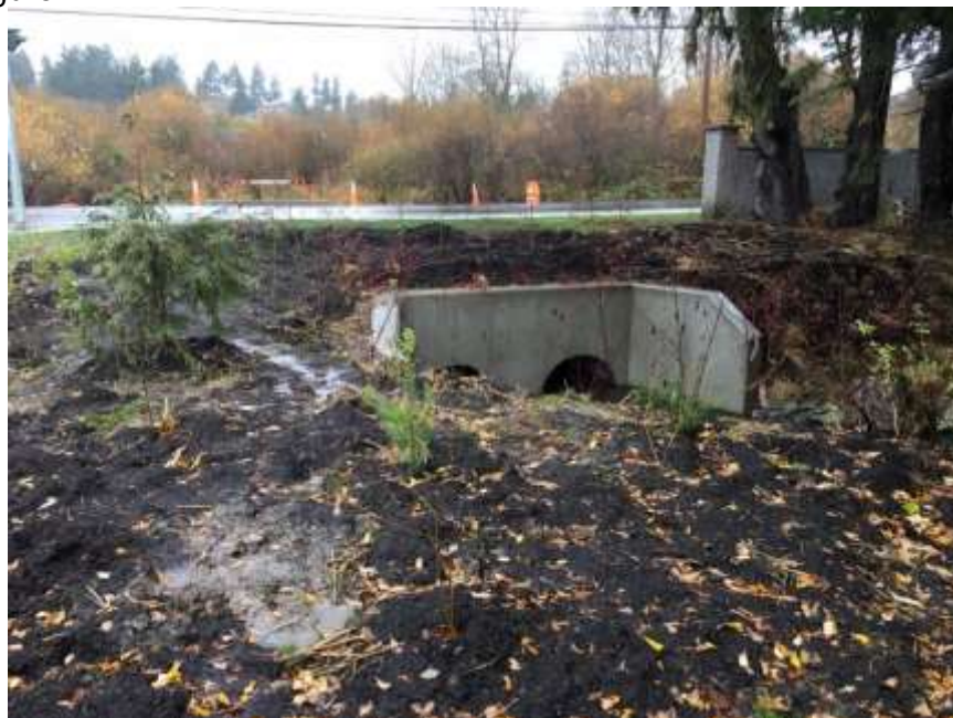
Figure 17–Residual Solids Pipes – Peers Creek – Vegetation restoration.
