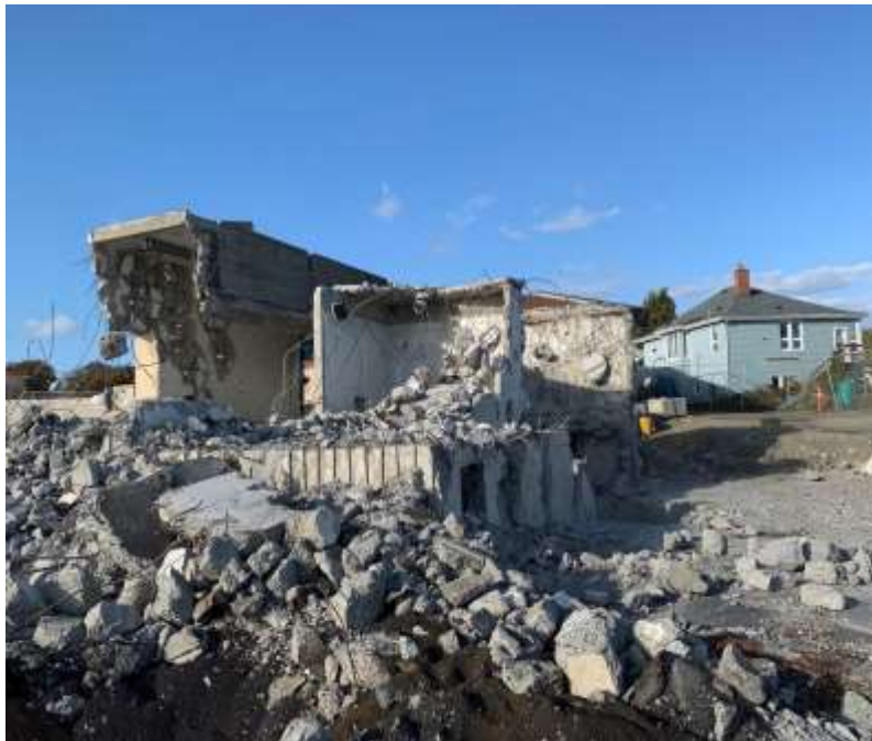
Figure 9–Macaulay Point Pump Station- Ongoing demolition of old pump station.
