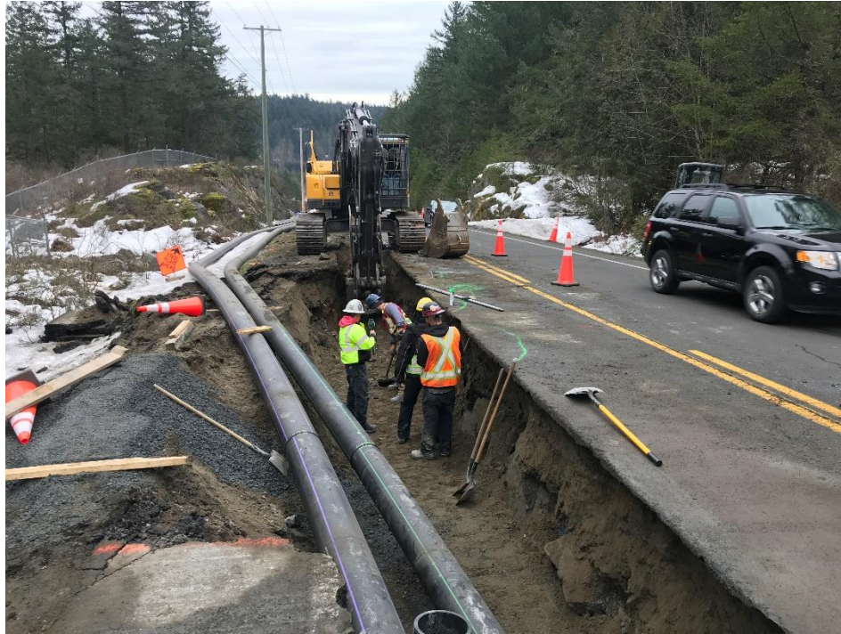
Figure 21 – Residual Solids Conveyance Line – Willis Point Road – Installing RSCL and CRL
