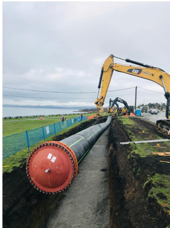
The 1.2m diameter Clover Forcemain is being lowered into the trench near Clover Point. There will be single lane alternating traffic on Dallas Road during construction.
