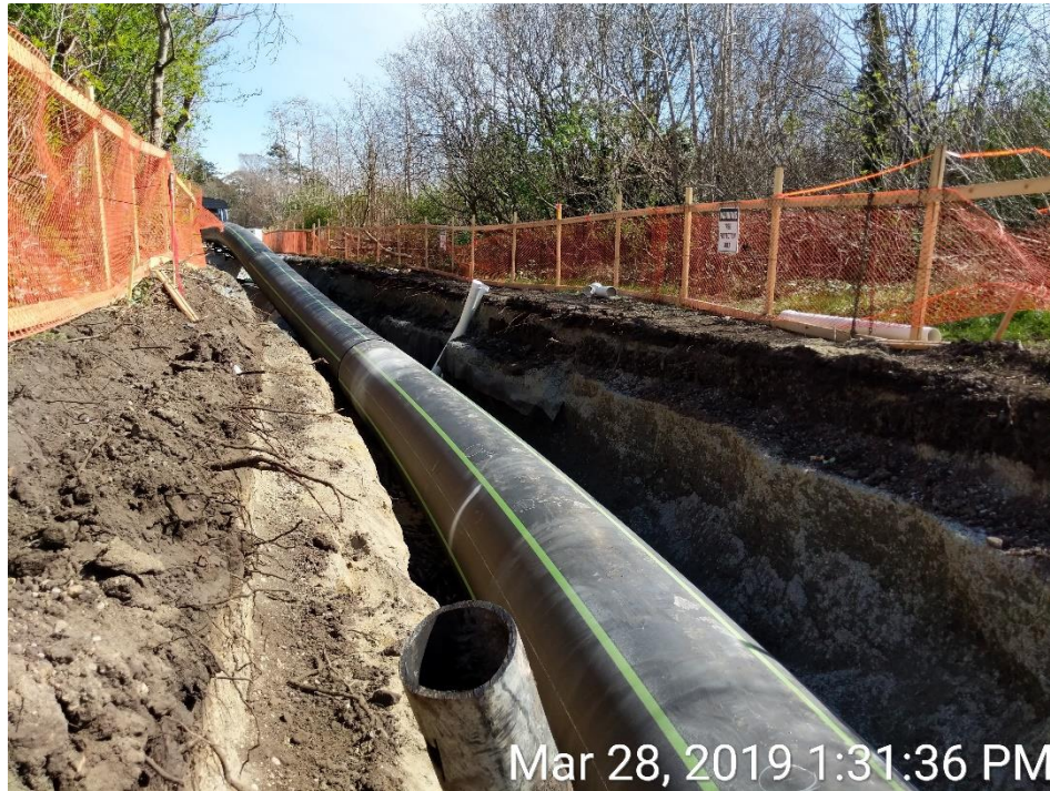
Figure 18 – Clover Forcemain: Dallas Road – installing forcemain through Camas Circle
