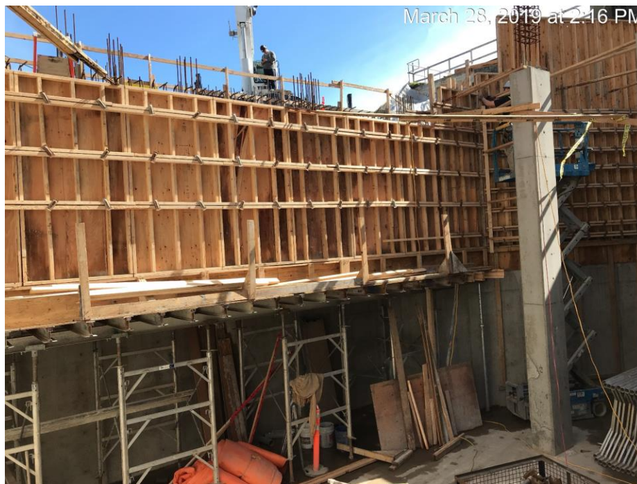
Figure 12 – Clover Point Pump Station: Wall 16 bracing being installed..
