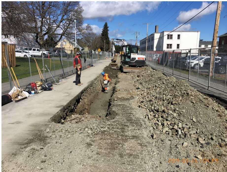
Figure 6 - McLoughlin Point Wastewater Treatment Plant: Installation of RSCL on Peter St.
