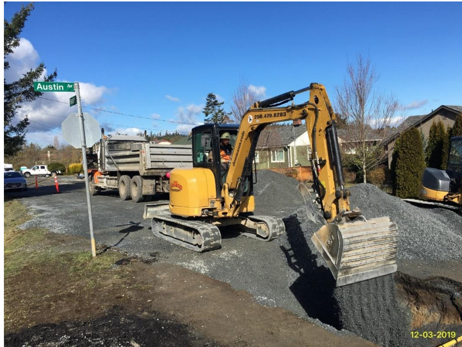
Figure 20– Residual Solids Conveyance Line: Newbury St – Back and compaction of RSCL
