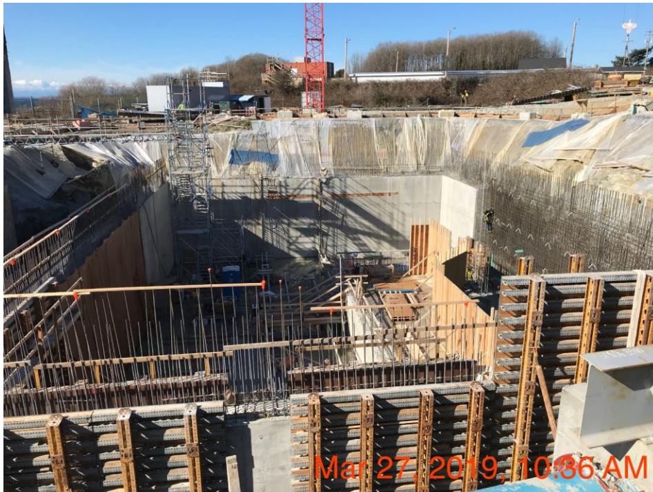
Figure 16 – Macaulay Point Pump Station: View looking west at overall site progress.
