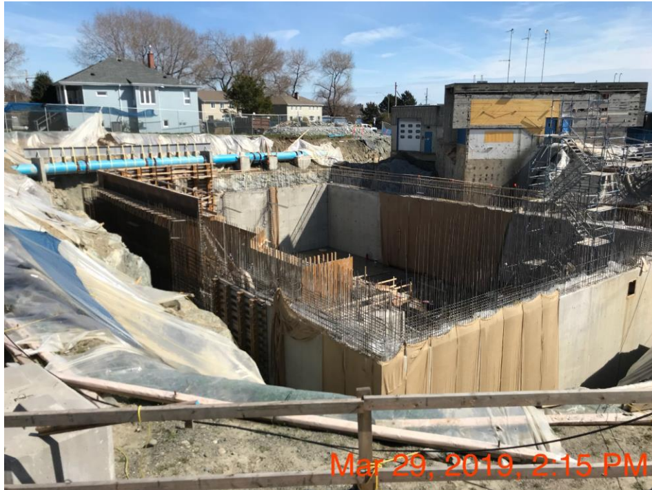
Figure 15 – Macaulay Point Pump Station: View looking SE at site progress.
