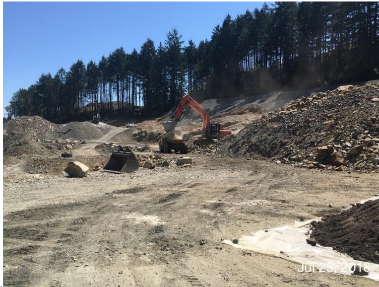
Figure 11 – Excavating and loading blast rock.
