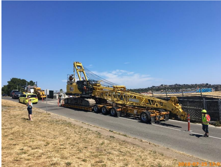
Figure 16 – Demobilizing crawler crane.
