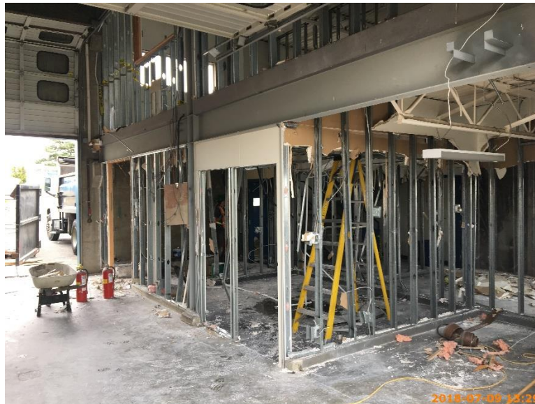
Figure 18 – demolition of interior walls.
