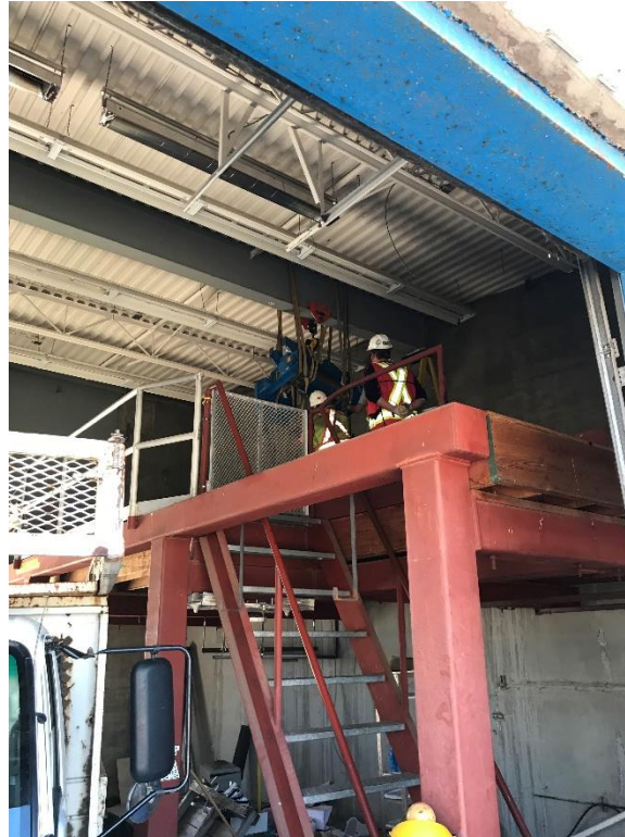
Figure 19 – Removal of gantry crane.
