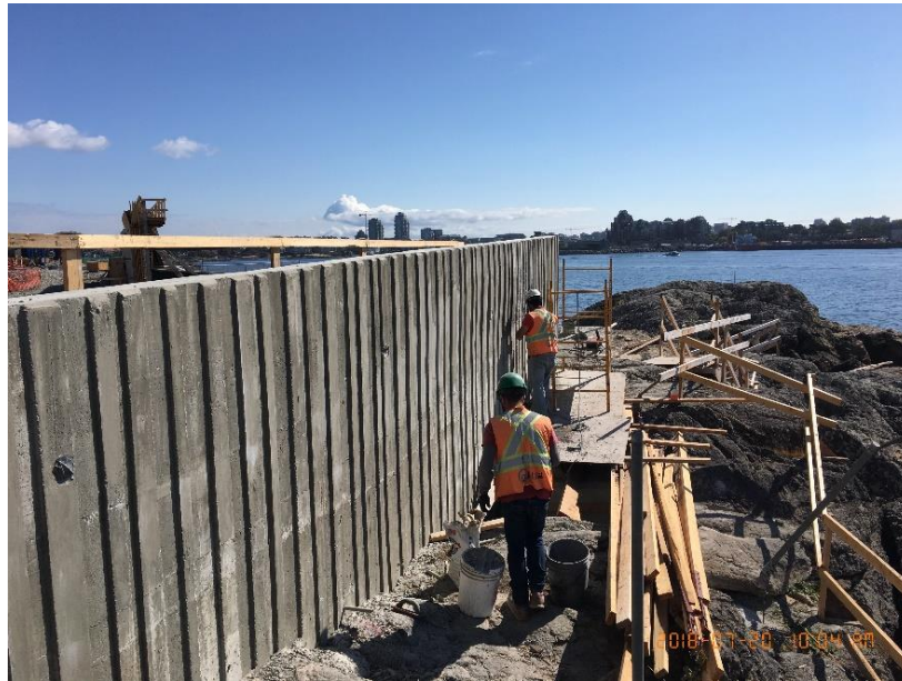
Figure 6 – Concrete finishing of planter wall #10.
