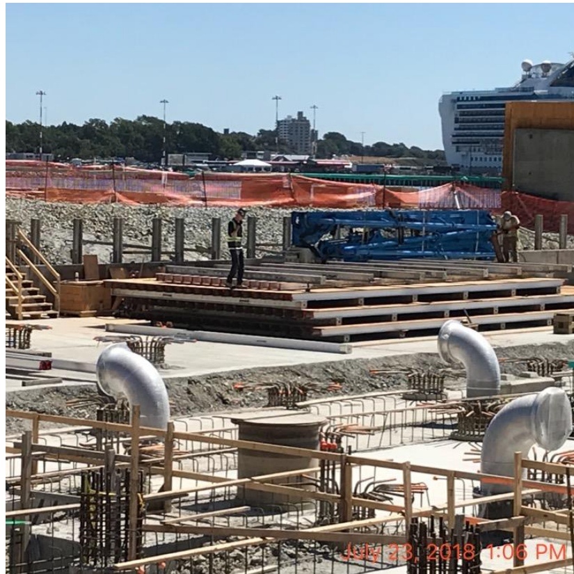
Figure 5 – Prefab wall gang forms for biological aerated filter (BAF) walls.
