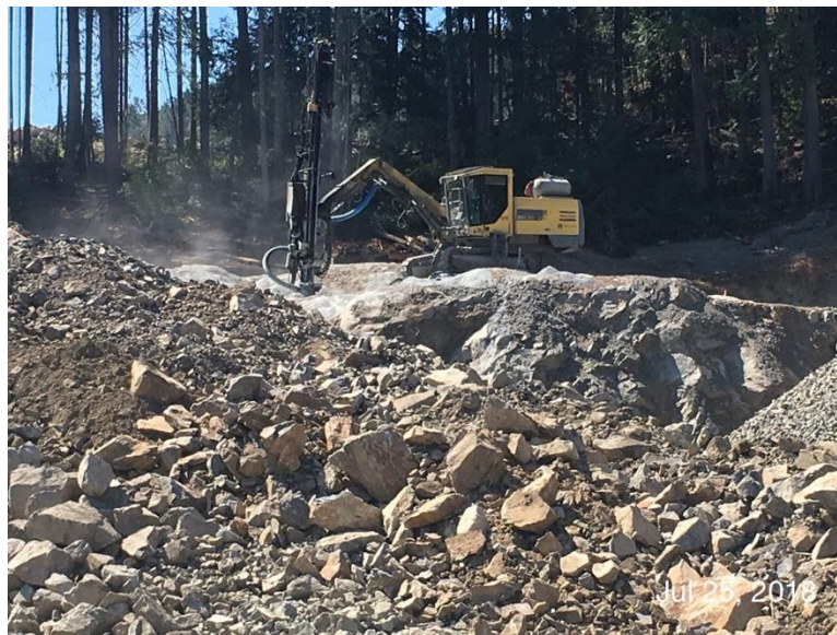
Figure 10 – Drilling holes for a blast
