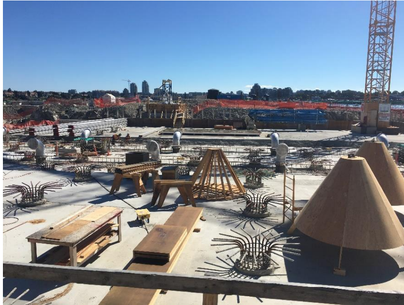
Figure 4 – Prefab Densadeg cones.
