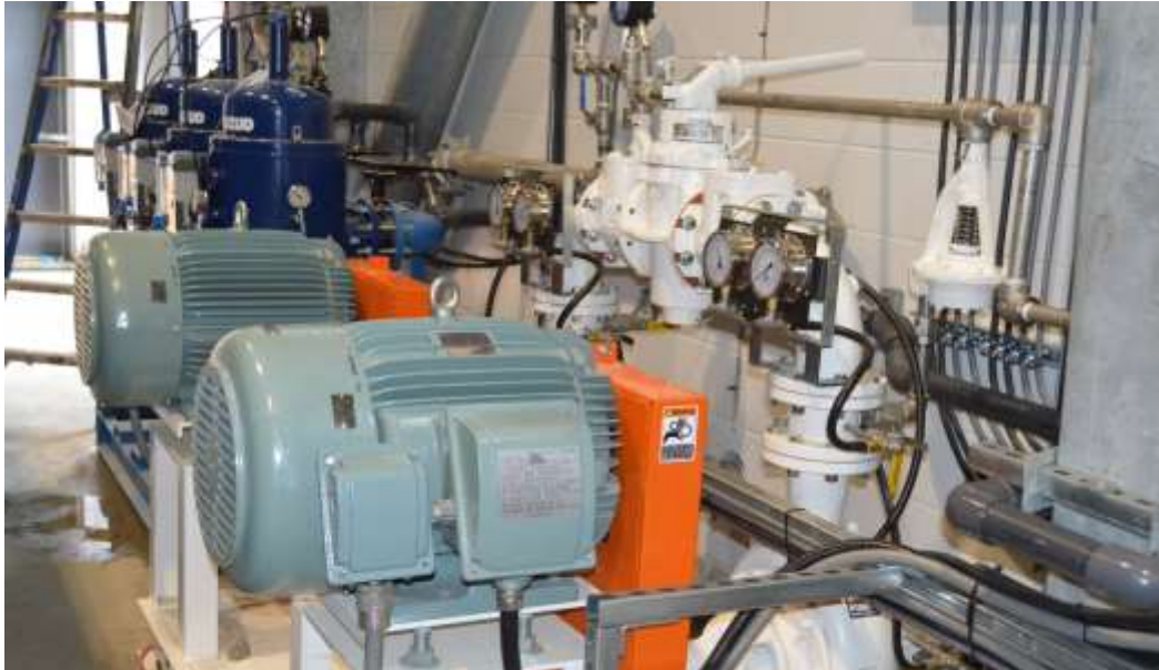
Figure 7- Residuals Treatment Facility- Filtrate self-priming pumps commissioning complete.
