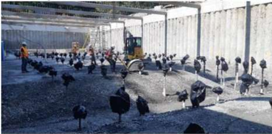
Figure 20–Arbutus Attenuation Tank- Installed Rock Anchors and Granular Material Compaction.
