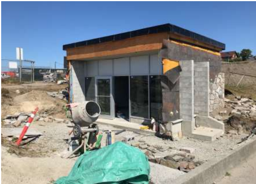
Figure 9–Clover Point Pump Station- Stone siding being installed on the public washroom.
