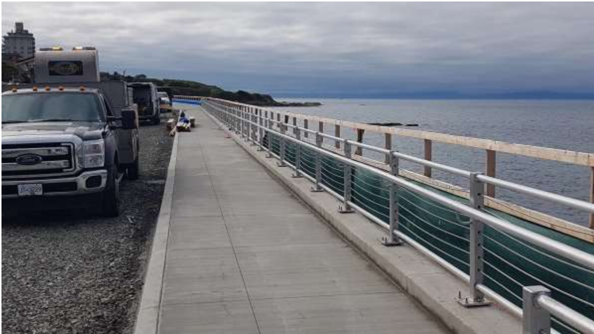
Figure 14–Clover Forcemain- New aluminium fence installed along Dallas Road.
