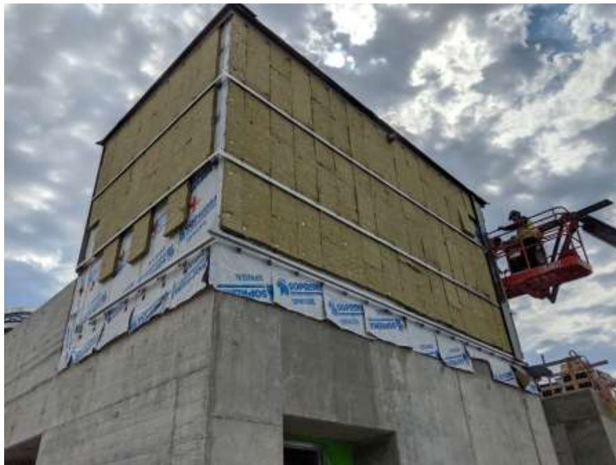
Figure 4- McLoughlin Point Wastewater Treatment Plant- Tertiary building stairway cladding installation.
