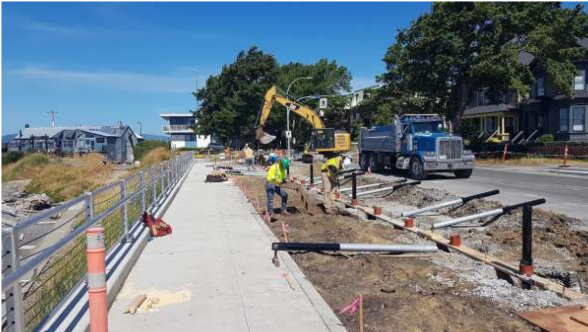
Figure 13–Clover Forcemain- Installing parking bollards along Dallas Road
