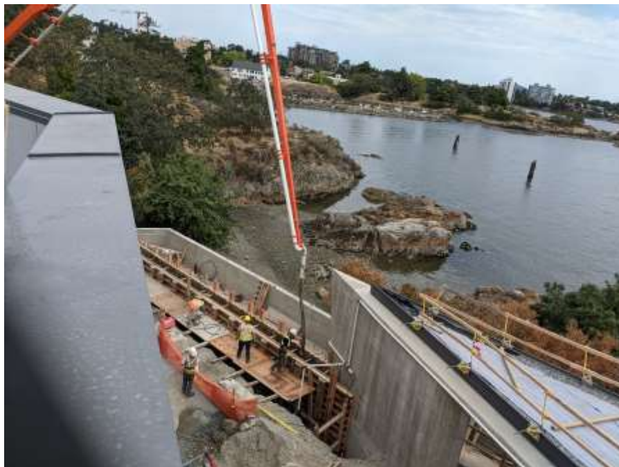
Figure 5- McLoughlin Point Wastewater Treatment Plant- North tsunami wall concrete pour.
