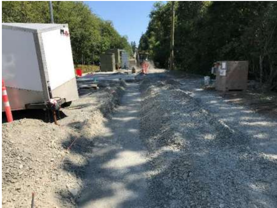
Figure 18 –Residual Solids Pump Stations – Pump Station # 1: Excavating to install curbs.
