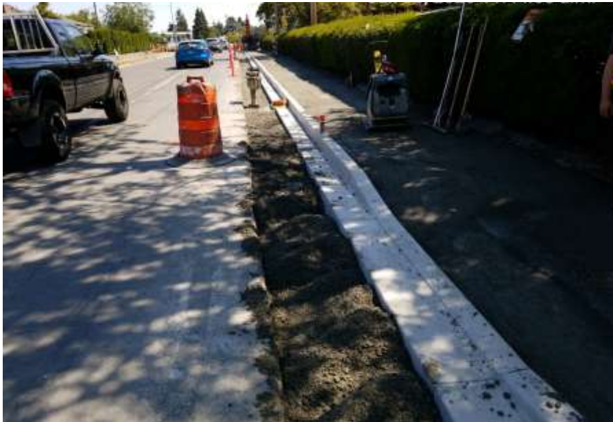
Figure 21–Trent Forcemain- Fairfield Road curb and sidewalk subgrade preparation.
