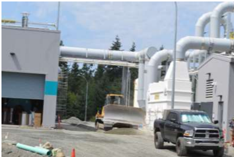
Figure 6– Residuals Treatment Facility- Ongoing placement and compaction of road base.
