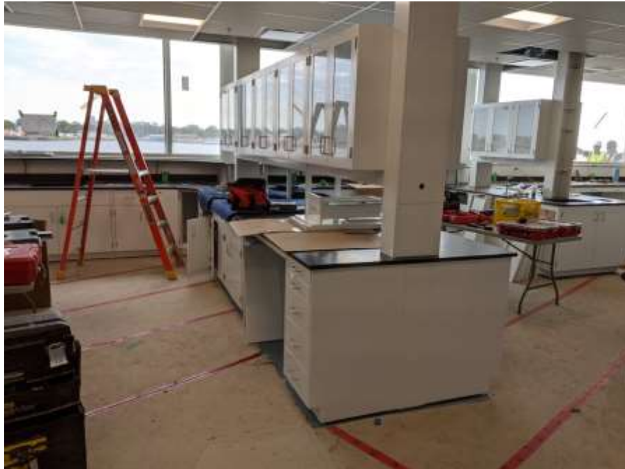
Figure 2– McLoughlin Point Wastewater Treatment Plant – Installation of cabinets in the Laboratory.
