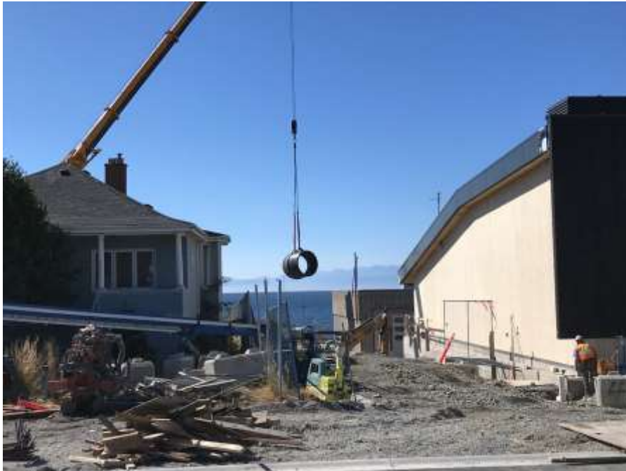
Figure 11–Macaulay Point Pump Station- Final section of pipe being installed.
