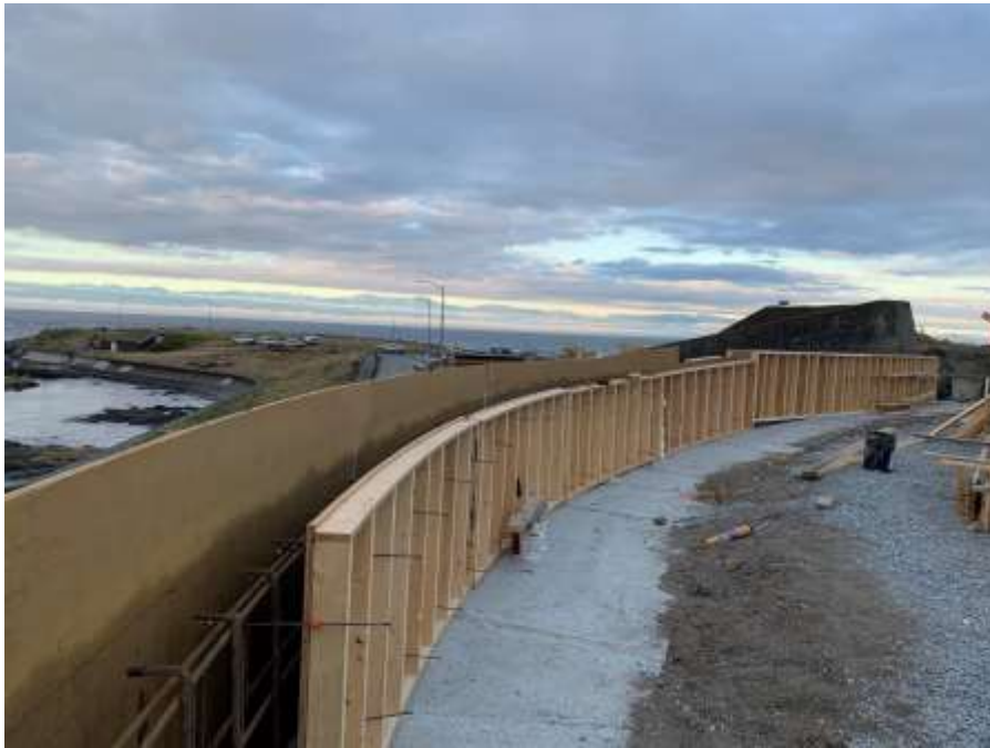
Figure 10- Clover Point Pump Station – Curved landscape retaining wall formwork.
