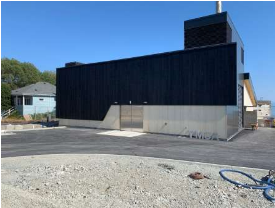
Figure 12–Macaulay Point Pump Station- Exterior finishes.
