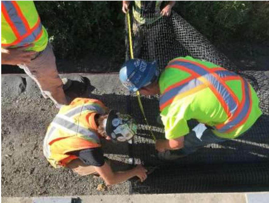
Figure 16-Residual Solids Pipes - Building layers of geobag wall at Admirals Bridge.
