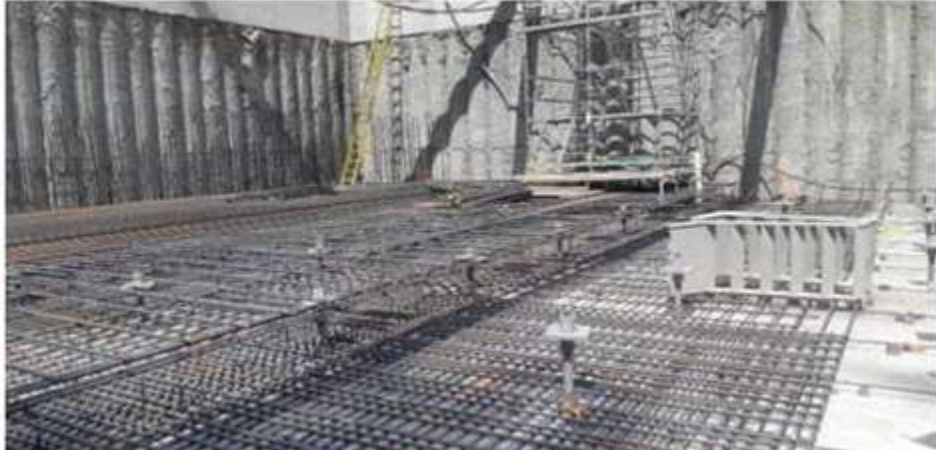
Figure 19–Arbutus Attenuation Tank- Base Slab Steel Installation Progress.
