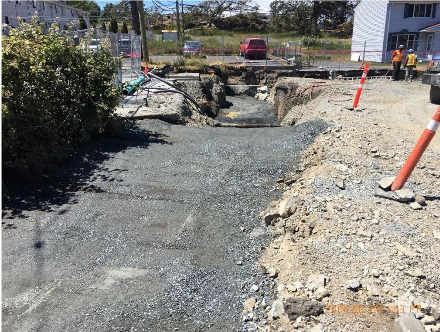
Figure 3 - Mcloughlin Point Wastewater Treatment Plant – Back filling BC Hydro duct bank Patricia Way
