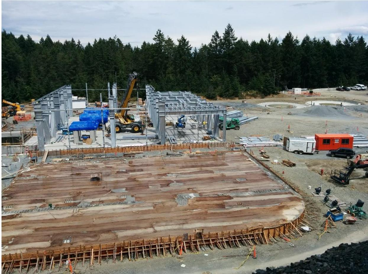
*Figure 8– Residuals Treatment Facility – Dry building foundation wet curing and steel erection of Residuals Handling Building.*
