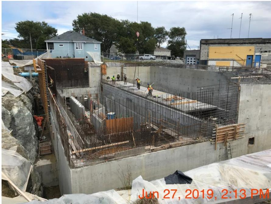
*Figure 15—Macaulay Point pump station & forcemain – placing precast concrete slabs over the wet well.*
