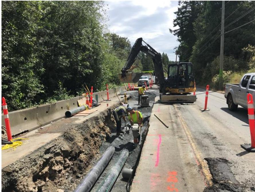
*Figure 20 – Residual Solids Conveyance Line: Bedding and backfilling pipe at Interurban Road.*
