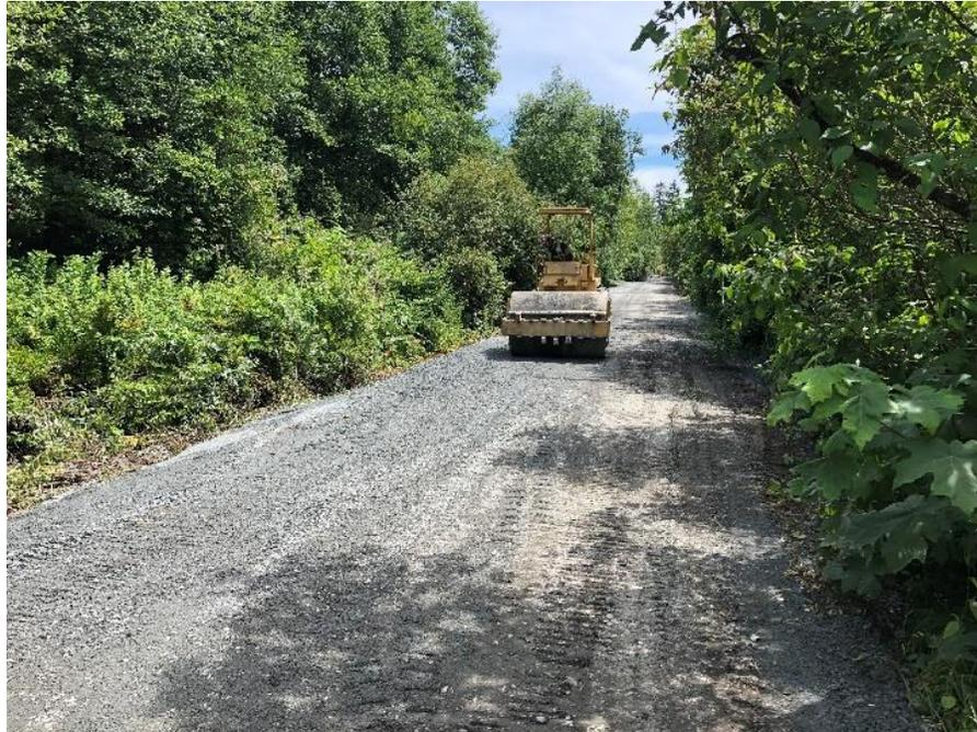
*Figure 19 – Residual Solids Conveyance Line: Compaction of surface lift of backfill gravel.*
