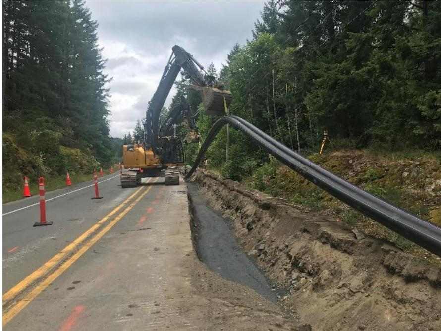
Figure 22 – Residual Solids Conveyance Line: lifting fused Residual Solids Forcemain and Residual Solids Return Line pipes into trench at Willis Point Road
