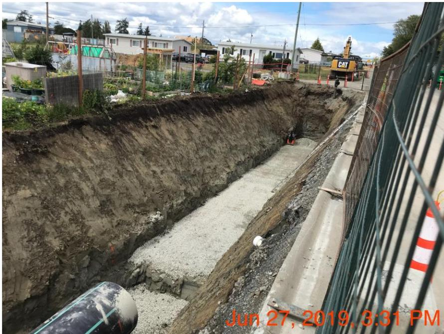
Figure 14–Macaulay Point pump station & forcemain – Forcemain bedding compaction in progress.
