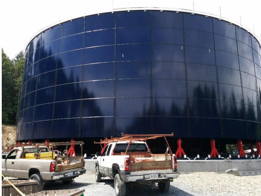
*Figure 6– Residuals Treatment Facility – Digester 1 final lift in progress.*
