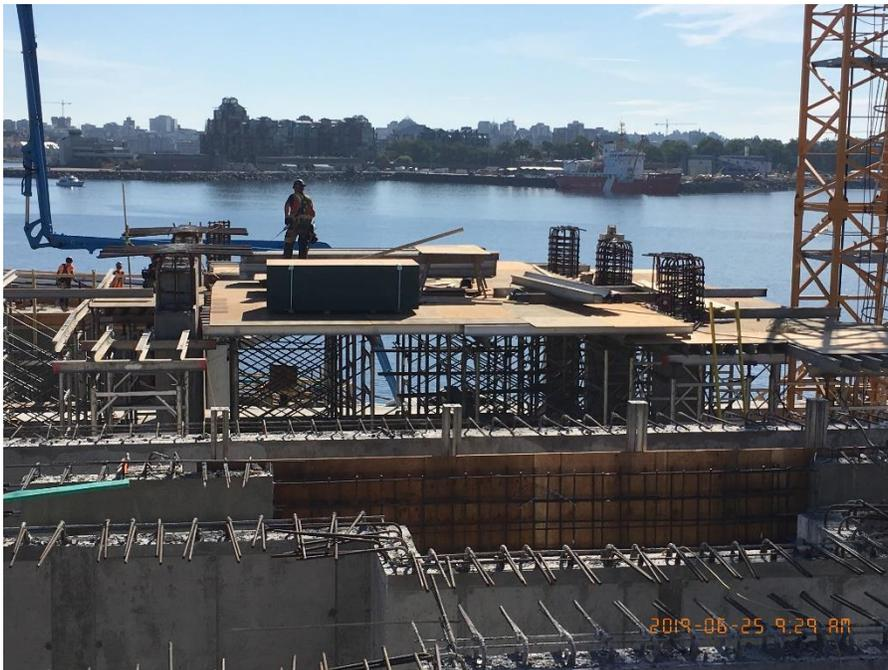
Figure 4 – Mcloughlin Point Wastewater Treatment Plant – decking of Biological Aerated Filter heat recovery room suspended slab.
