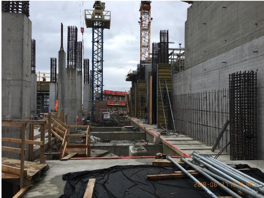
*Figure 2 – McLoughlin Point Wastewater Treatment Plant – Forming columns in Operations & Maintenance breeze way.*
