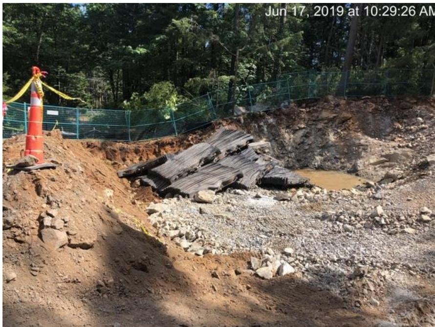
Figure 23 – Residual Solids Conveyance Line: Blast mats in place prior to blast #1 at pump station #3
