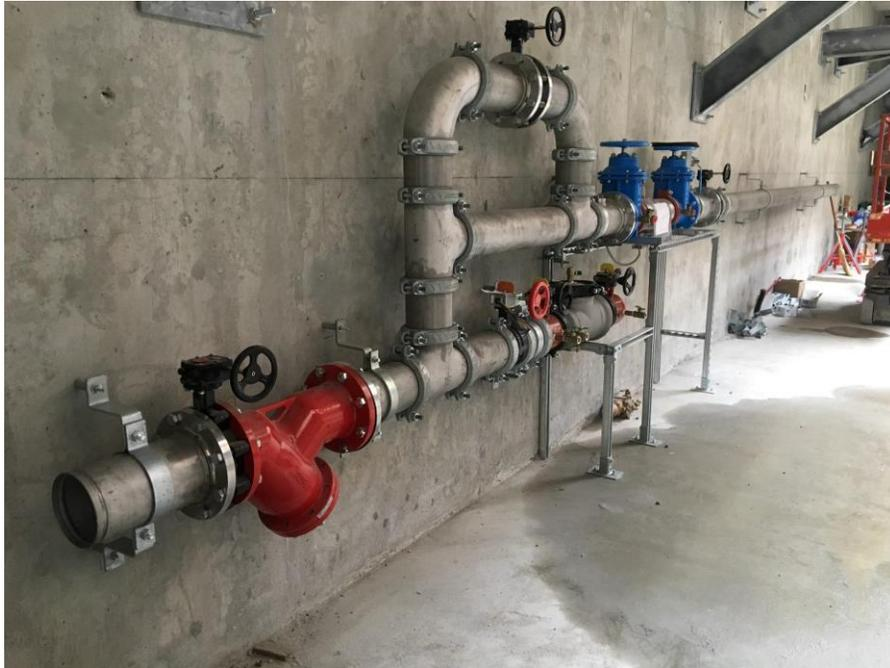
*Figure 9–Clover Point Pump Station – installation of water entry piping in the pump room*
