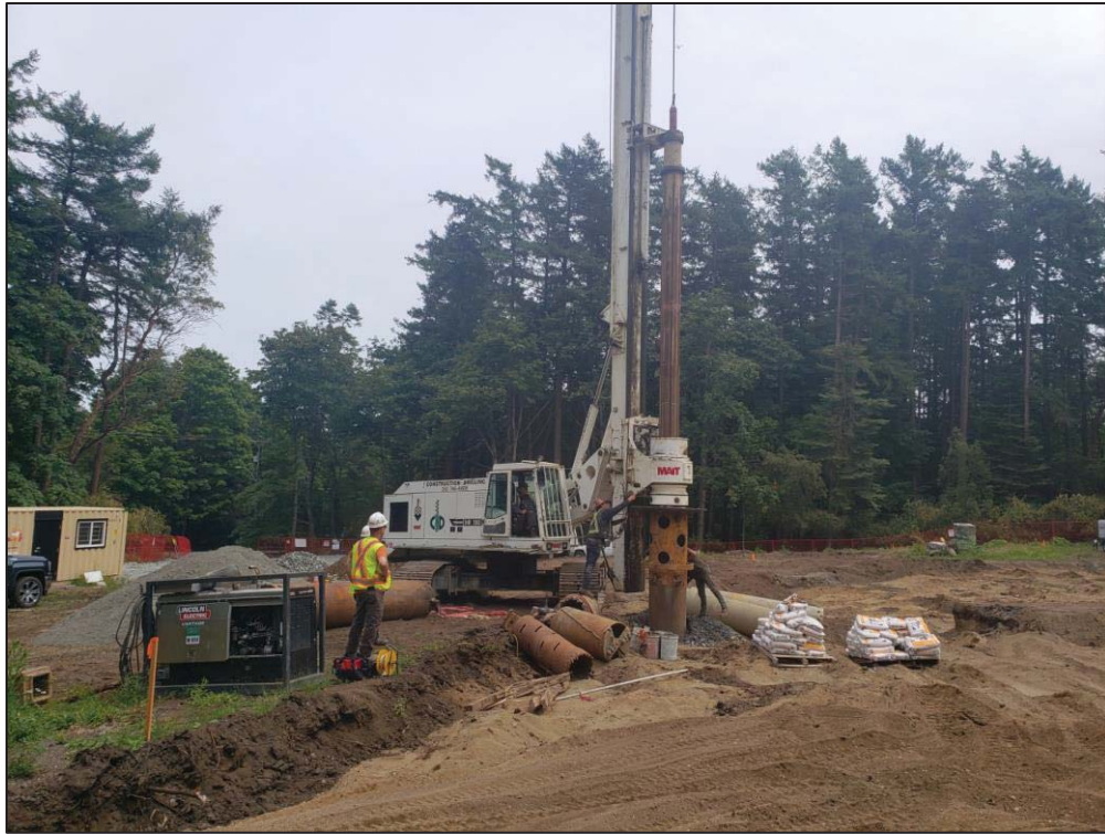
Figure 30– Arbutus Attenuation Tank - Drilling dewatering test wells
