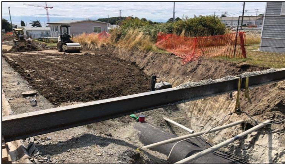
Figure 15–Macaulay Point Pump Station- Backfilling and compacting forcemain trench with native material.
