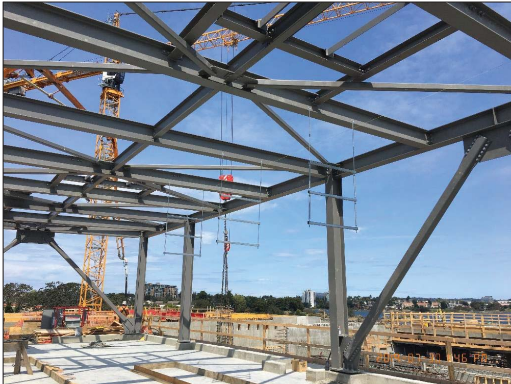
Figure 3– McLoughlin Point Wastewater Treatment Plant- Cable tray hangers in electrical room.
