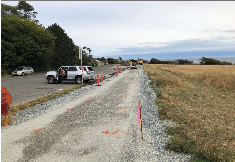
Figure 21–Clover Forcemain-Cycle Track Base Preparation (Clover Point).
