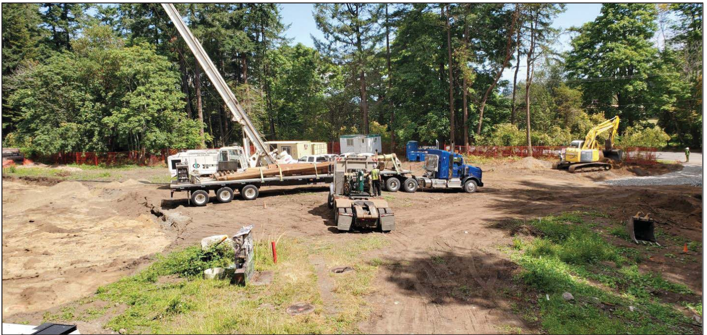
Figure 31– Arbutus Attenuation Tank- Mobilizing drill rig to site
