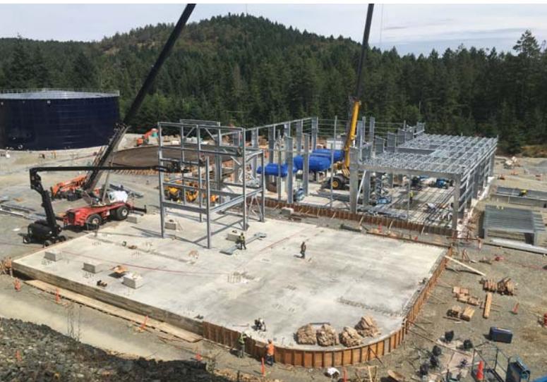
Progress at the Residuals Treatment Facility
