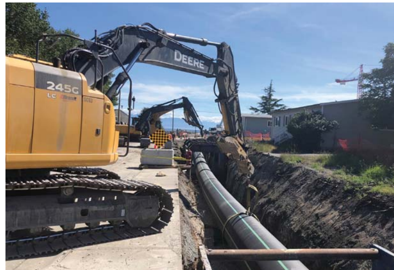
Installation of the Macaulay Forcemain on Anson Street
