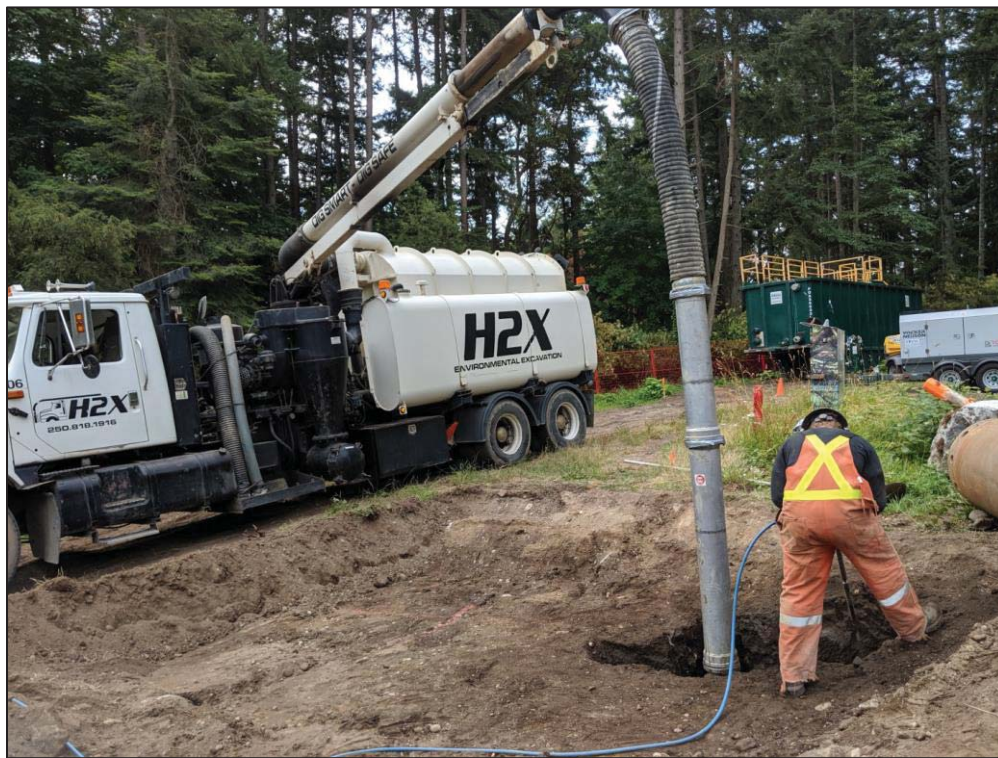
Figure 29–Arbutus Attenuation Tank- Daylighting existing utilities
