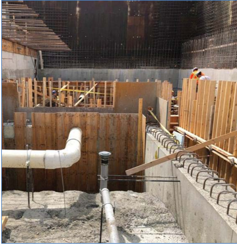
Figure 16–Macaulay Point Pump Station- Installing vertical form work around vortex degritter.
