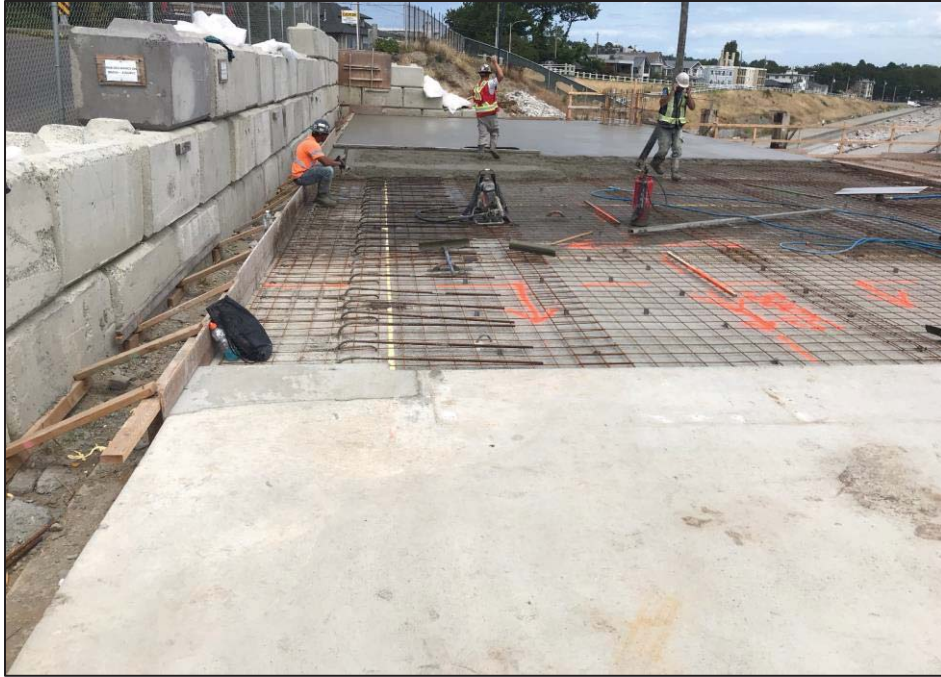
Figure 11–Clover Point Pump Station- Roof slab concrete pour.
