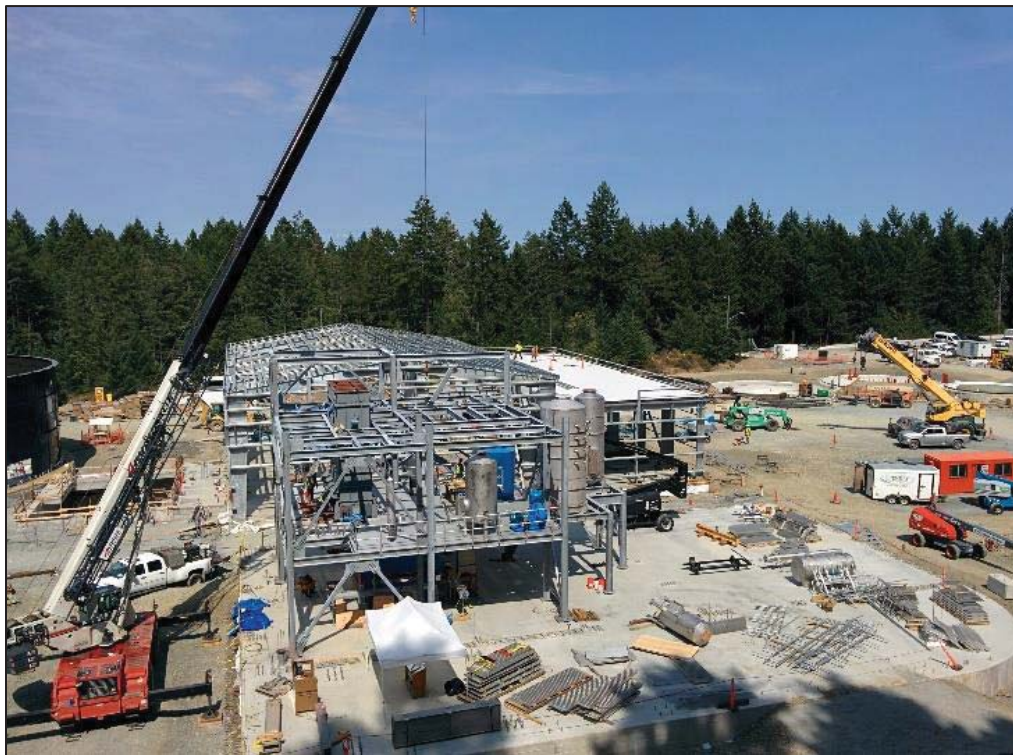
Figure 7- Residuals Treatment Facility- Residual drying facility mechanical equipment installation.
