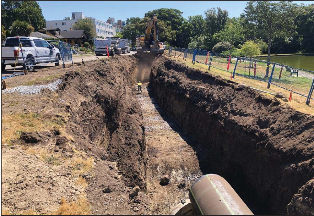
Figure 19–Clover Forcemain- Trenching advanced through Holland Point Park (Yacht Pond)
