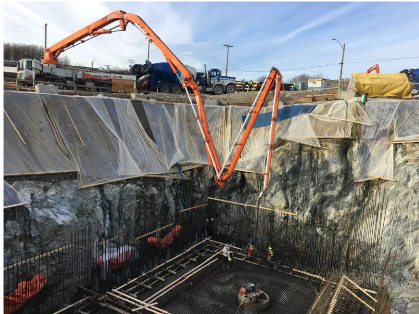
Figure 20 – Macaulay Point Pump Station: commencement of base slab pour.
