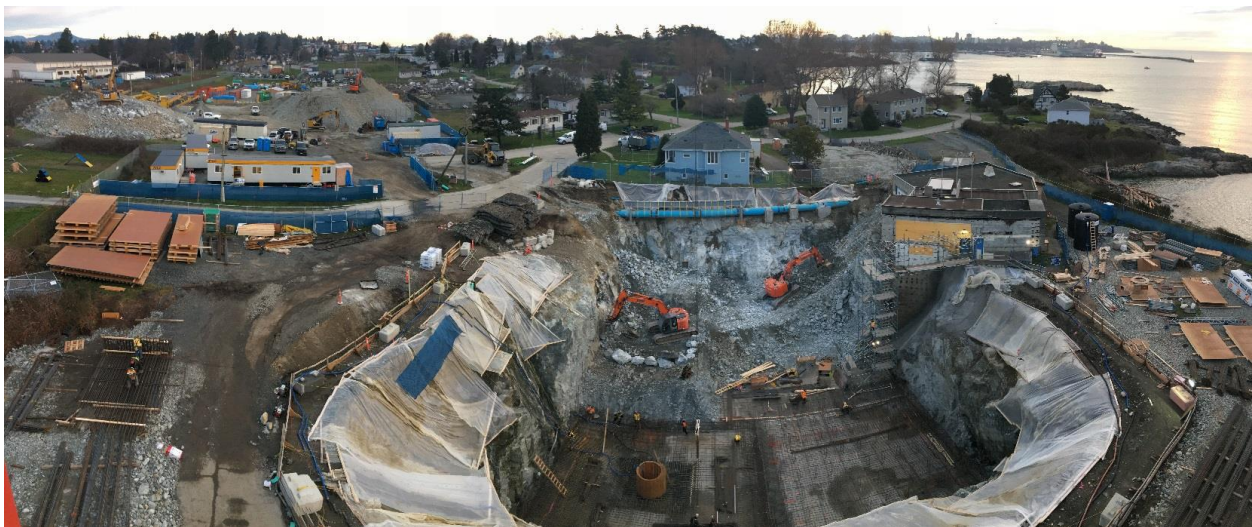
Figure 18 – Macaulay Point Pump Station: view from the tower crane looking east.
