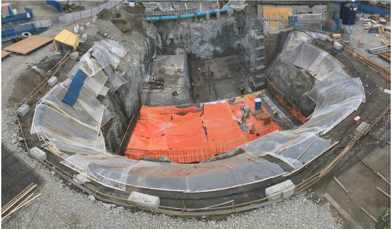
Figure 19 – Macaulay Point Pump Station: progression of south east quadrant base slab.
