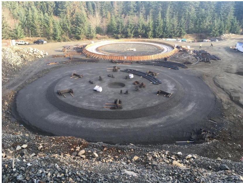
Figure 9 – Residuals Treatment Facility: digester #1 and #2 perimeter slab and base gravels.
