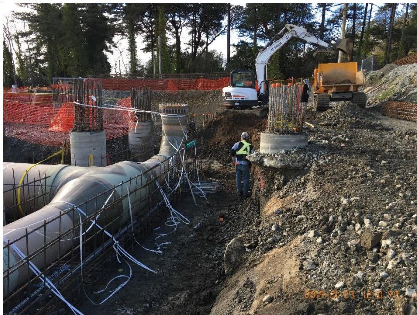
Figure 8 – McLoughlin Point Wastewater Treatment Plant: excavating for Densadeg sludge lines.
