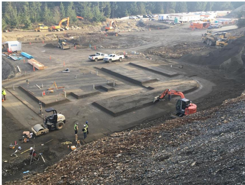
Figure 10 – Residuals Treatment Facility: dryer building base gravels, ready for formwork.
