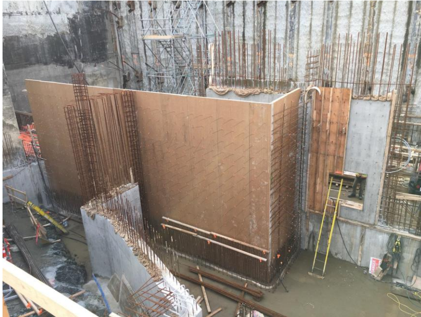
Figure 16 – Clover Point Pump Station: formwork ongoing – sanitary wet well wall.
