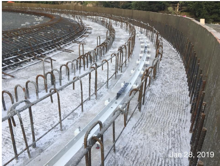
Figure 12 – Residuals Treatment Facility: installing levelling ring in digester #1.
