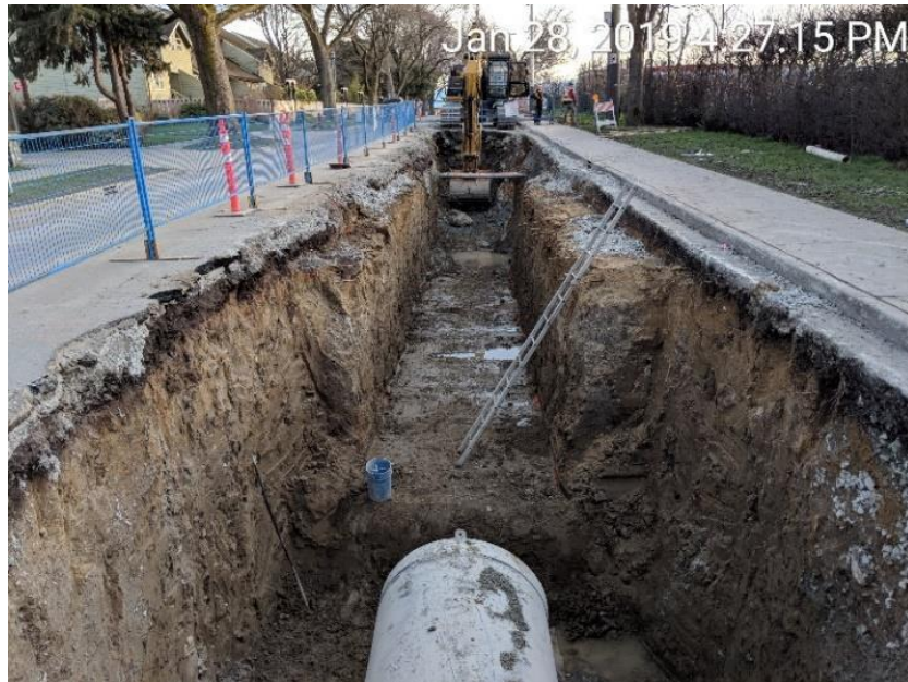
Figure 22 – Clover Forcemain: forcemain trench excavation in progress.
