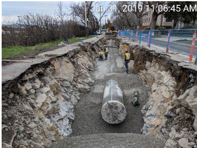
Figure 21 – Clover Forcemain: backfilling and compacting forcemain at Ogden Point end.
