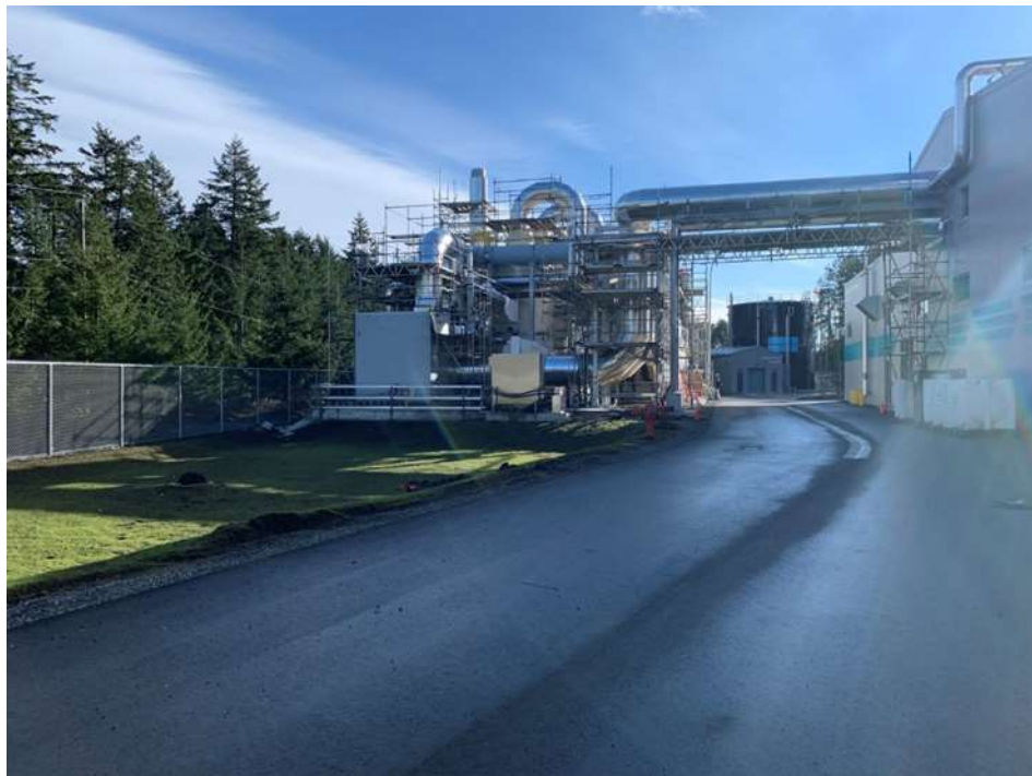
Figure 2– Residuals Treatment Facility- Odour Control and Storm Pond.
