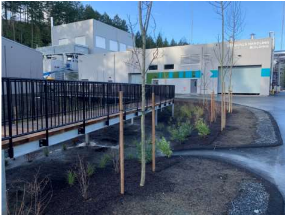
Figure 3- Residuals Treatment Facility- Boardwalk and Landscaping.
