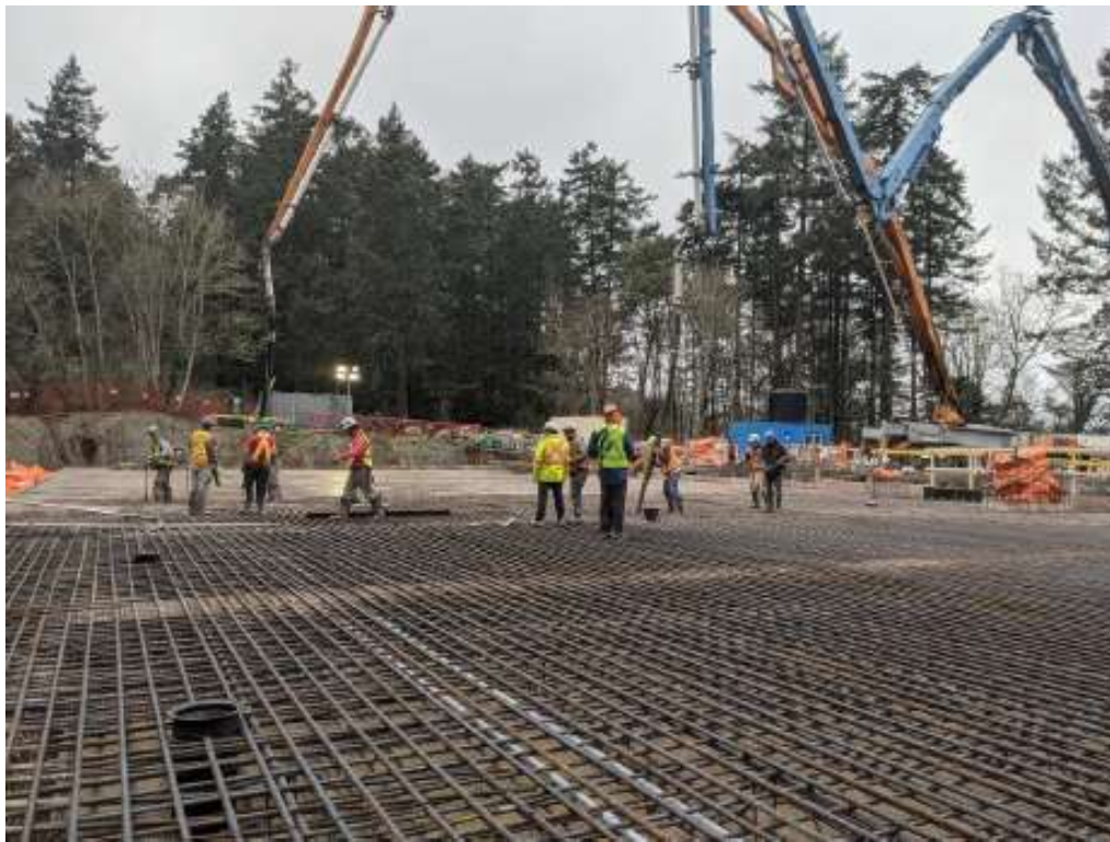
Figure 10–Arbutus Attenuation Tank- Concrete pours are ongoing.
