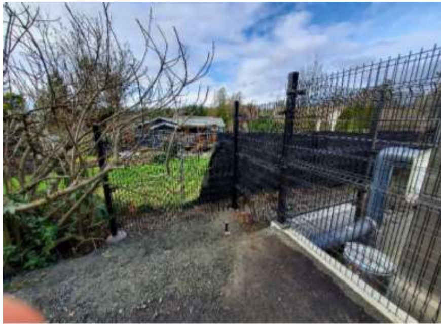
Figure 8–Residual Solids Pump Stations– completed fence installation at Pump Station 1
