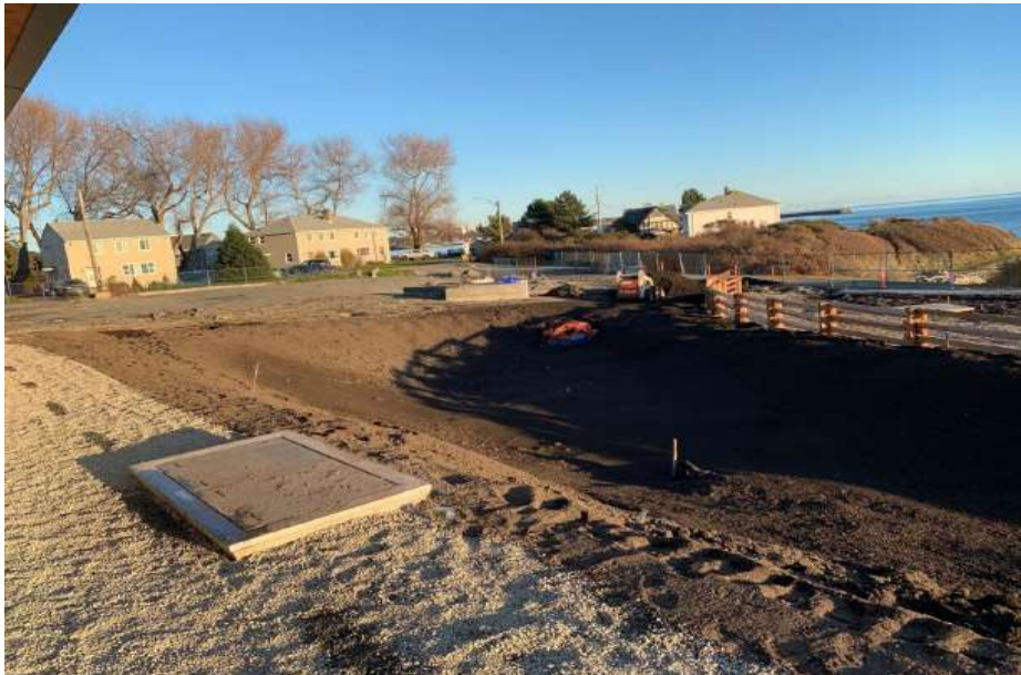
Figure 6–Macaulay Point Pump Station: Rain garden excavation
