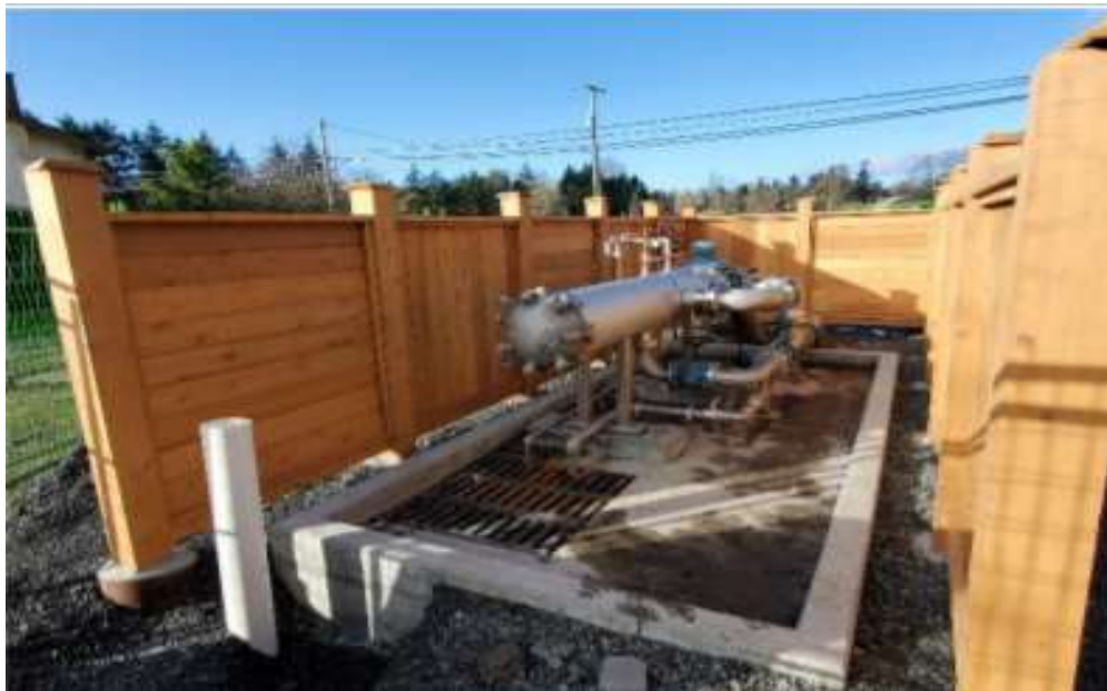
Figure 9 –Residual Solids Pump Stations – Fencing installed at the Marigold Valve Chamber
