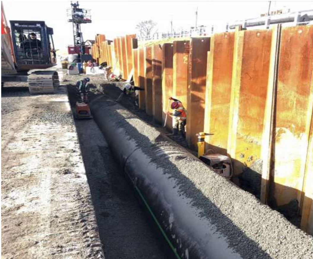
Figure 12-Trent Forcemain- Backfilling at the Seawall
