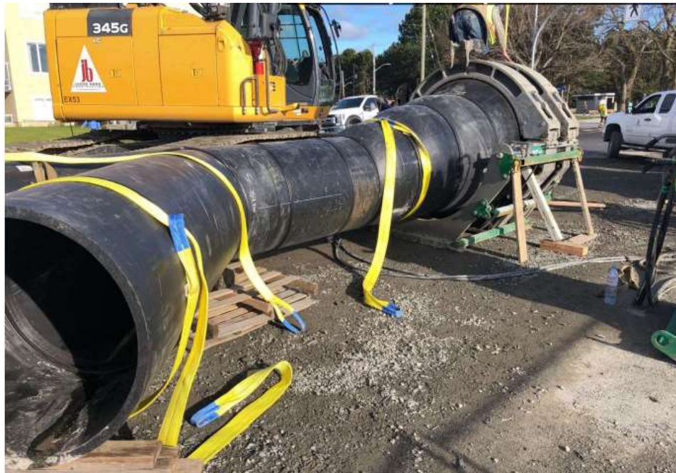
Figure 13-Trent Forcemain- Seawall field fusion of wye-reducer-bend section.
