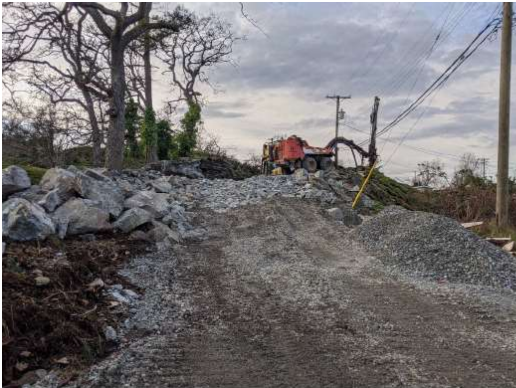
Figure 7-BC Hydro Access Road excavation
