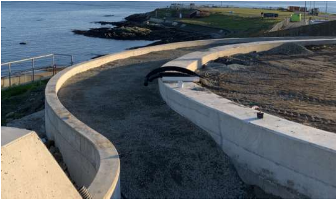
Figure 4—Clover Point Pump Station- Continuing landscaping.
