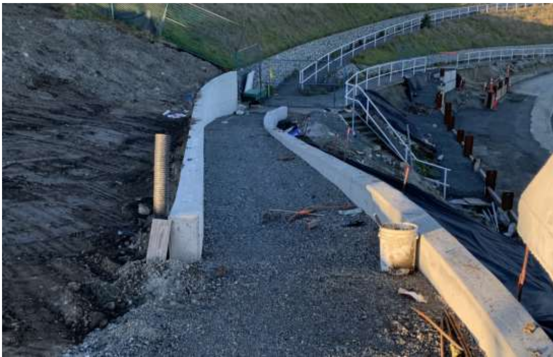
Figure 5—Clover Point Pump Station- Continuing landscaping.
