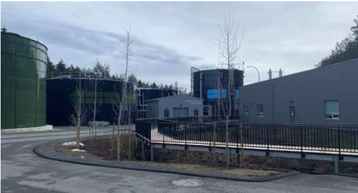
Figure 3– Residuals Treatment Facility- Operations Building Boardwalk.
