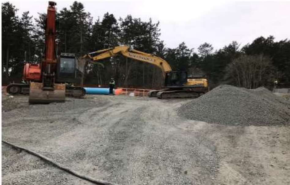
Figure 8–Arbutus Attenuation Tank- Site view facing north.
