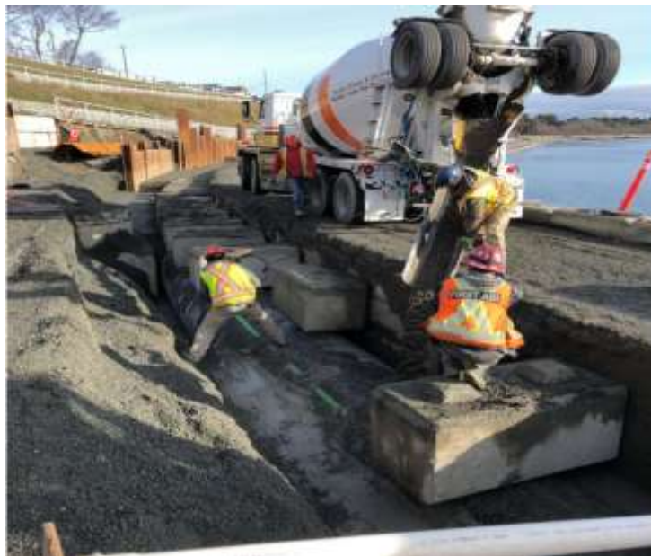
Figure 11–Trent Forcemain- Controlled density fill installation around high density polyethylene pipe.
