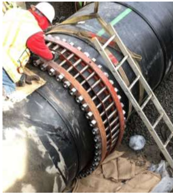
Figure 10–Trent Forcemain- Seawall Flange Bolt up
