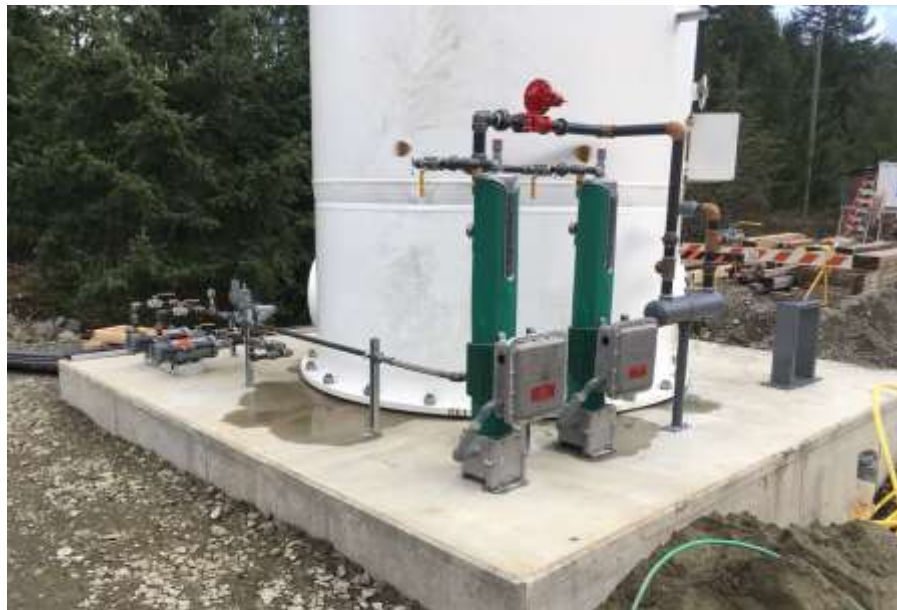
Figure 9– Residuals Treatment Facility- Installation of mechanical equipment at propane storage tank.
