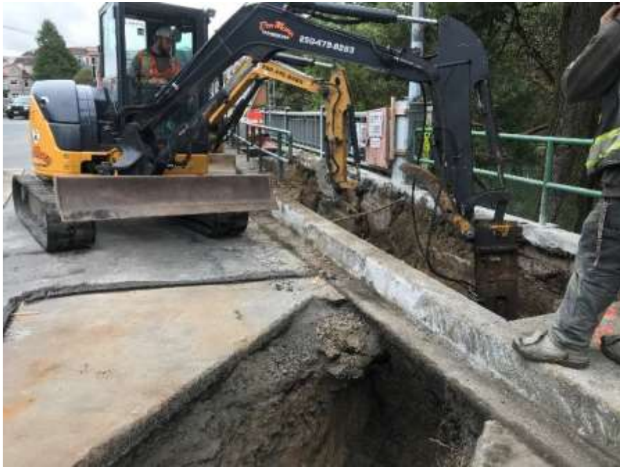
Figure 23–Residual Solids Pipes - Excavation of sidewalk for pipe installation.
