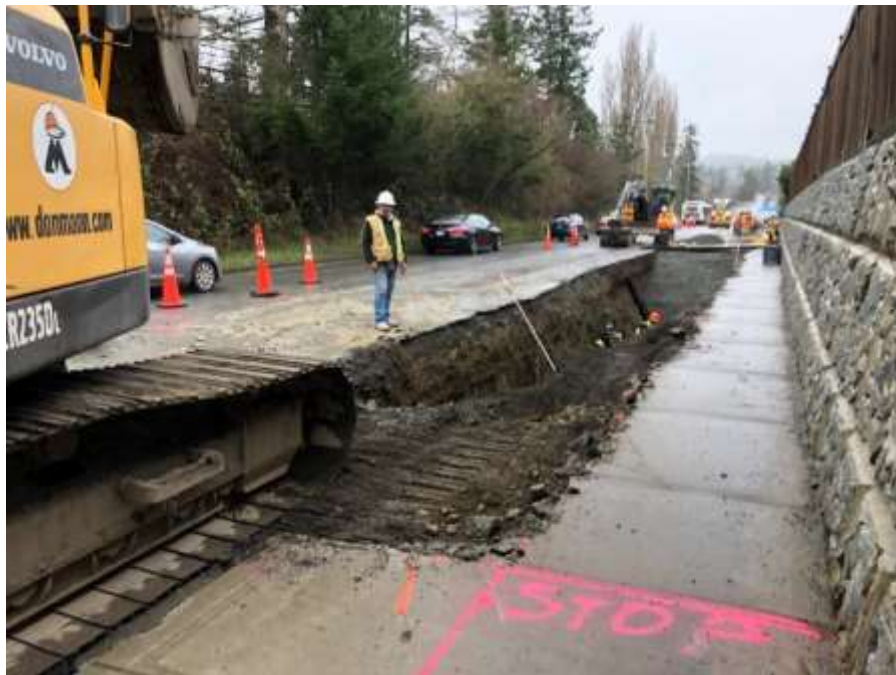
Figure 21–Residual Solids Pipes- installation of pipe on Interurban Road.
