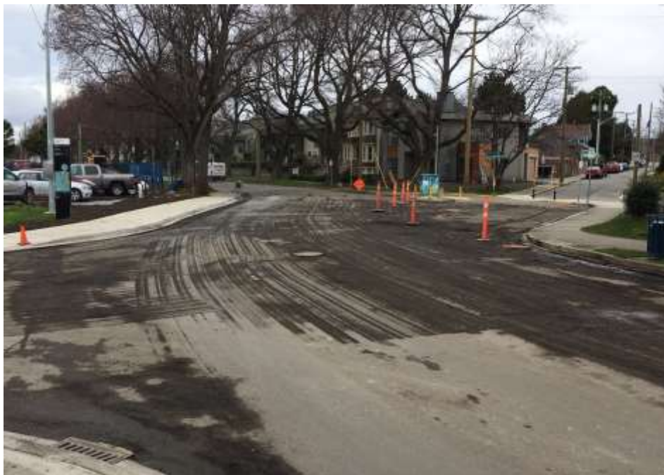
Figure 18–Clover Forcemain– Road restoration between Niagara and Dock streets.
