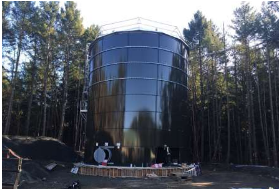
Figure 24–Residual Solids Pump Stations– Hartland Water System Improvements – Reservoir installation progress.
