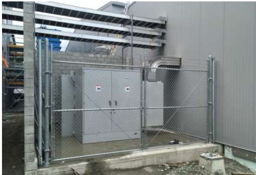
Figure 8– Residuals Treatment Facility- chain link fence enclosure installed around main transformer.
