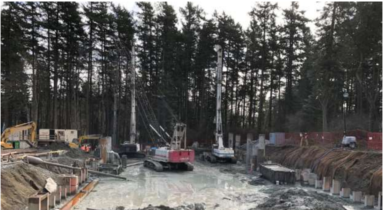
Figure 26–Arbutus Attenuation Tank- Secant Pile Installation – 2 drill rigs & 1 crane.
