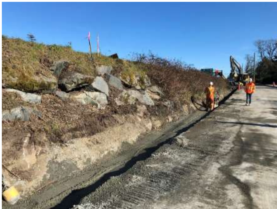
Figure 22–Residual Solids Pipes – Pipe installation on Portage Road.
