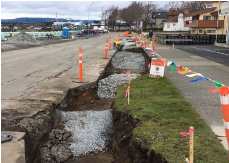
Figure 17–Clover Forcemain- Curb and gutter restoration between Dock and Oswego streets.
