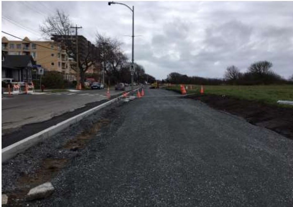
Figure 16–Clover Forcemain- Cycle track base prep between Lewis and Douglas Streets.
