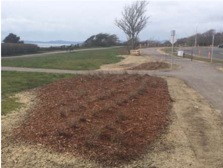
Figure 19–Clover Forcemain- Landscaping near corner of Cook Street and Dallas Road.
