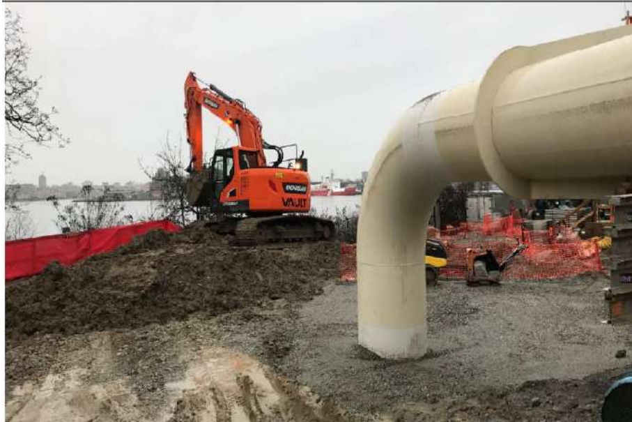
Figure 2– McLoughlin Point Wastewater Treatment Plant- Backfilling harbour crossing pipe.
