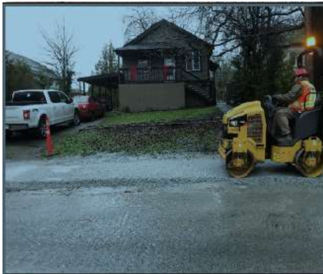
Figure 22—Residual Solids Pipes- Compacting gravel on Vincent Ave.
