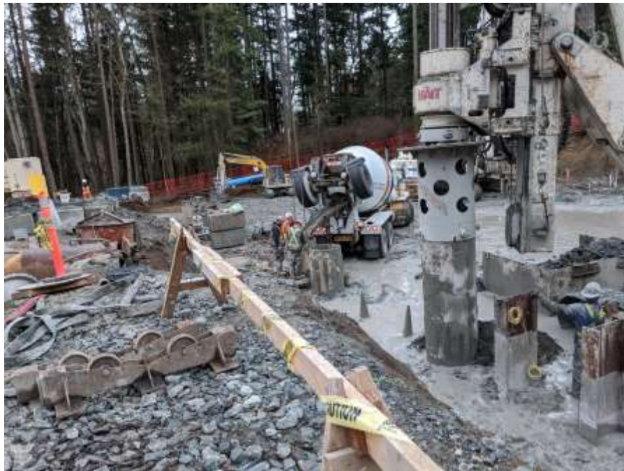
Figure 29– Arbutus Attenuation Tank –Concrete pour for piles and continued drilling.
