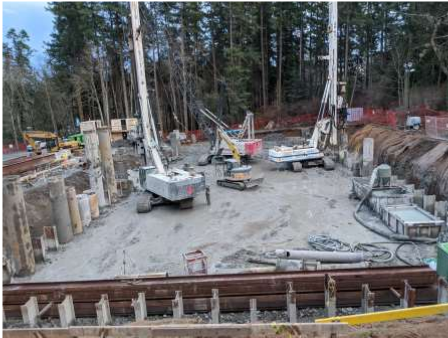
Figure 28–Arbutus Attenuation Tank- Second drill mobilised to site.
