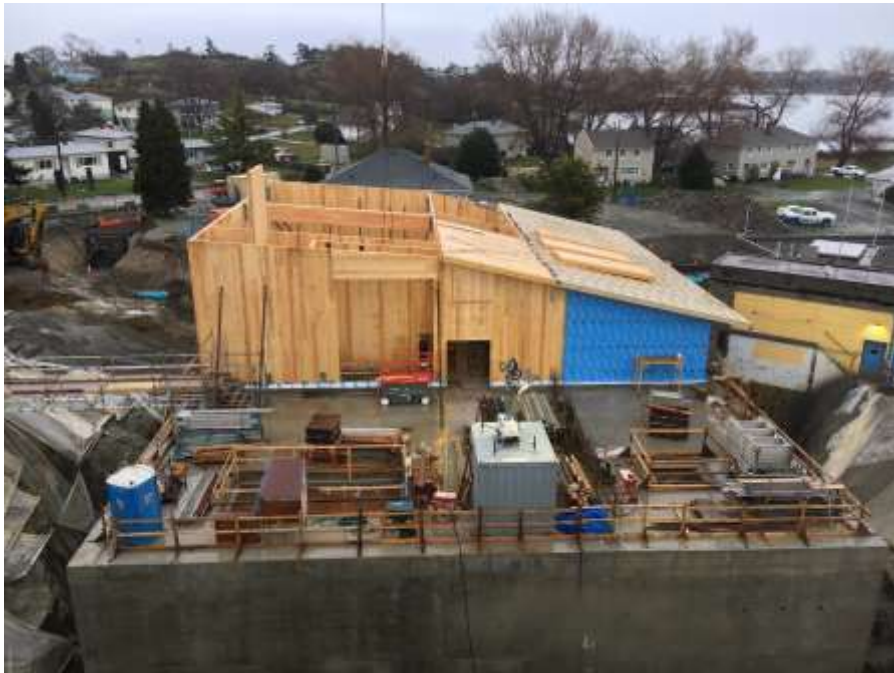
Figure 15–Macaulay Point Pump Station- Pump station progression, facing east.
