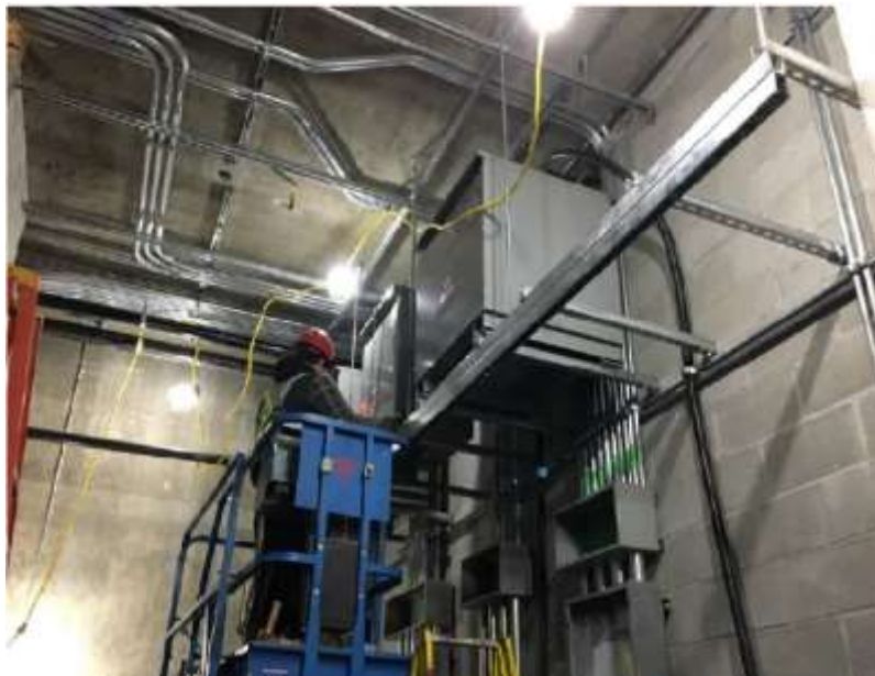
Figure 3– McLoughlin Point Wastewater Treatment Plant- Installing transformers in O&M electrical room.
