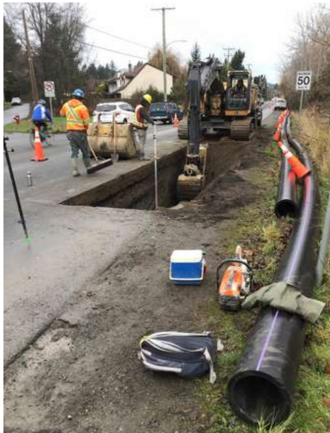
Figure 26 –Residual Solids Pump Stations – Commence pipe installation at Interurban Road.
