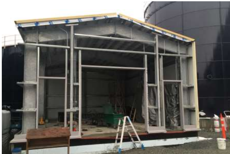
Figure 9– Residuals Treatment Facility- Installation of exterior insulated cladding on Equalization Building.
