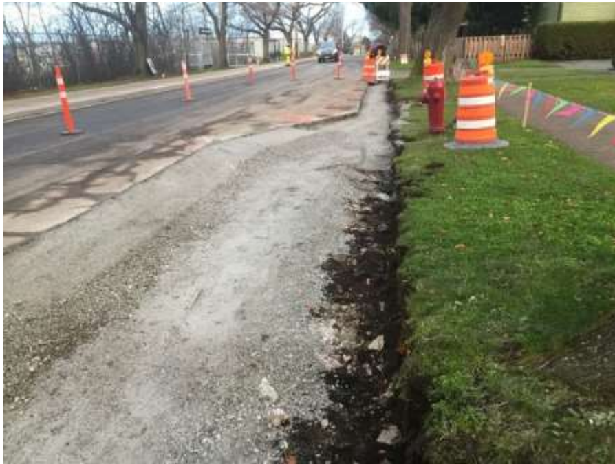
Figure 20–Clover Forcemain- Preparation for sidewalk and curb construction near Montreal St.
