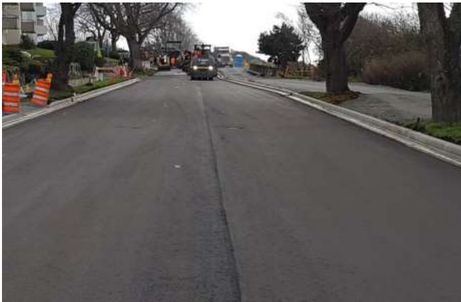
Figure 17–Clover Forcemain- Road restoration between Government St and Douglas St.
