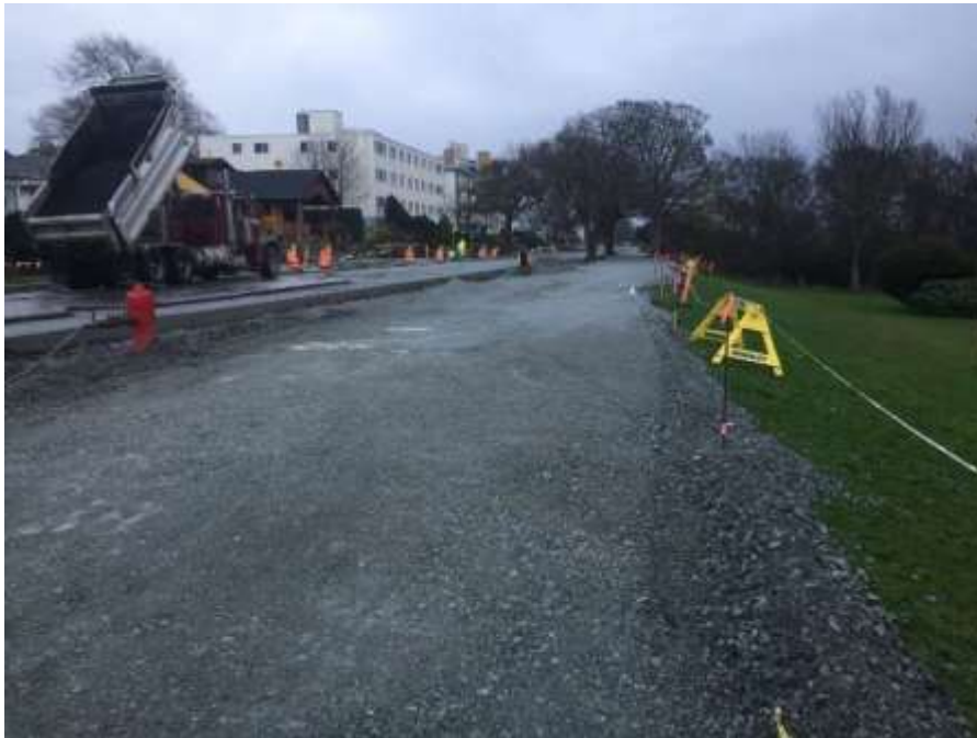
Figure 18–Clover Forcemain- Cycle track paving near Paddon Ave.
