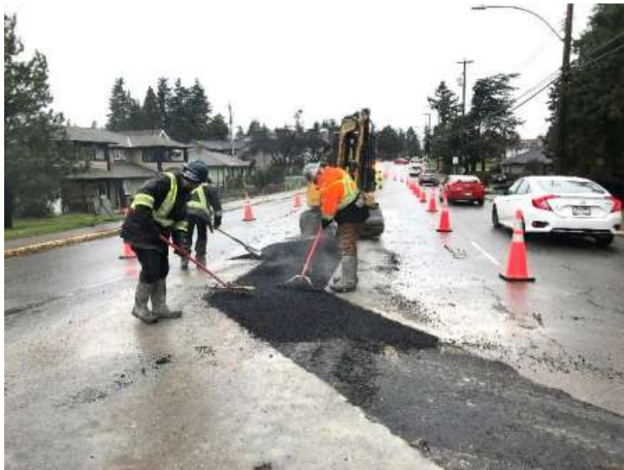
Figure 24--Residual Solids Pipes- Temporary paving on Tillicum Road at Selkirk Ave.
