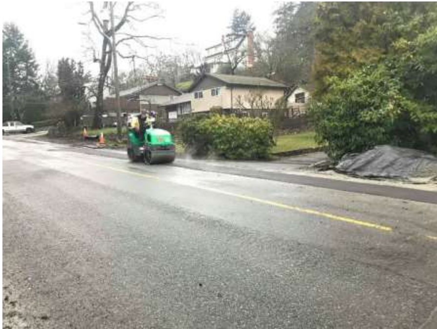
Figure 21—Residual Solids Pipes- Compacting asphalt on Interurban Road.
