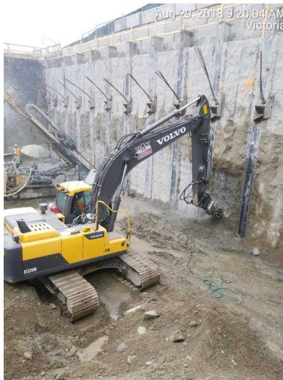
Figure 15 – Grinding concrete flush with king piles.
