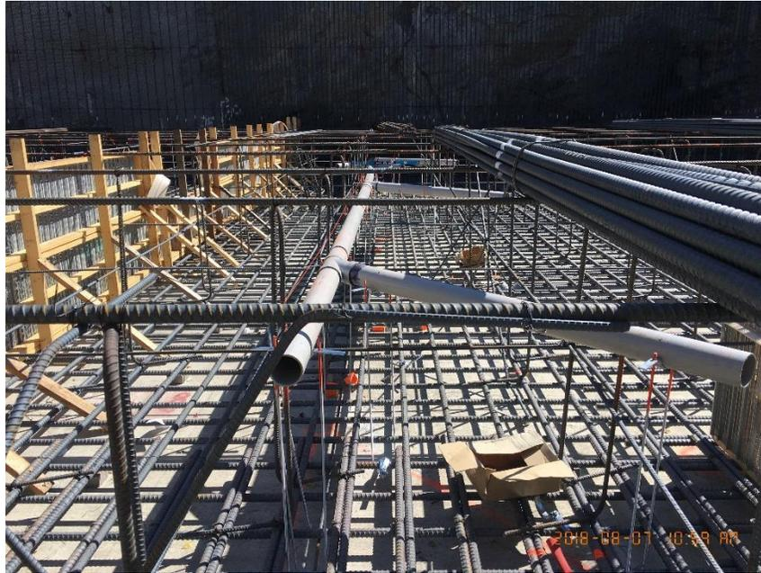
*Figure 4 – Setting floor drains in the tertiary slab.*
