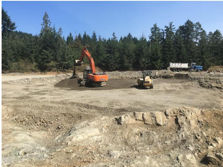
*Figure 10 – Spreading and compacting aggregate at digester #1 location.*
