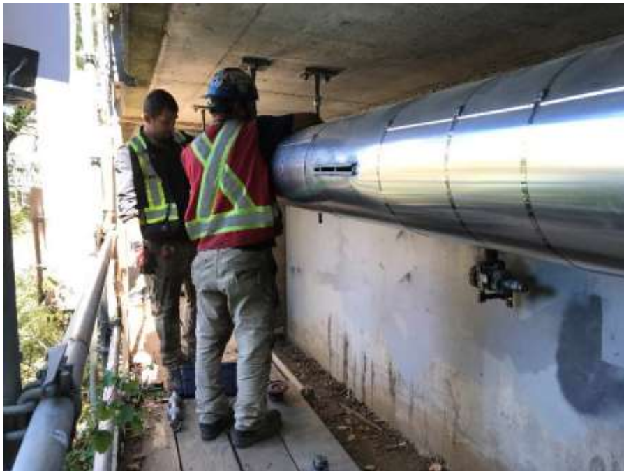
Figure 18–Residual Solids Pump Stations– Tillicum Bridge – Installing new hanger rods.
