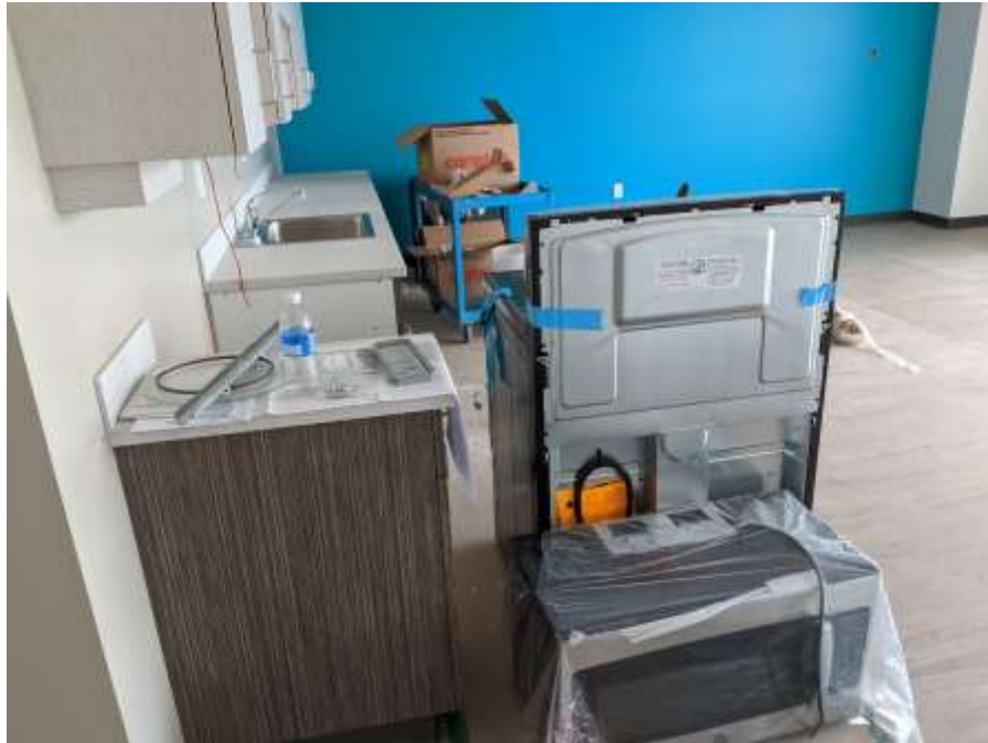
Figure 2– McLoughlin Point Wastewater Treatment Plant – appliances being installed
