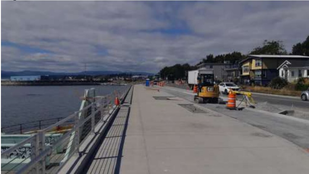
Figure 14–Clover Forcemain- new aluminium railing is installed and sidewalk ongoing
