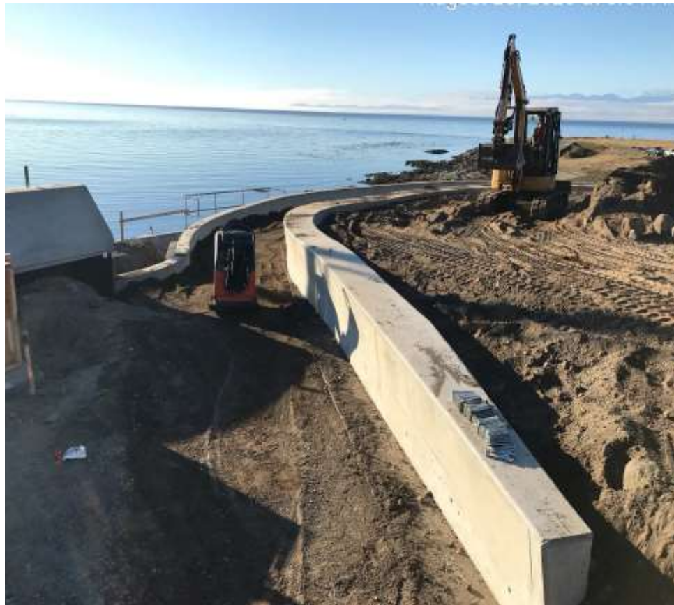
Figure 11- Clover Point Pump Station – Backfill and grading around the landscaping walls.
