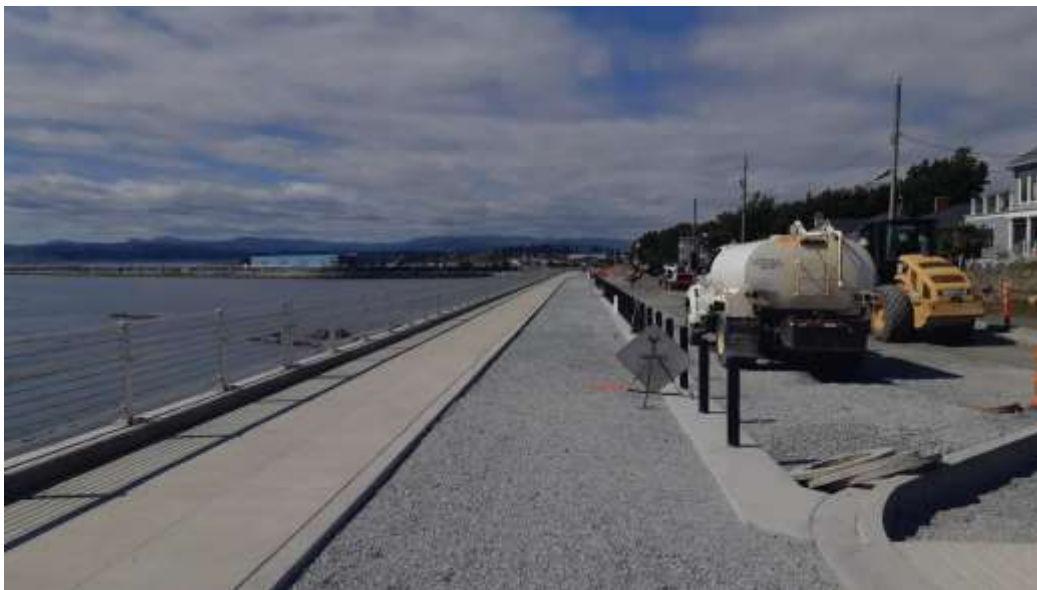
Figure 15–Clover Forcemain- Parking bollards installed.
