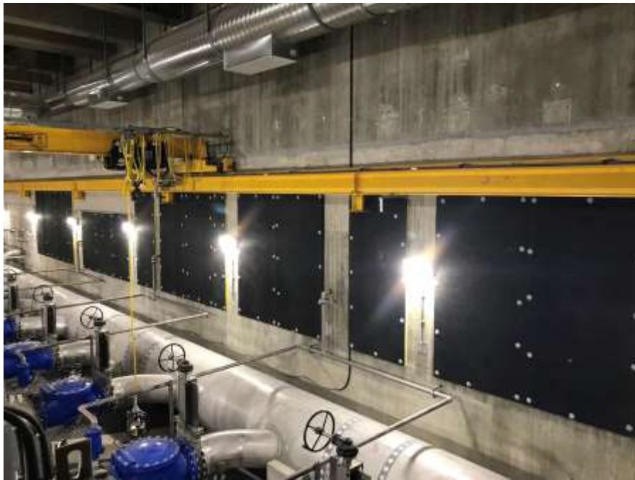
Figure 12–Macaulay Point Pump Station- Installation of acoustic panels in Drywell.
