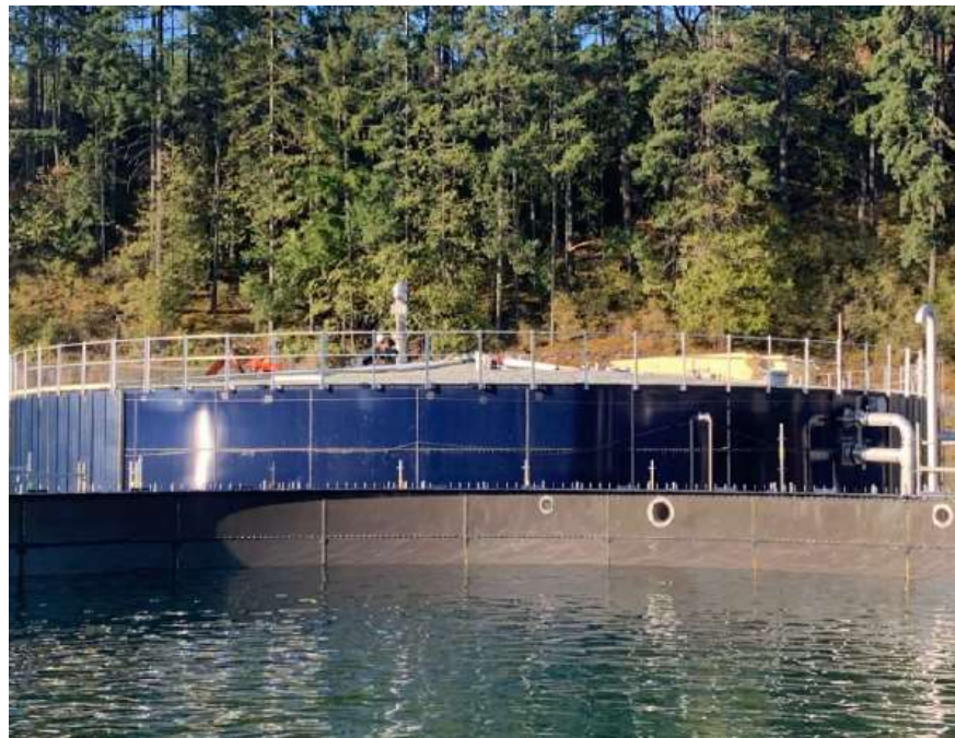
Figure 8- Residuals Treatment Facility – Filling of the Digested Solids Storage Tank.
