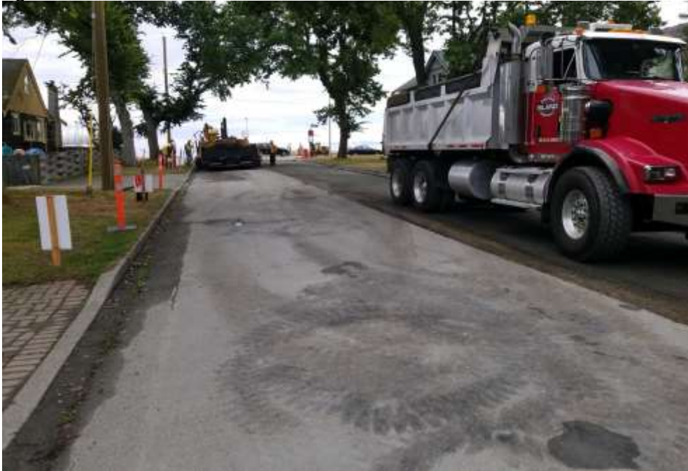
Figure 22–Trent Forcemain- base course paving on Eberts Street.
