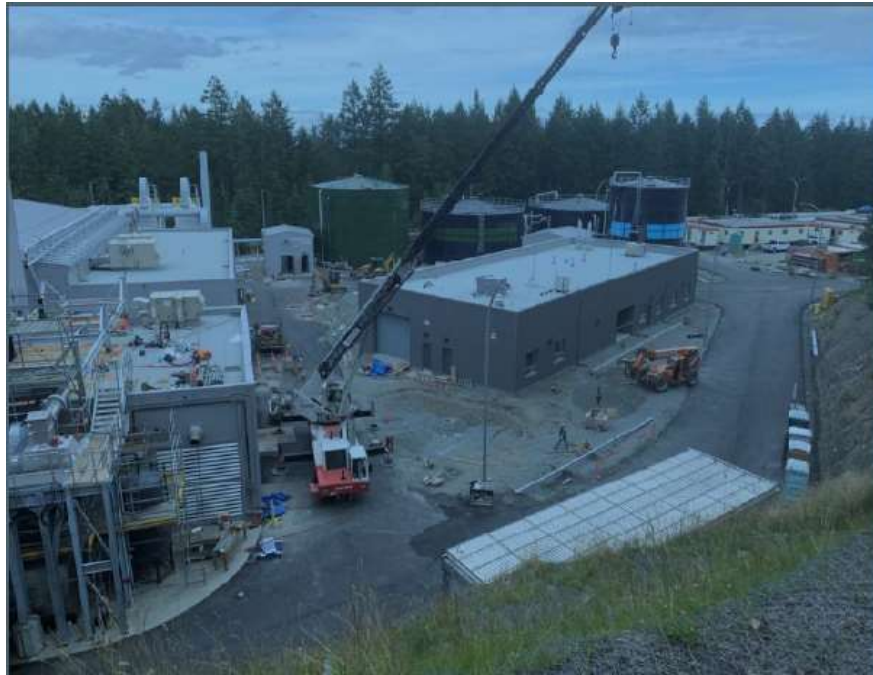
Figure 7- Residuals Treatment Facility- Operations building area.
