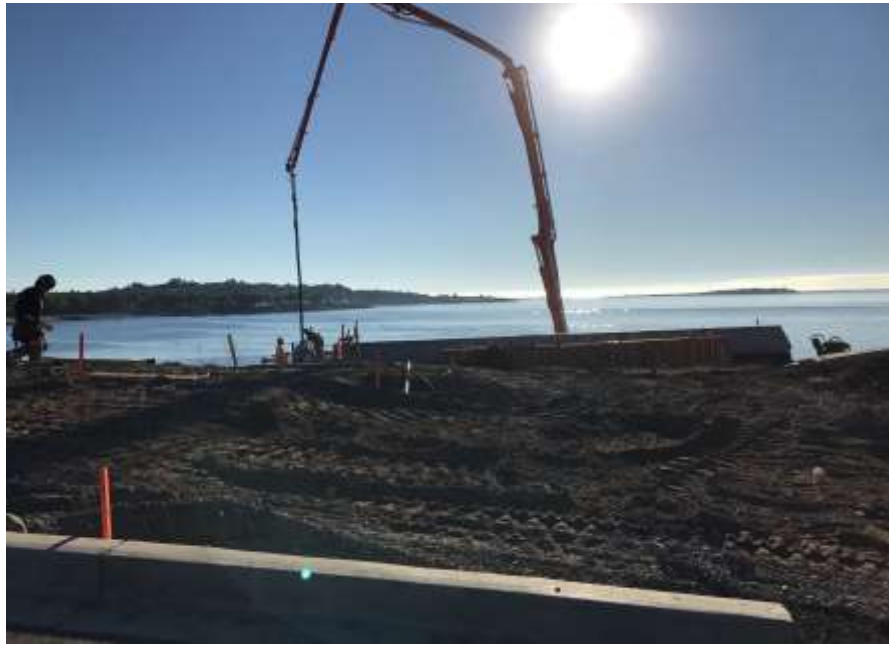
Figure 10–Clover Point Pump Station- concrete pour of north retaining wall.
