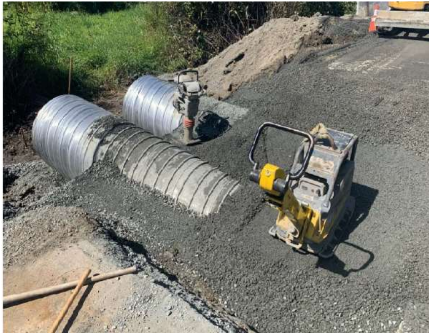
Figure 17-Residual Solids Pipes – Peers Creek – Backfilling and compacting of culverts.
