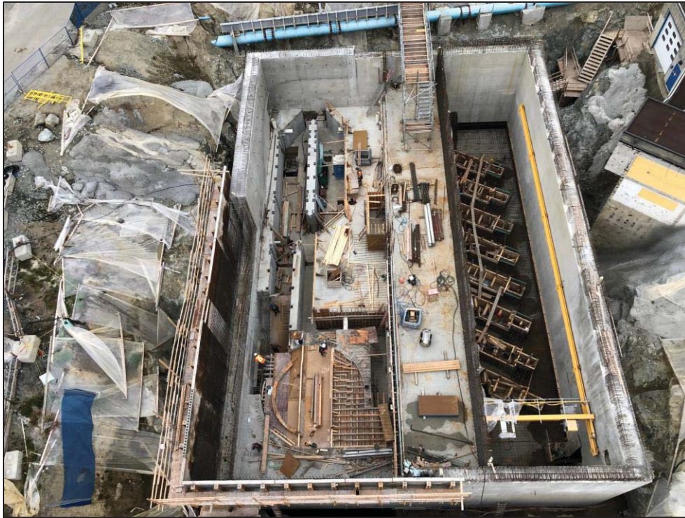
Figure 16–Macaulay Point Pump Station- pump station progression facing east.
