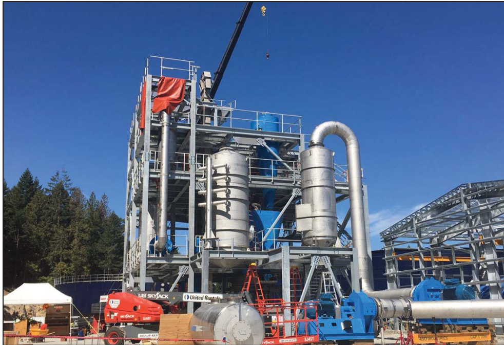
Figure 7- Residuals Treatment Facility- Crews installing dust collection cyclones in dryer building.
