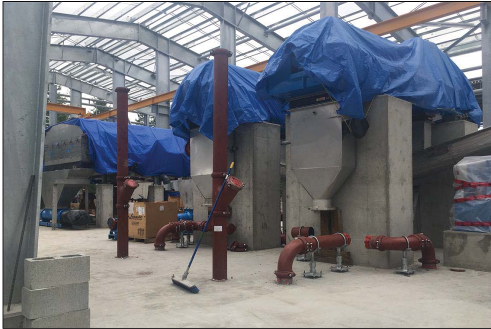
Figure 9- Residuals Treatment Facility- Installation of mechanical piping for centrifuges ongoing.
