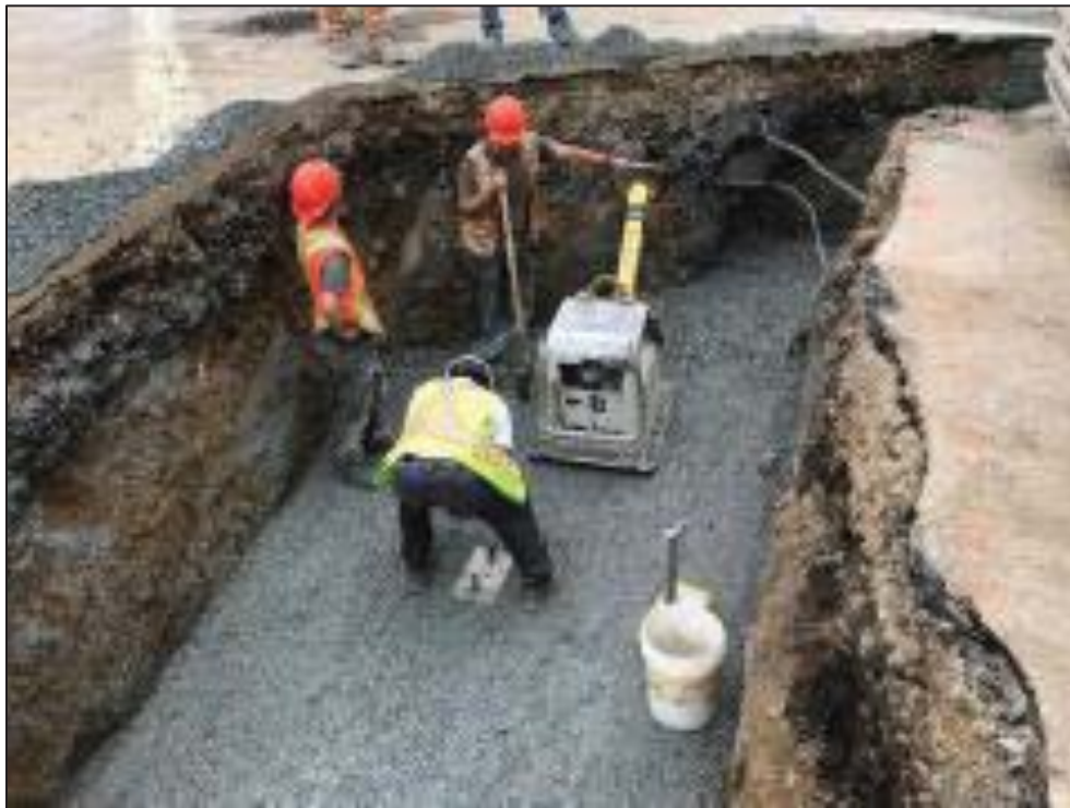
Figure 21–Residual Solids Conveyance Line- Compaction tests on Lyall Street.
