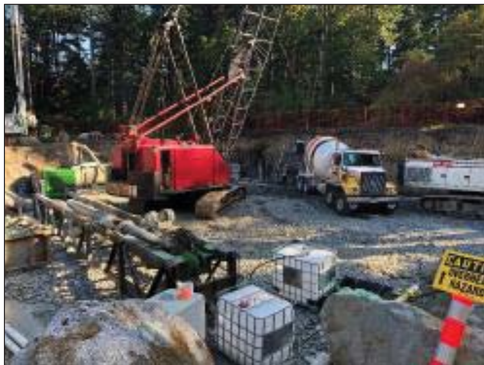
Figure 29– Arbutus Attenuation Tank – Placing concrete in Pile 85A
