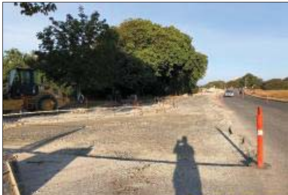
Figure 20—Clover Forcemain—Curb and gutter string set.
