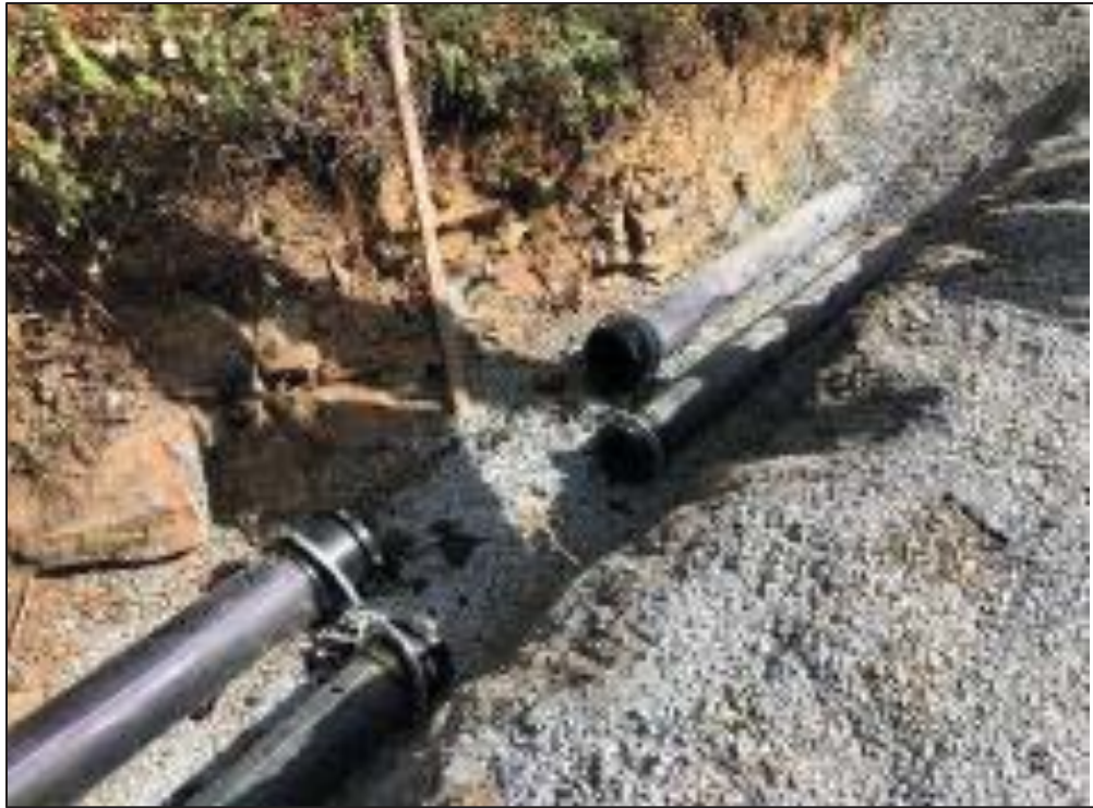
Figure 24–Residual Solids Conveyance Line- In ditch fusion welds completed at Interurban Trail.
