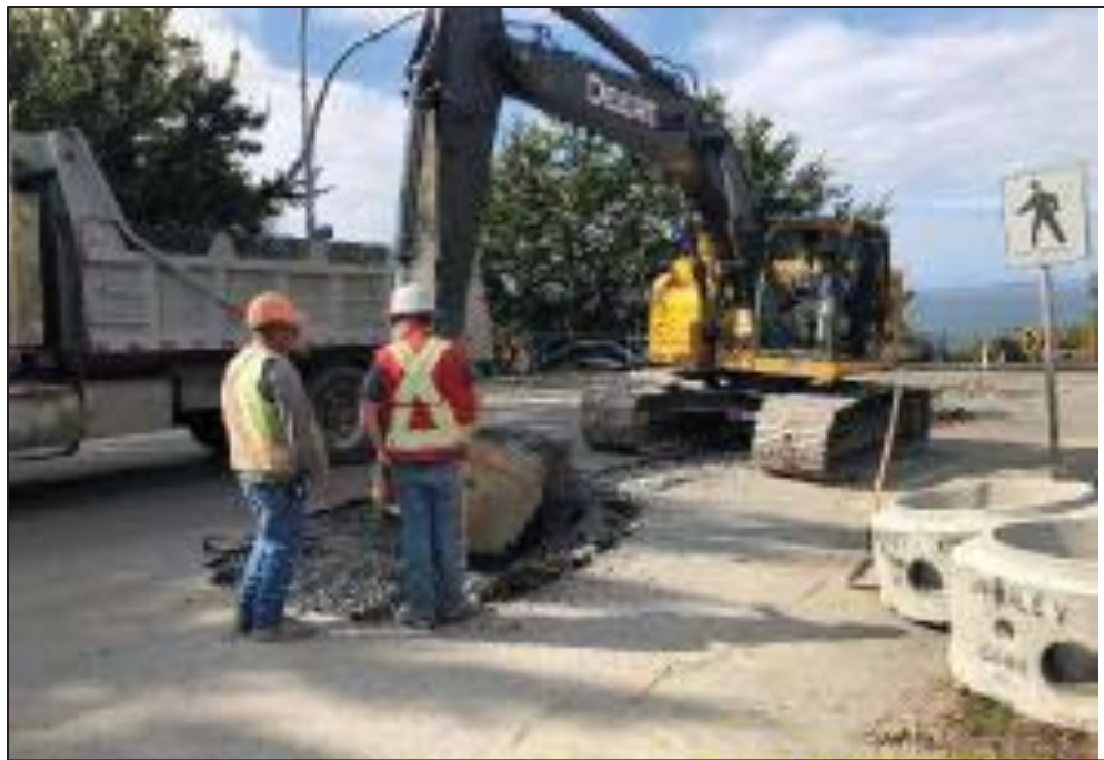
Figure 19—Clover Forcemain—commence excavation for City of Victoria sanitary main relocates.
