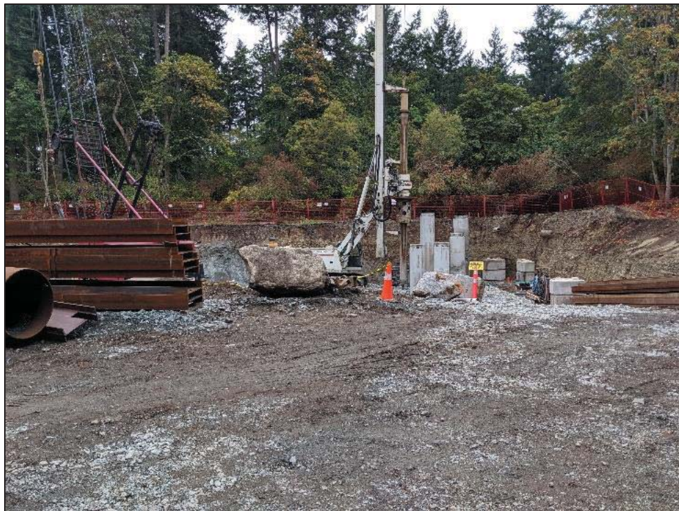
Figure 28–Arbutus Attenuation Tank- Drilling operation of Secant Pile
