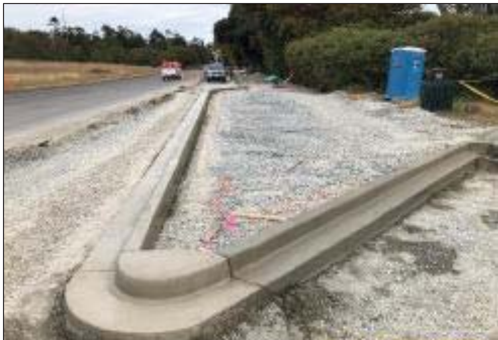
Figure 18–Clover Forcemain- Dallas Road curb and gutter installed
