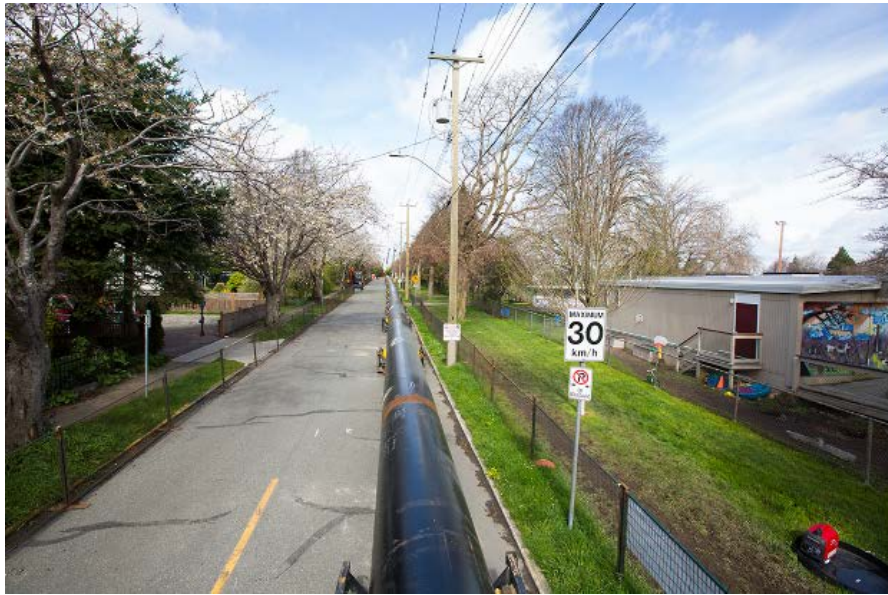
Figure 2 – Harbour Crossing pipe welded and assembled on Niagara Street
