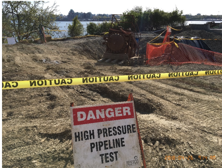
Figure 8 – Hydrostatic test in progress – the test passed.
