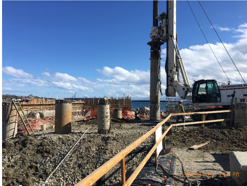
Figure 4 – Drilling piles in the BAF area
