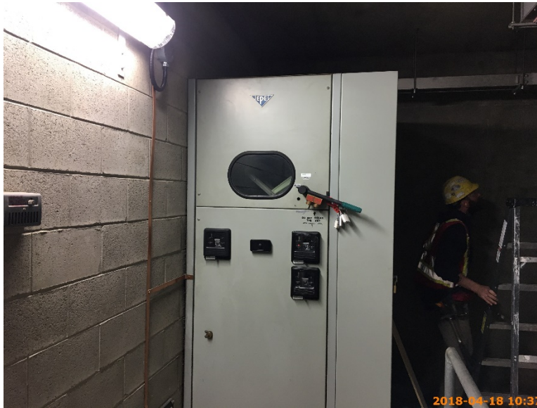
Figure 11 – Existing permanent power locked out to switch over to temporary power.
