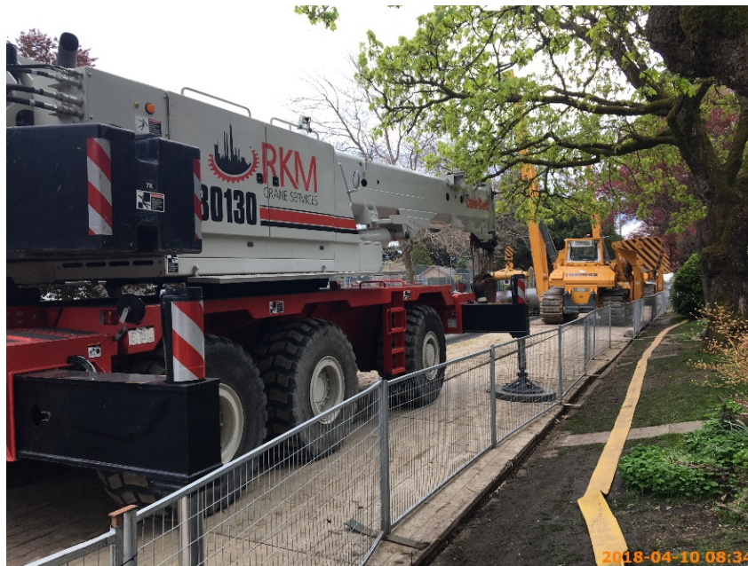
Figure 5 – Mobilizing equipment for the Pipe Pull.
