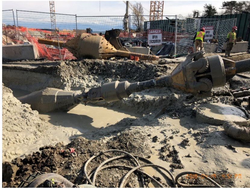
Figure 6 – Pipe pull complete, coming out at McLoughlin side
