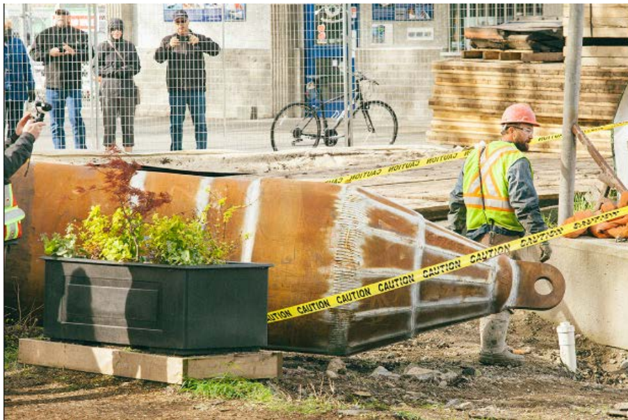
Figure 3- Pull head to be welded on to Harbour Crossing Pipe.
