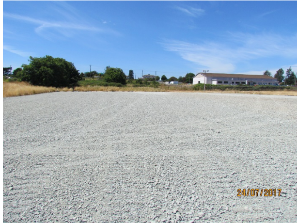
Figure 3- Employee parking lot constructed at DND Area "E"
