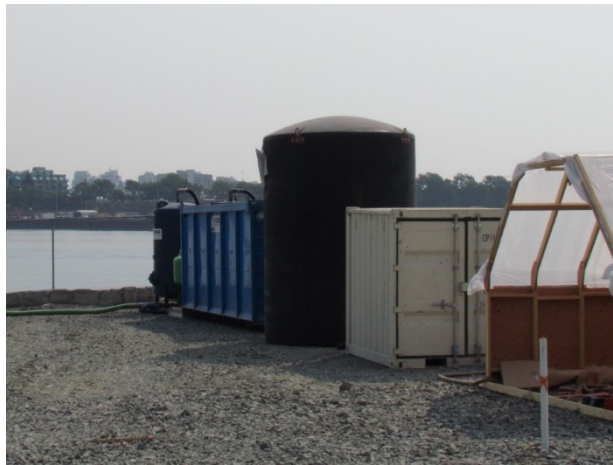
Figure 4 - Installation of water treatment plant
