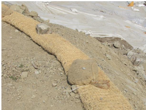
Figure 5 – Erosion and sediment control in place
