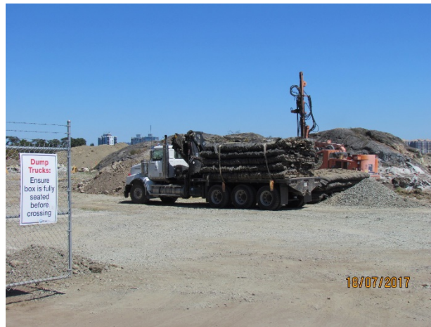
Figure 1- Mobilization of blasting equipment
