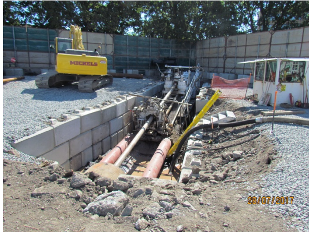
Figure 6 – Drilling of HDD pilot hole
