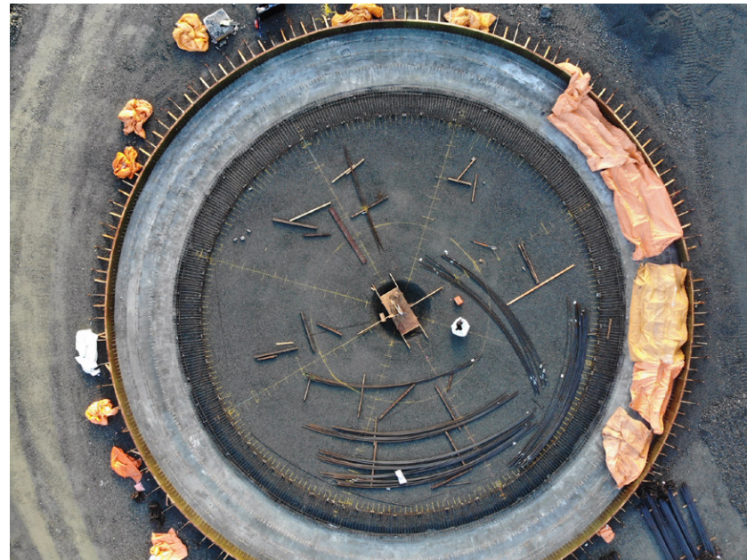
Construction of a digester at the Residuals Treatment Facility.
