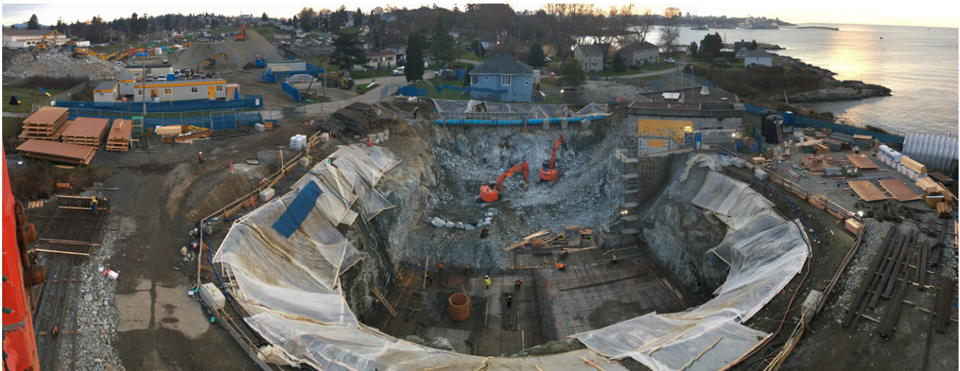
Aerial view of construction progress at the Macaulay Point Pump Station.
