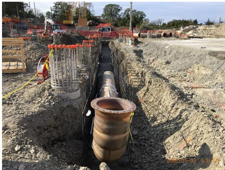
*Figure 3- Installation of under slab pipe*
