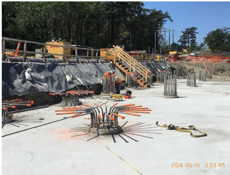
Figure 5 – Cleaning of pile tops and bending pile rebar in West BAF
