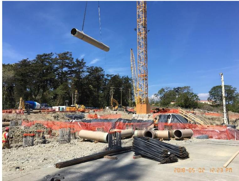
*Figure 2 – Staging of under slab BAF piping*
