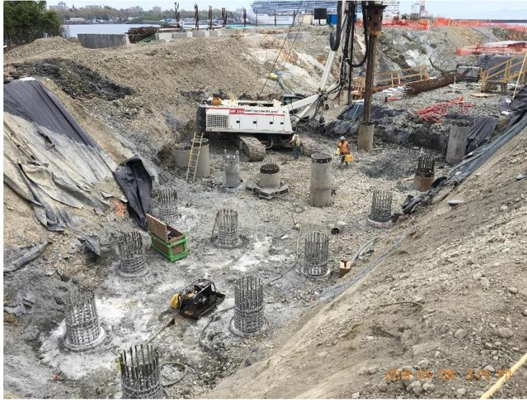
Figure 4 – Installation of foundation piles in odour control area
