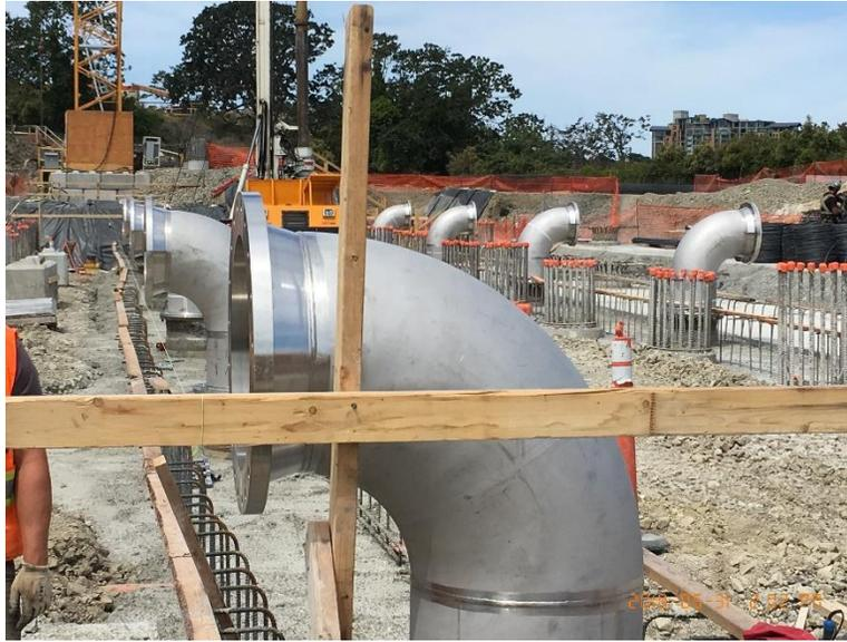
*Figure 8 – Install & align stainless steel risers in West BAF drain*
