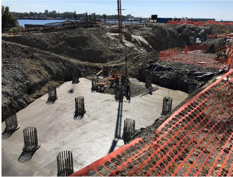
*Figure 6 – Placing concrete mud slab in odour control area*
