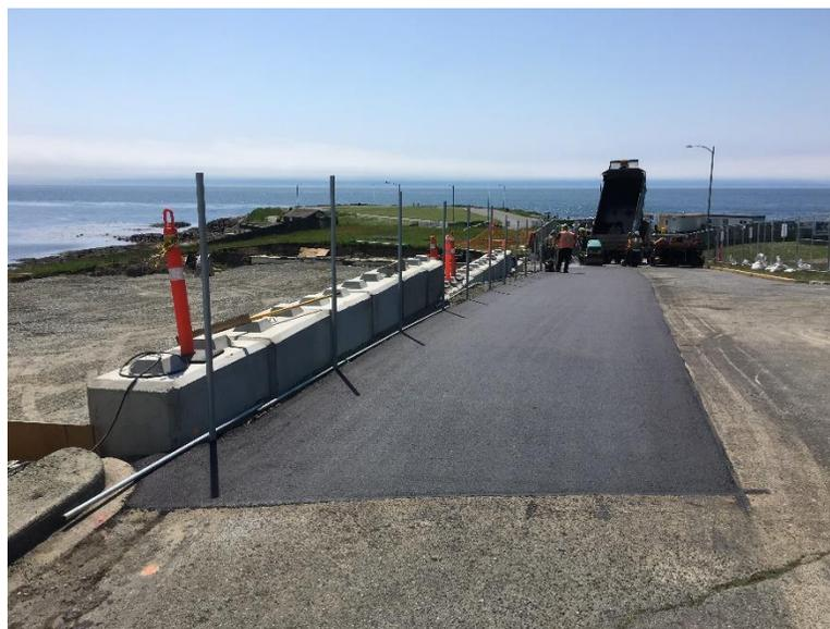
*Figure 10 – Re-install asphalt and fencing along Clover Point Road*
