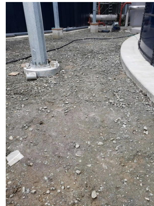
Photo 16 • Spill Pathway after spill clean-up
