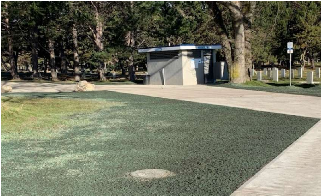
Figure 15-Trent Forcemain- Seeding along Memorial Avenue.
