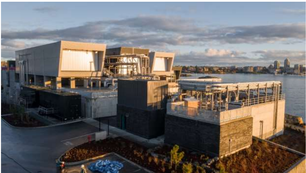
Figure 4- McLoughlin Point Wastewater Treatment Plant- Site view looking east
