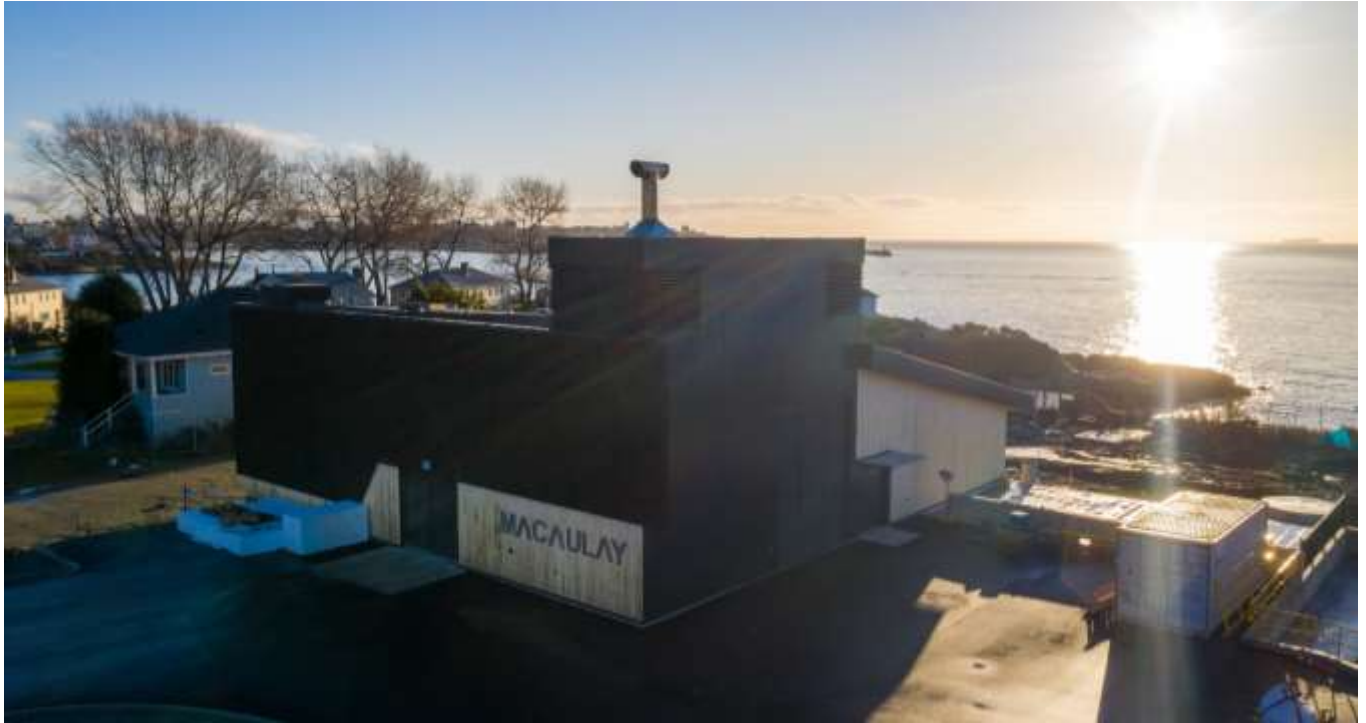
Figure 9–Macaulay Point Pump Station
