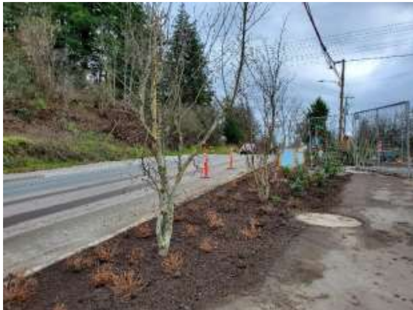
Figure 12 –Residual Solids Pump Stations – Pump Station Landscaping
