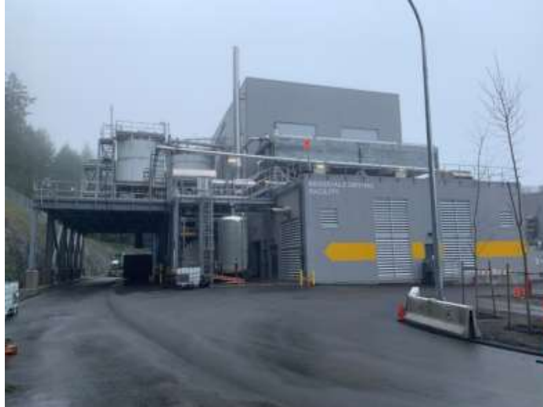
Figure 5- Residuals Treatment Facility- Residuals Drying Facility Building
