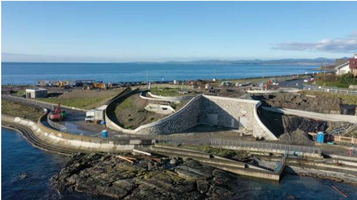
Figure 8–Clover Point Pump Station- Site Overview
