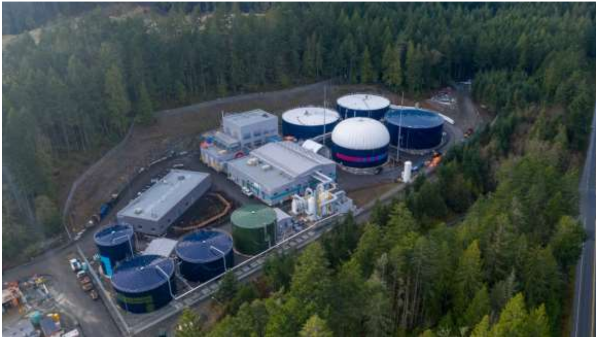
Figure 6– Residuals Treatment Facility- Aerial view of RTF
