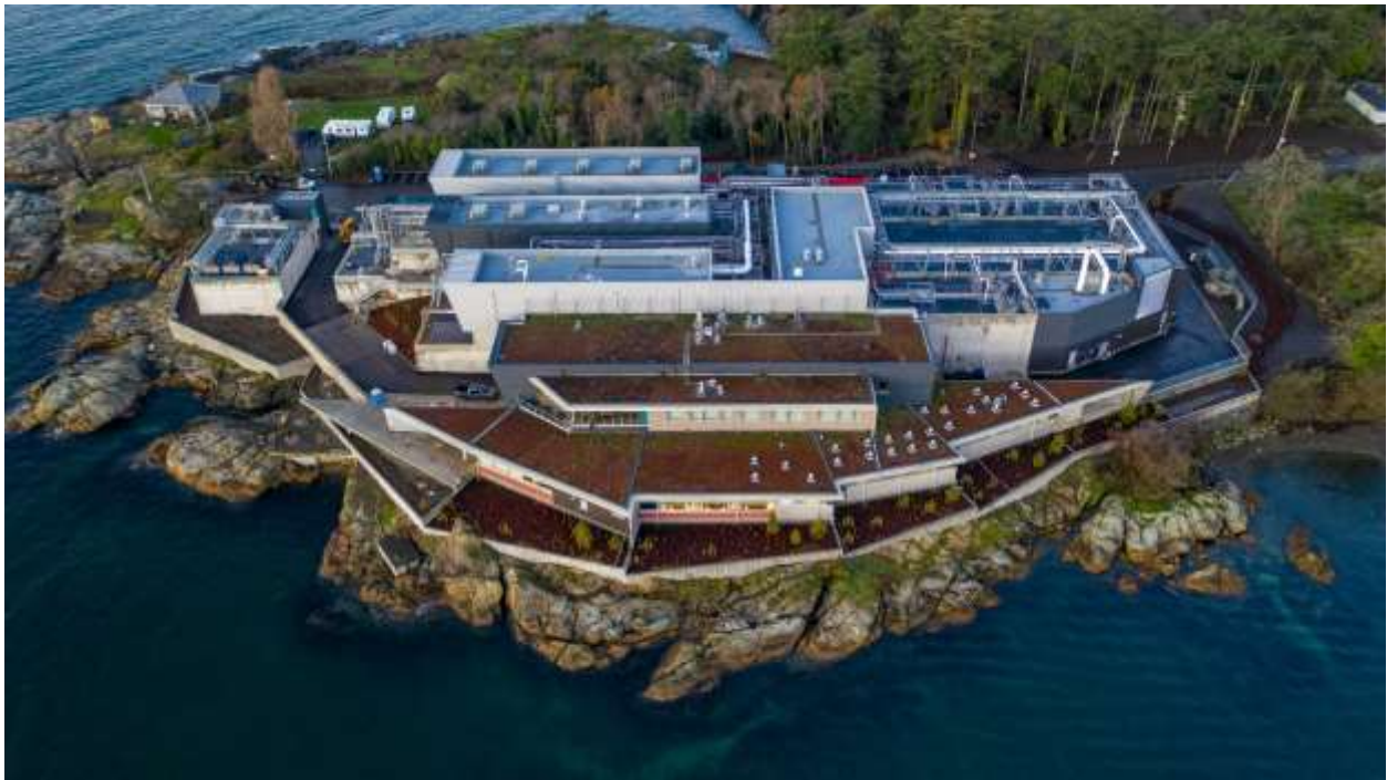
Figure 3- McLoughlin Point Wastewater Treatment Plant- Aerial view of plant
