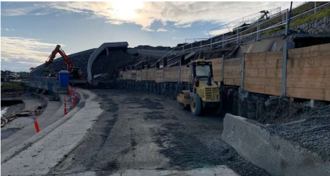
Figure 16-Trent Forcemain- Work area by Seawall
