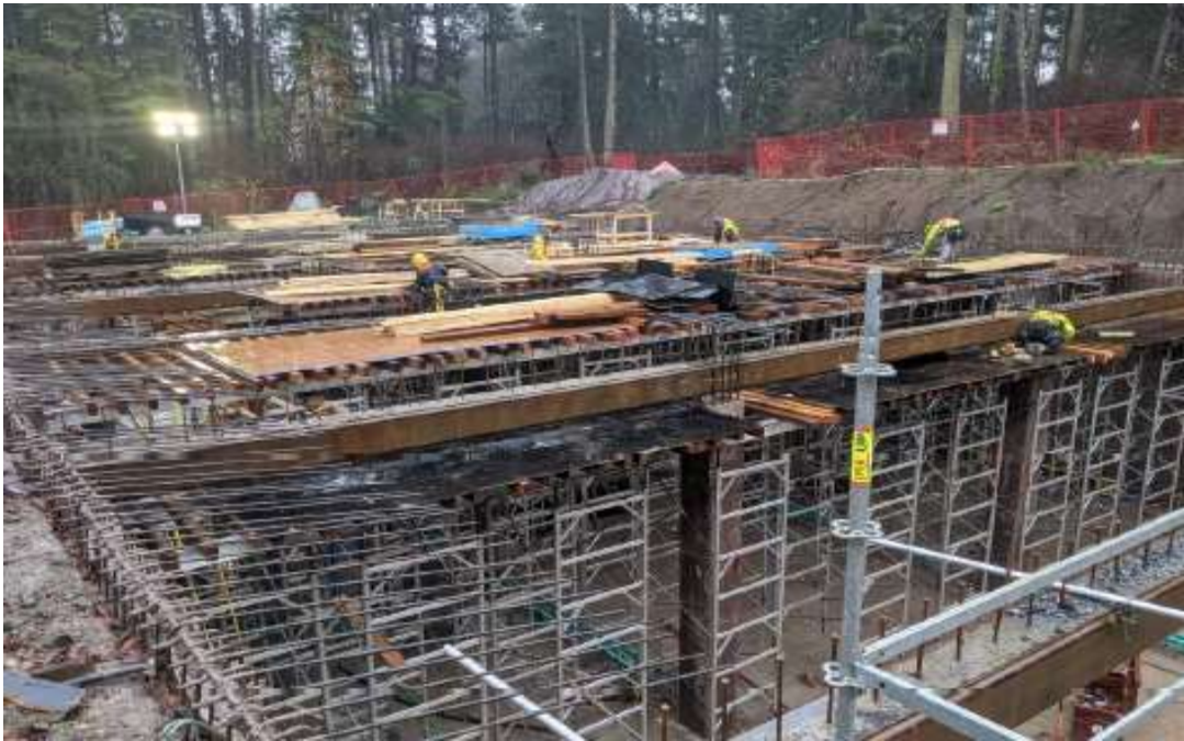
Figure 13–Arbutus Attenuation Tank- View of Tank looking south
