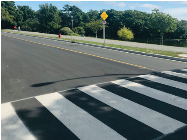
New crosswalk at Government Street on the newly paved Dallas Road.
