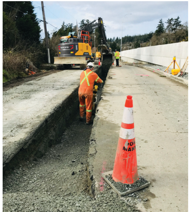
Pipe installation on Portage Road in Saanich.
