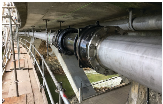
The pipe has been installed under the Gorge Bridge on Tillicum Road.
