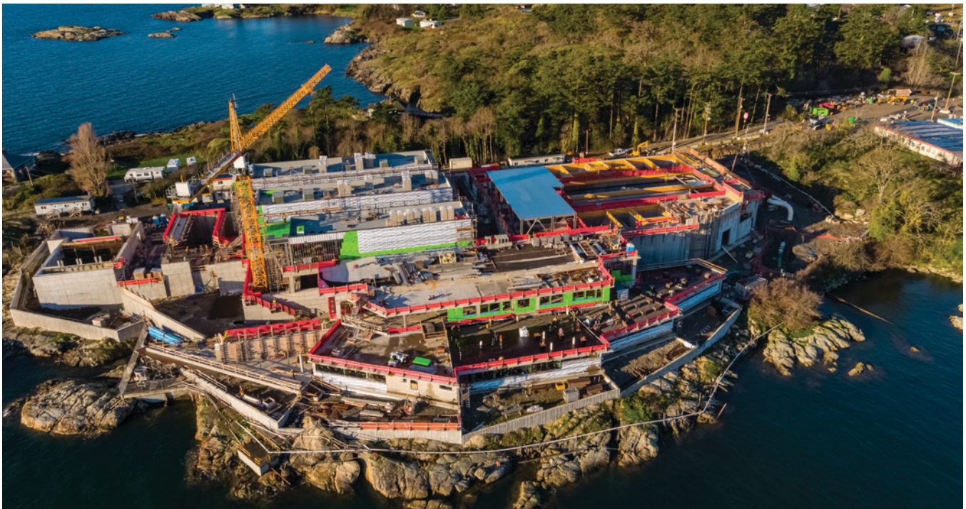
Aerial view of McLoughlin Point Wastewater Treatment Plant.
