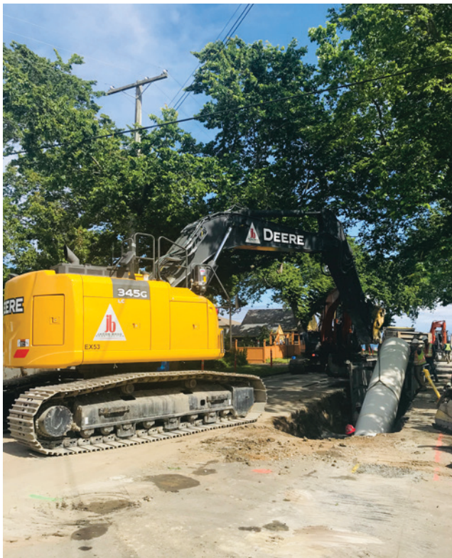
A section of pipe being installed for the Trent Forcemain.
