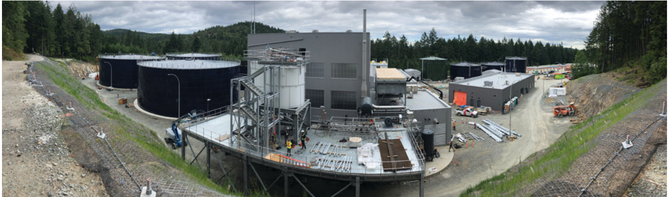
Construction progress at the Residuals Treatment Facility.
