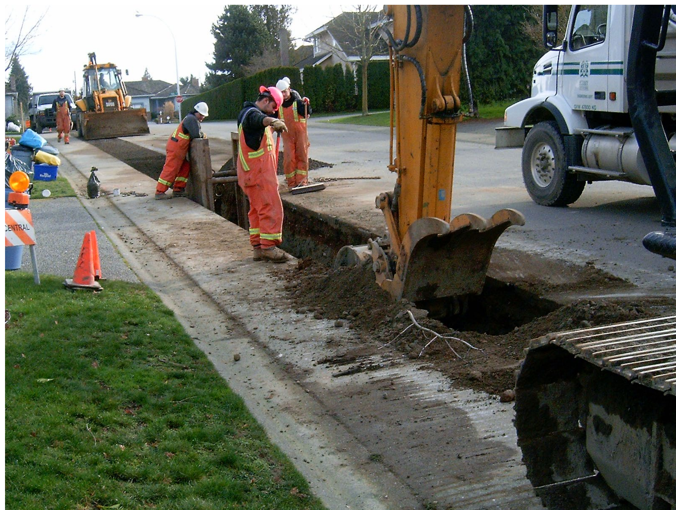
Conveyance pipe installation
