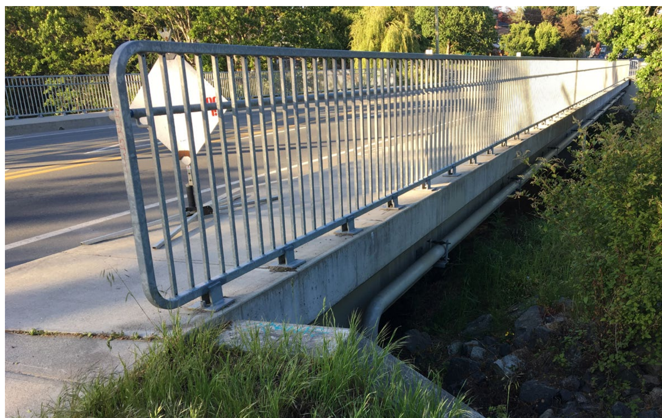
Conveyance pipe on bridge
