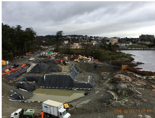
Figure 3- View looking north from the tower crane
