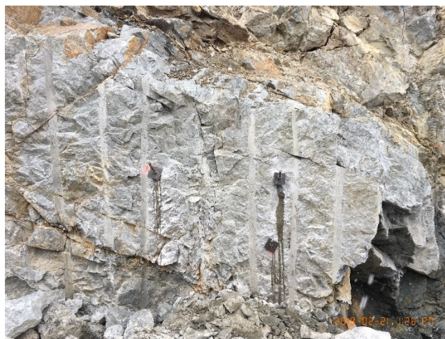
Figure 7 – Install rock anchor bolts at outfall
