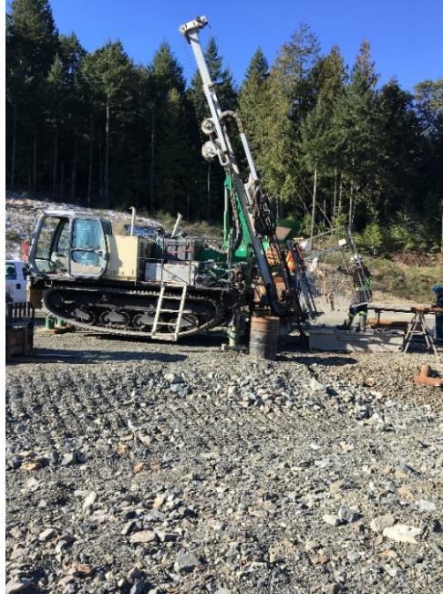
Figure 9 - Geotechnical Drilling Operation
