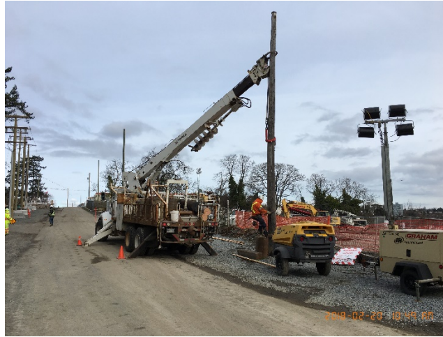
Figure 8 – Remove old utility poles from East side of Victoria View Road
