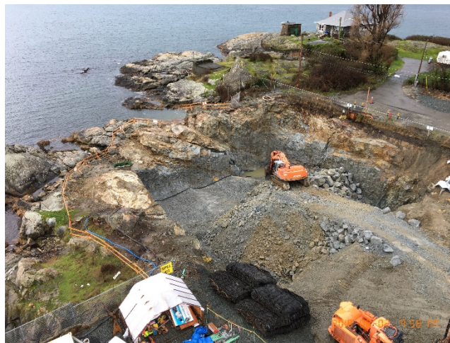
Figure 4 – View of the outfall shaft area from the tower crane
