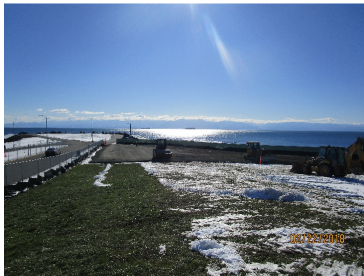
Figure 12 – Installation of gravel base at Office/laydown compound
