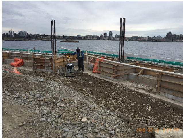
Figure 5 – Compaction of crushed rock backfill at tsunami wall
