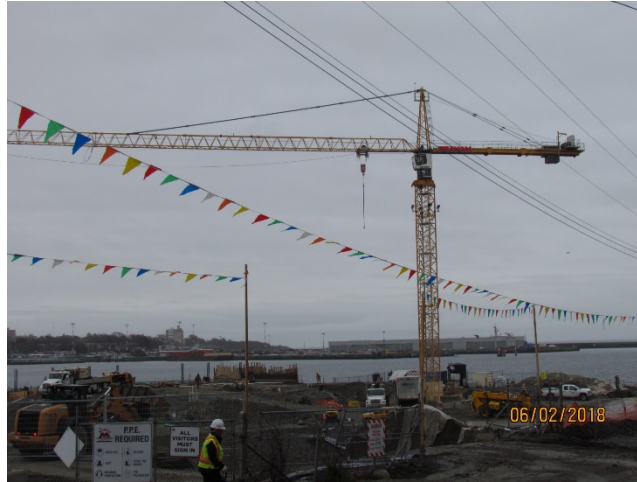
Figure 2 – Tower crane erection complete
