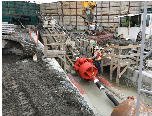
Figure 6 – Installing 54" reaming bit at Ogden Point
