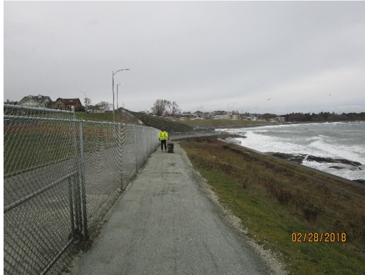
Figure 11 – Compacting temporary seawall walking path
