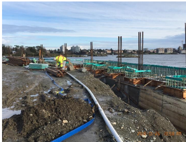
Figure 3- Forming and rebar for tsunami wall
