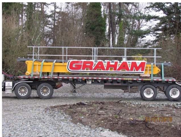
Figure 7 – Transporting jib section for erection
