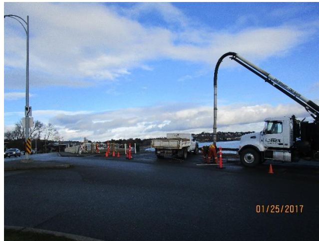
Figure 8 – Daylighting existing duct bank at Clover Point
