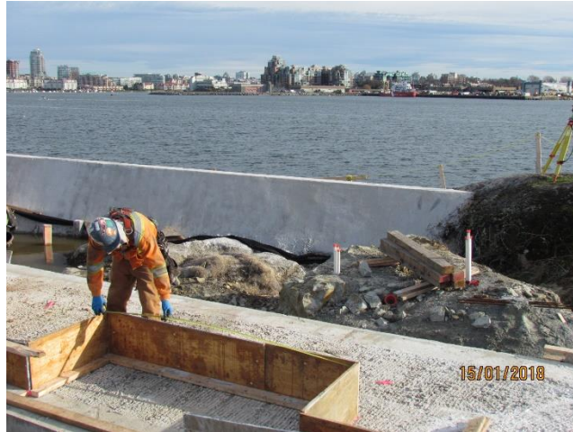
Figure 2 – Forming of tsunami wall foundation
