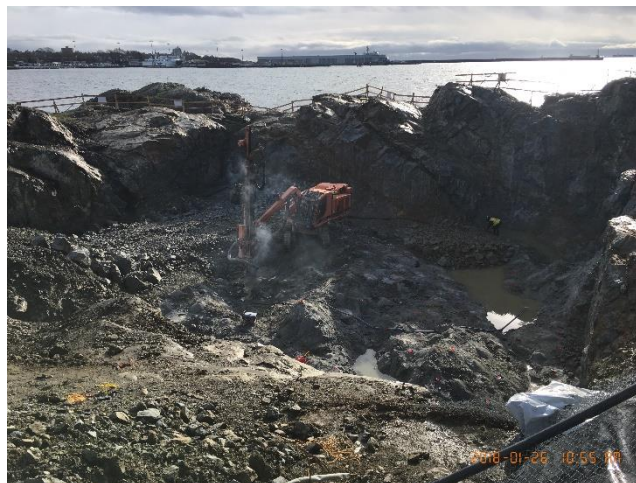
Figure 4 – Drilling for blast in outfall area
