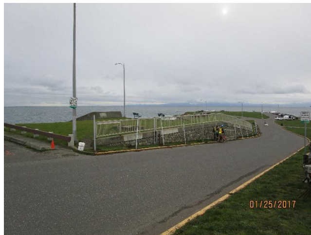
Figure 9 – Installing fence post at Clover Point pump station site compound
