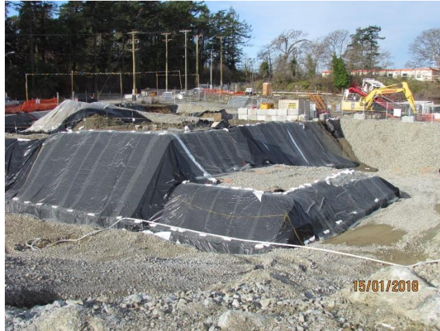
Figure 5 – Slope stabilization
