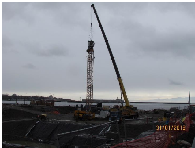
Figure 6 – Placing cabin on tower section
