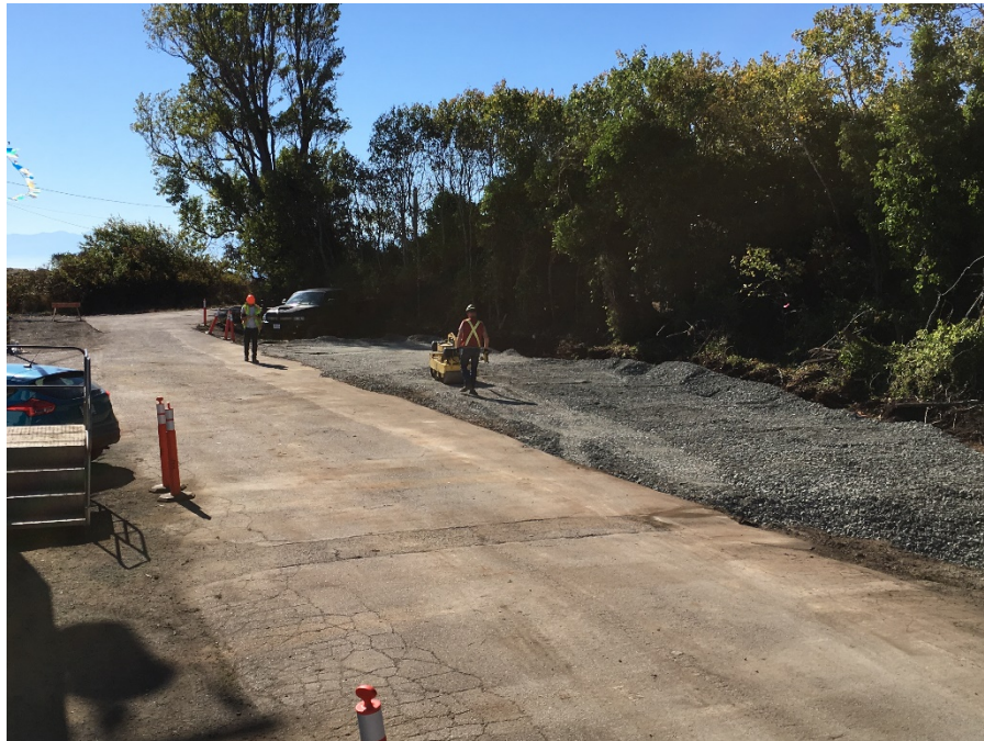
Figure 9 – Place and compact aggregate at BC Hydro right-of-way
