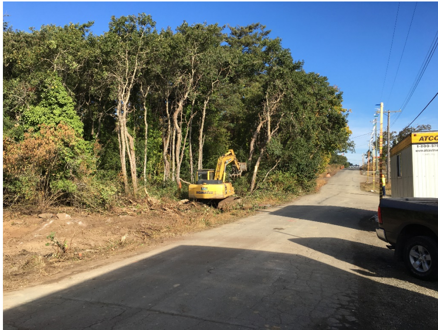
Figure 7 - Clearing and grubbing BC Hydro right-of-way
