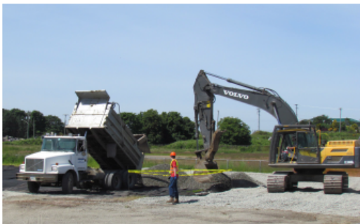
Crews placing aggregate in a laydown area for the McLoughlin Point Wastewater Treatment Plant in Esquimalt.
