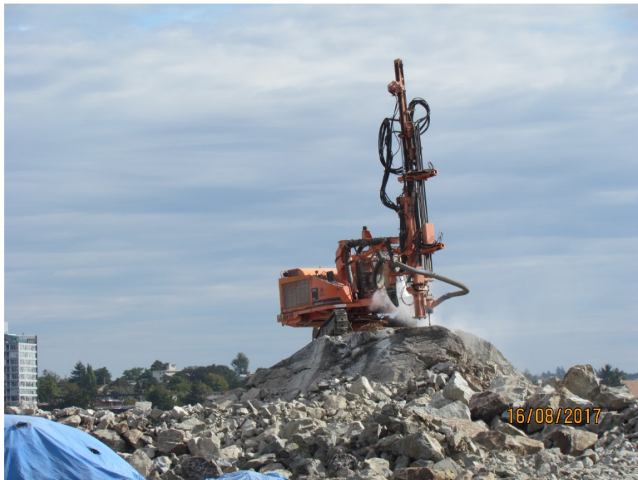
Figure 3 - Drilling and blasting at McLoughlin Point
