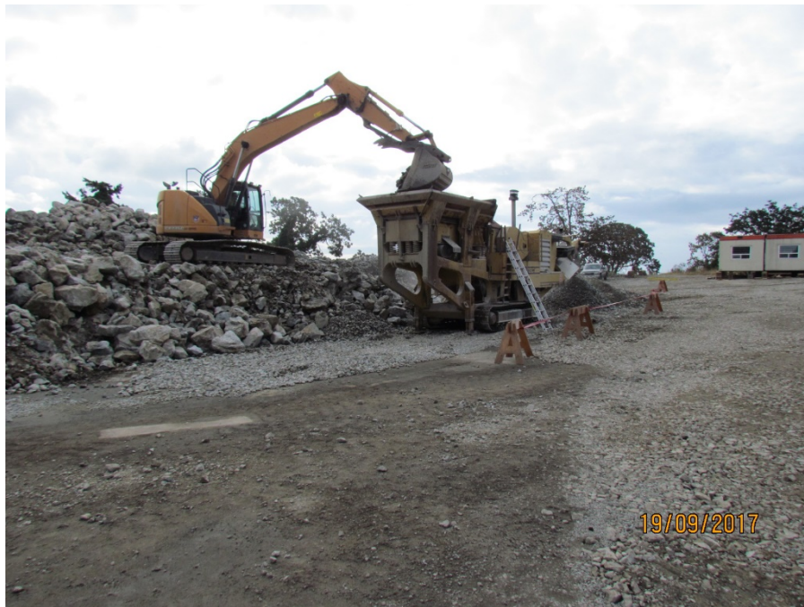
Figure 4 - Crush blast rock in area A
