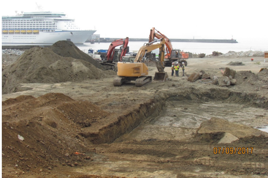
Figure 5 - Excavate contaminated materials
