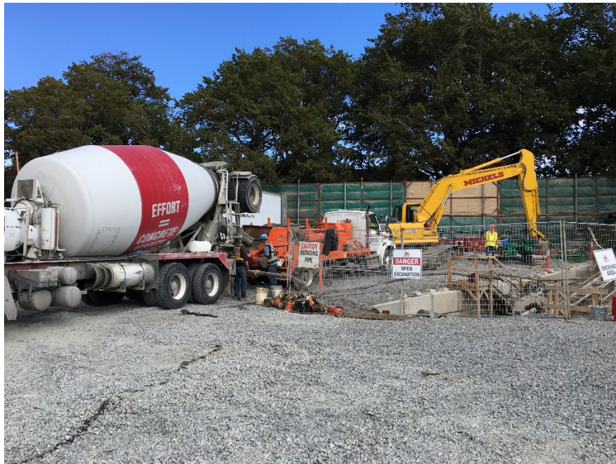
Figure 10 – Grout pumped in pilot hole to seal fissure
