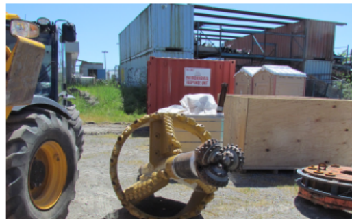
The horizontal directional drill bit being used to drill the hole for the cross-harbour undersea pipe that will go from Ogden Point to McLoughlin Point.
