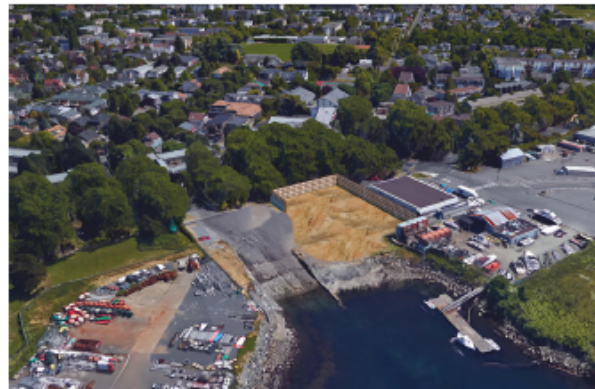
Noise Wall – Aerial view
