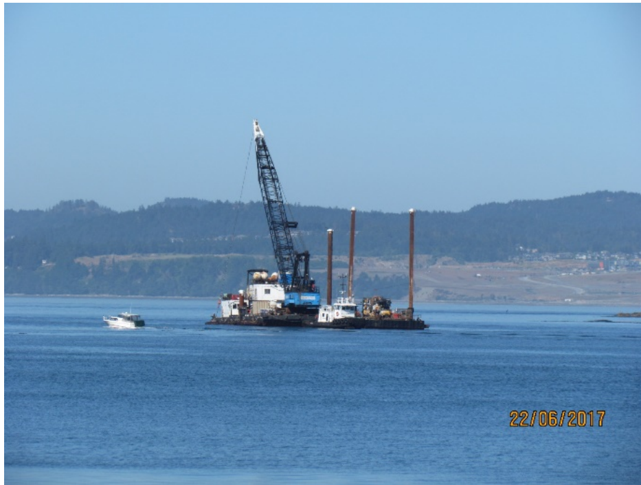
Figure 7- Marine geotechnical investigation for outfall
