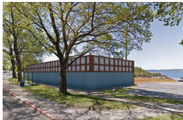
Noise Wall – Street view
