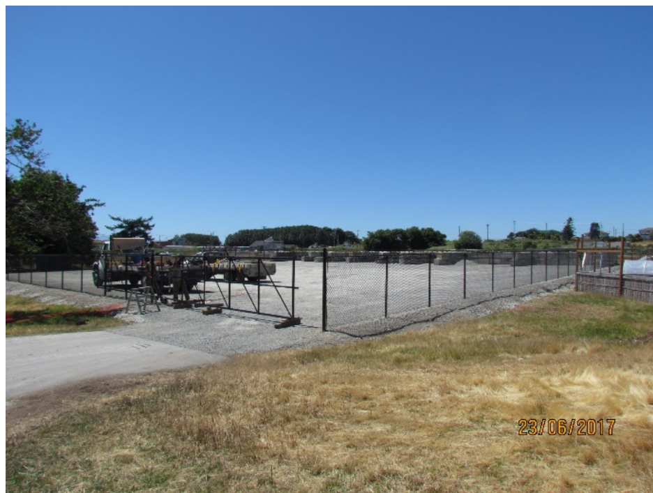
Figure 6- DND temporary works yard
