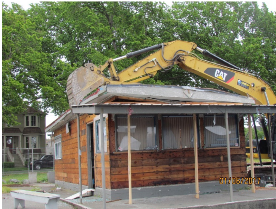
Figure 8- Demolition of angler's hut
