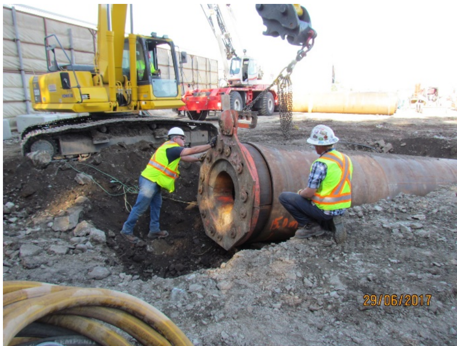
Figure 10- Installing hammer die in HDD casing
