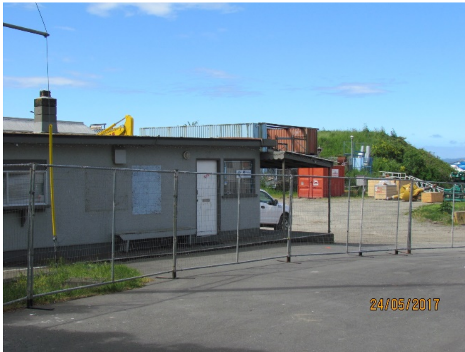
Figure 5- Temporary fencing installed
