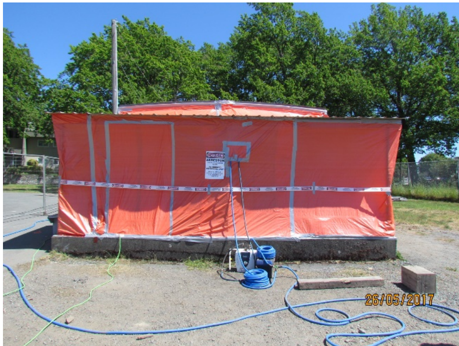
Figure 2- Negative air pressure asbestos enclosure
