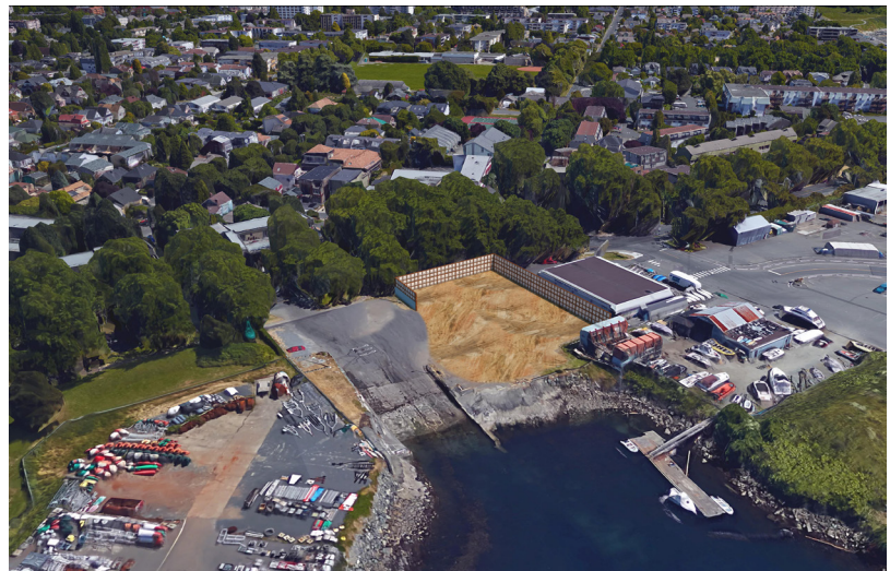
Noise Wall – Aerial view
