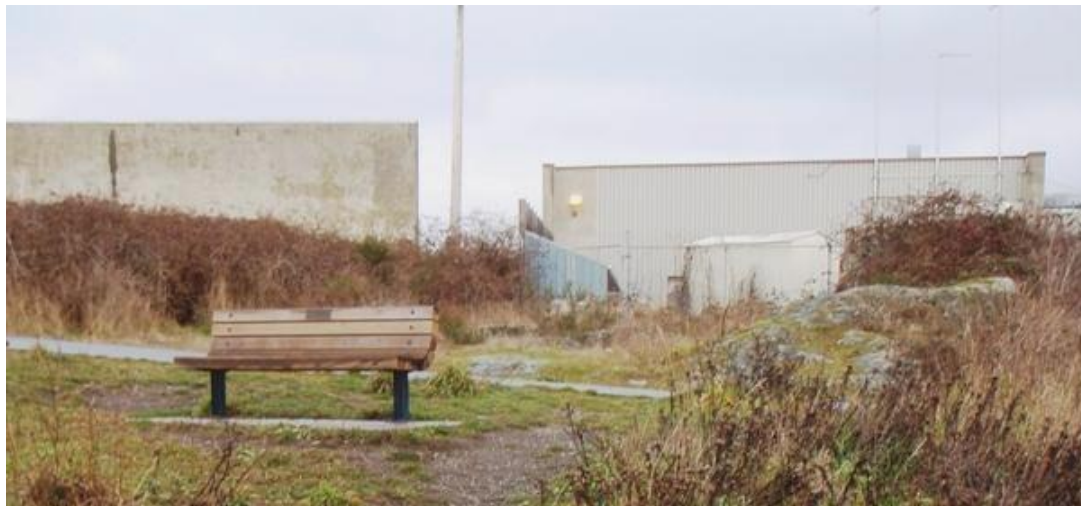
Figure 5-15. Southwestern edge of the Macaulay Point pump station between existing facility and walkway; note bedrock outcrop in foreground
