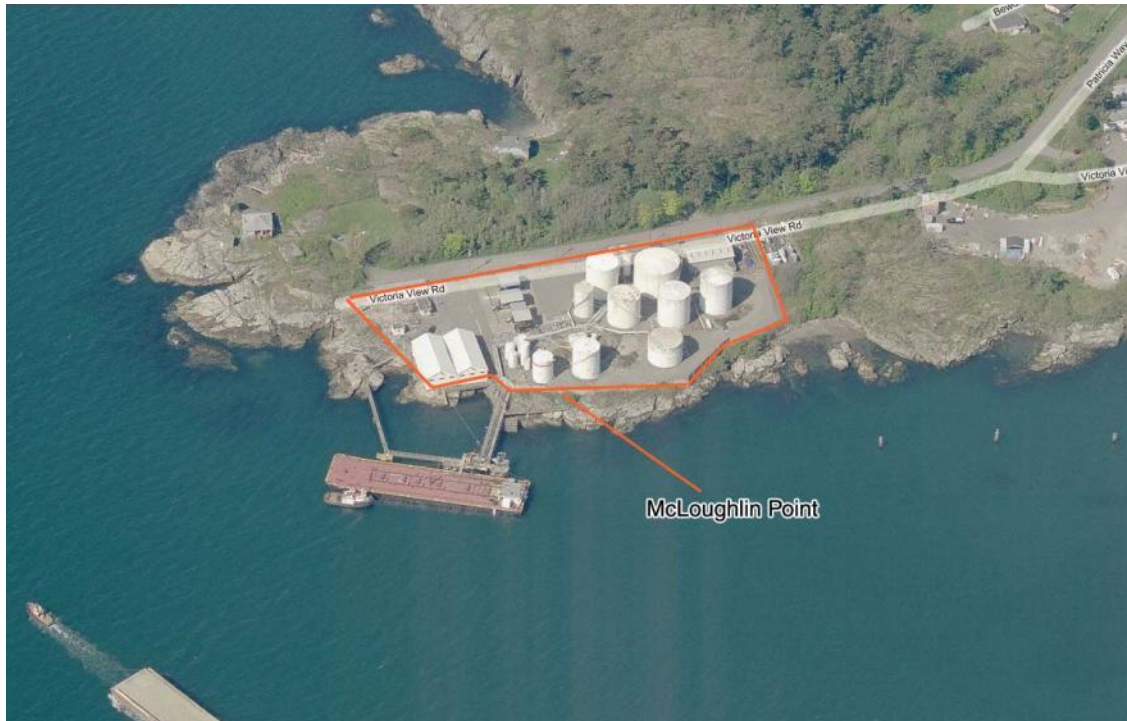
Figure 5-40. McLoughlin Point site before fuel tank decommissioning in 2008
