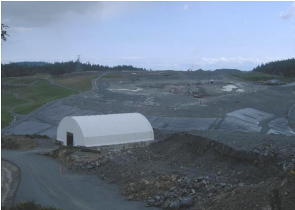
Figure 5-34. Hartland Landfill, looking southeast from the Hartland North site
