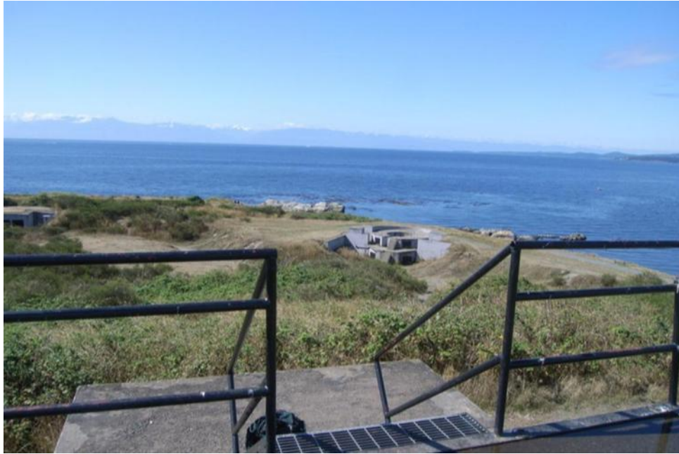
Figure 5-25. World War II military infrastructure on Macaulay Point
