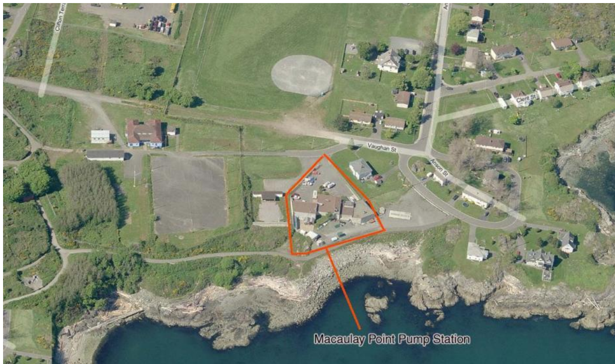
Figure 5-1. Oblique View of Macaulay Point Pump Station looking north
