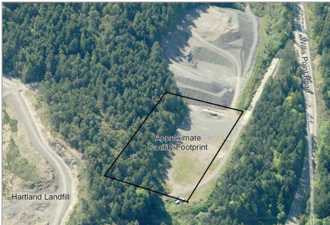
Figure 5-5. Aerial view of Hartland North site
