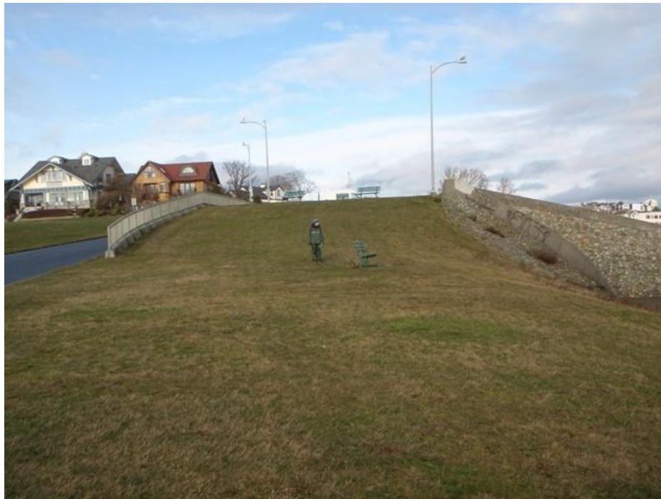
Figure 5-17. Looking north, immediately west of the existing Clover Point pump station
