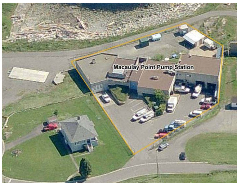
Figure 61 Macaulay Point Pump Station Oblique View (Looking South)
