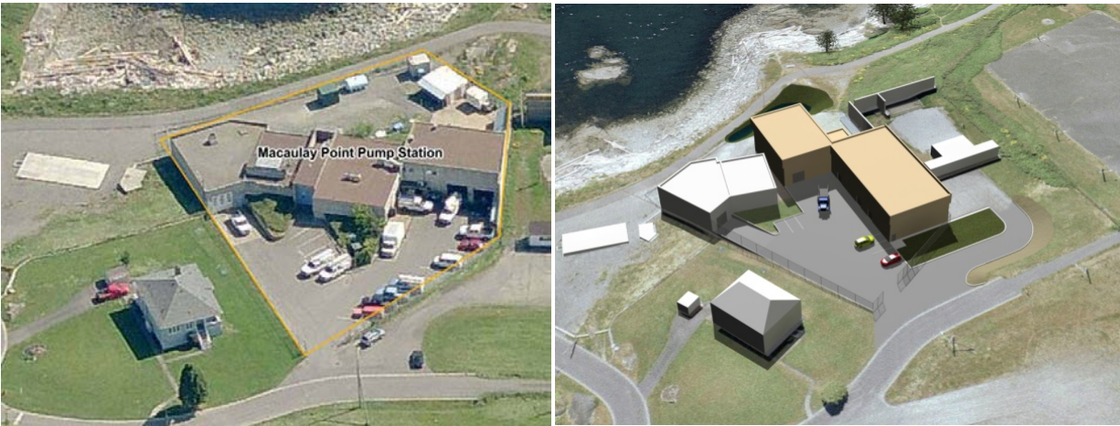
Figure 71 Aerial View of Macaulay Point before (Left) and After (Right) Upgrades
