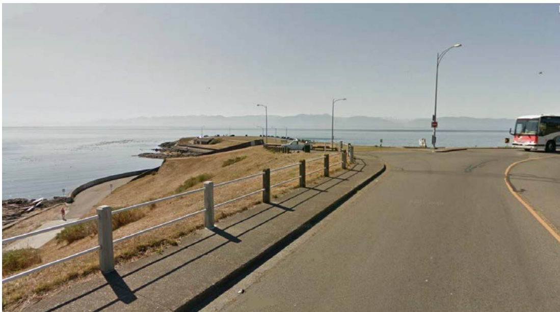
Figure 74 Clover Point Pump Station Looking South from Dallas Road
