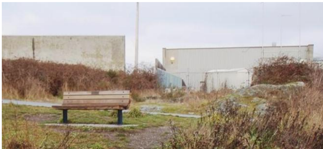
Figure 32 Southwestern Edge of the Macaulay Point Pump Station Between Existing Facility and Walkway. Note Bedrock Outcrop in Foreground
