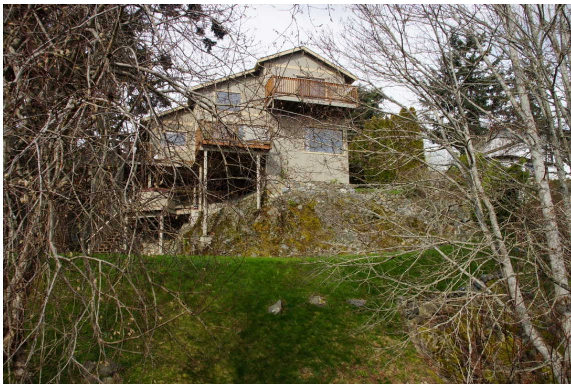
Figure 70 View of Residence to the West of the E&N Railway
