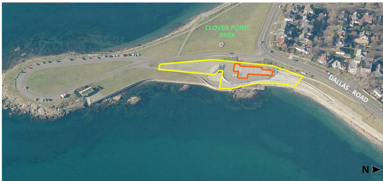
Figure 13 Oblique View of Clover Point Pump Station Looking West
