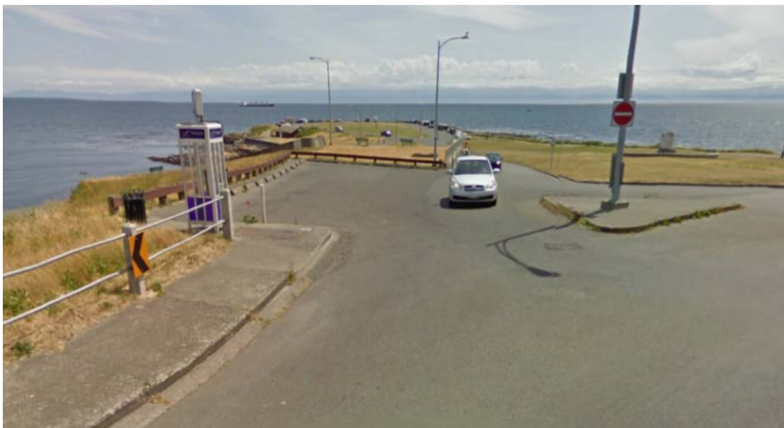
Figure 47 Looking South Over Existing Underground CRD Clover Point Pump Station from Dallas Road and Clover Point Road Intersection
