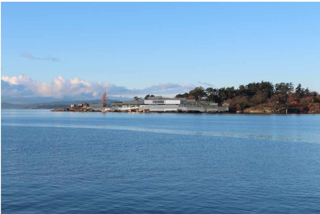
Figure 81 Rendered View of the McLoughlin Point Site with the Proposed Wastewater Treatment Facility Superimposed
