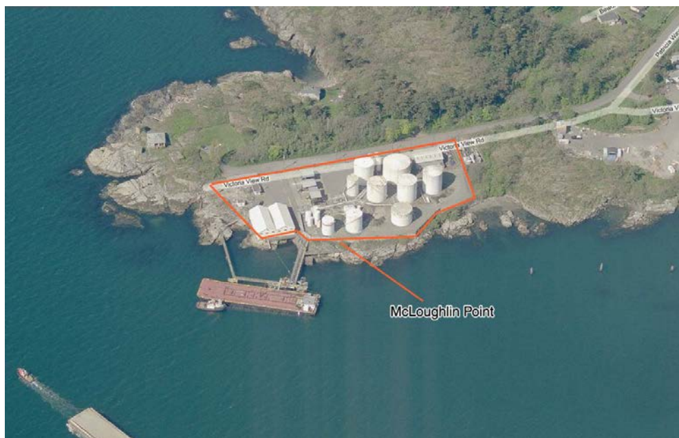
Figure 64 McLoughlin Point Site before Fuel Tank Decommissioning in 2008 (Looking West)
