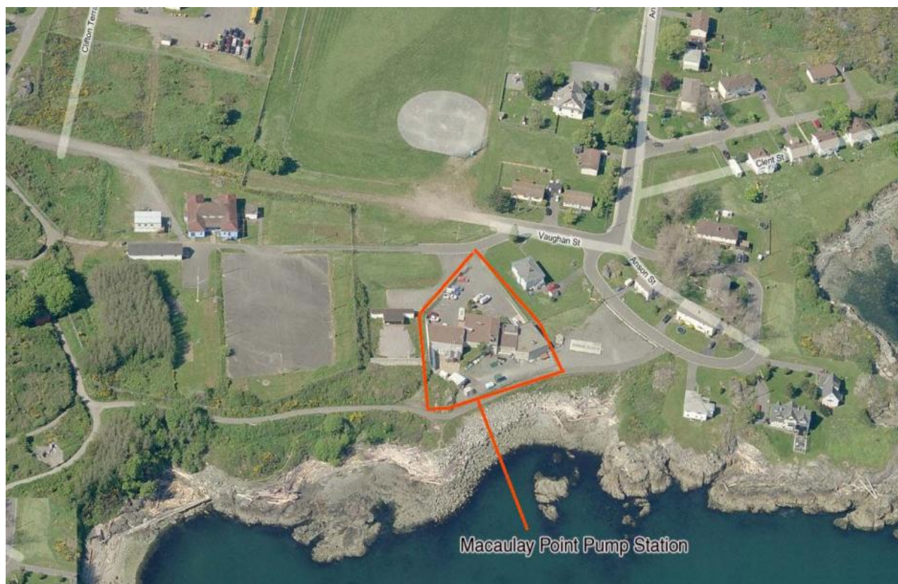
Figure 11 Oblique View of Macaulay Point Pump Station Looking North
