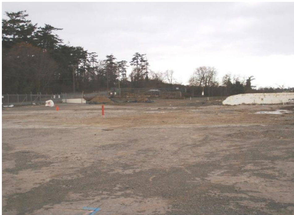
Figure 38 McLoughlin Point Property, Looking North. Asphalt Pad and Concrete Slab Capping in Foreground
