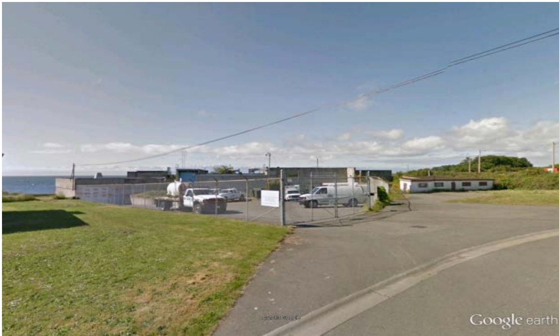
Figure 72 View of Macaulay Point Pump Station Looking South from Vaughan Street
