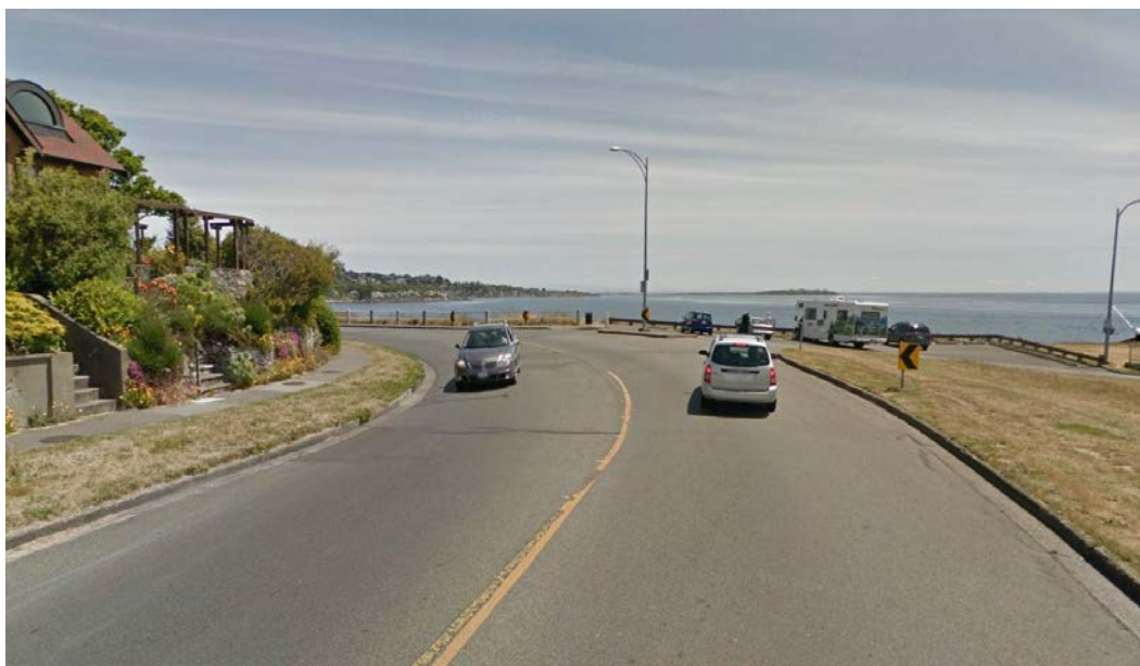
Figure 76 Clover Point Pump Station Looking East from Dallas Road
