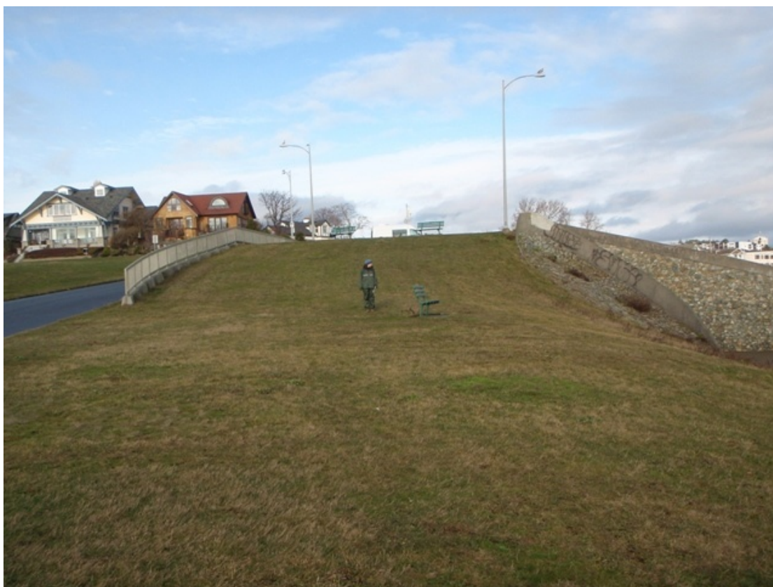
Figure 36 Facility Expansion Area, Looking North, Immediately West of the Existing Clover Point Pump Station
