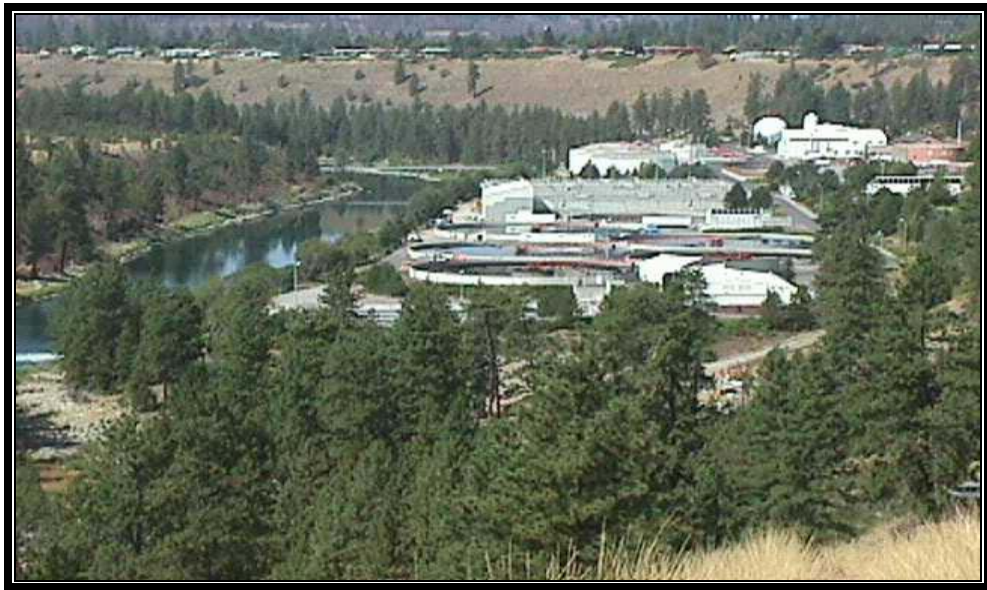
Photo C-1 Spokane Wastewater Treatment Plant, Washington.
