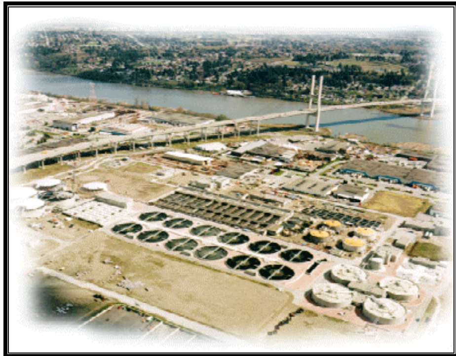
Photo C-2 Annacis Island Wastewater Treatment Plant, Greater Vancouver Regional District.
