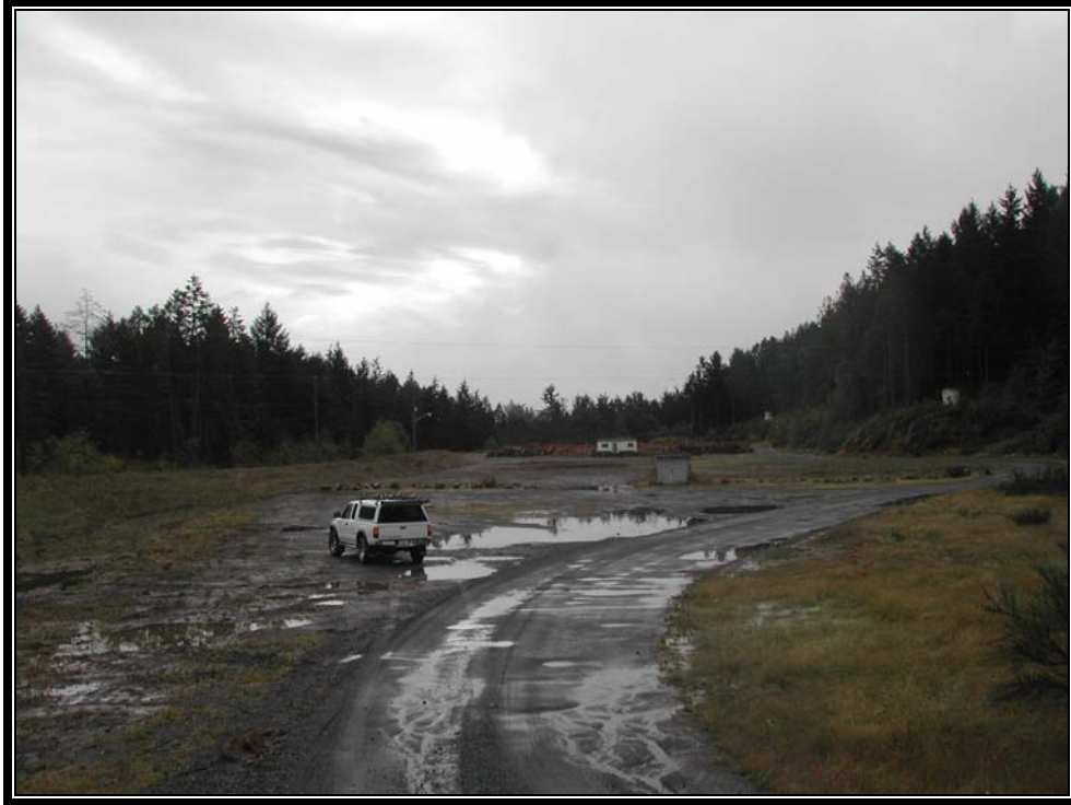
Photo 5-3 The disturbed area at the northern end of the Hartland site. The area in the background will house the administration, wastewater treatment and garage facilities.
