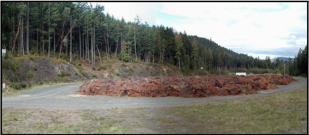
Photo 5-11 This cleared and levelled portion of the Hartland site would house administration, wastewater treatment, and garage structures. The CRD proposes to store gravel on most of the site. Treed buffers would be retained around this pad.
