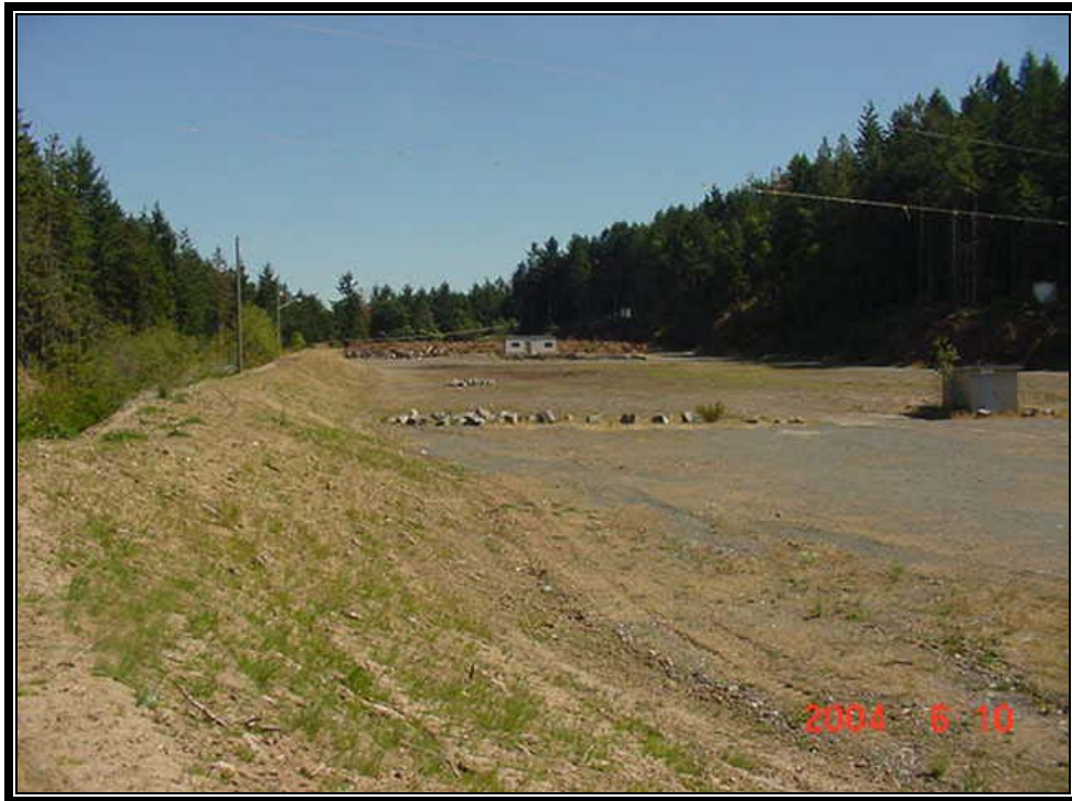
Photo 3-13 Hartland site at lower bench looking east to proposed digester site.
