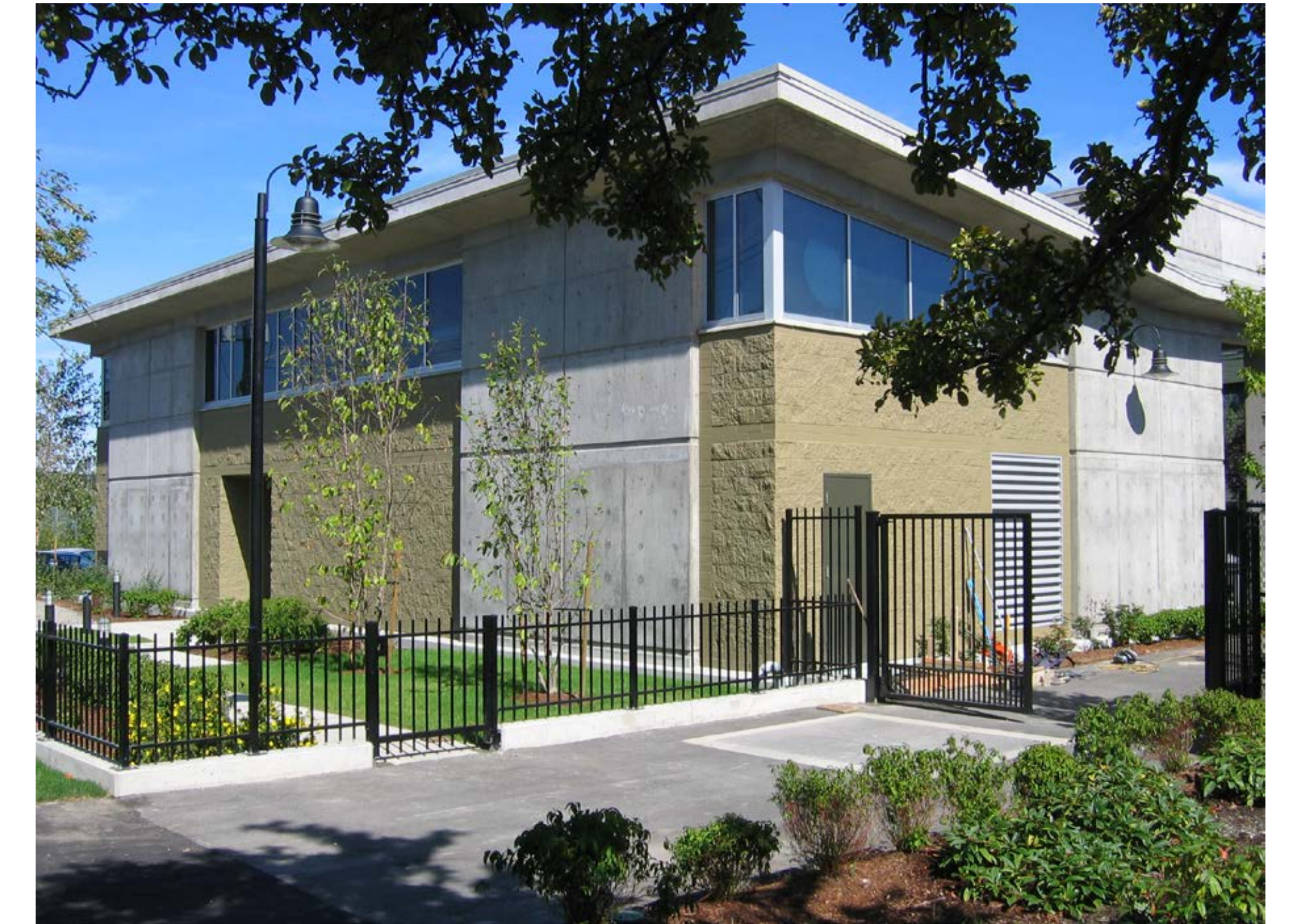
>> Trent Pump Station
