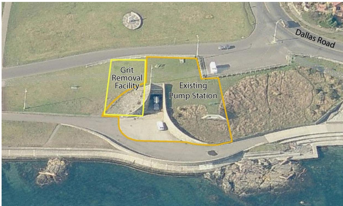
Figure 5-3. Oblique view of Clover Point Pump Station access looking west
