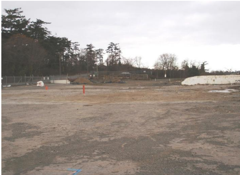
Figure 5-19. McLoughlin Point property, looking north. Asphalt pad and concrete slab capping in foreground.
