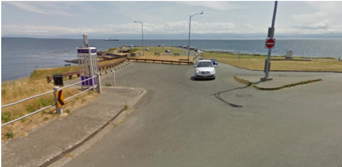
Figure 5-29. Looking south over existing underground CRD pump station from Clover Point site at Dallas Road and Clover Point Road intersection
