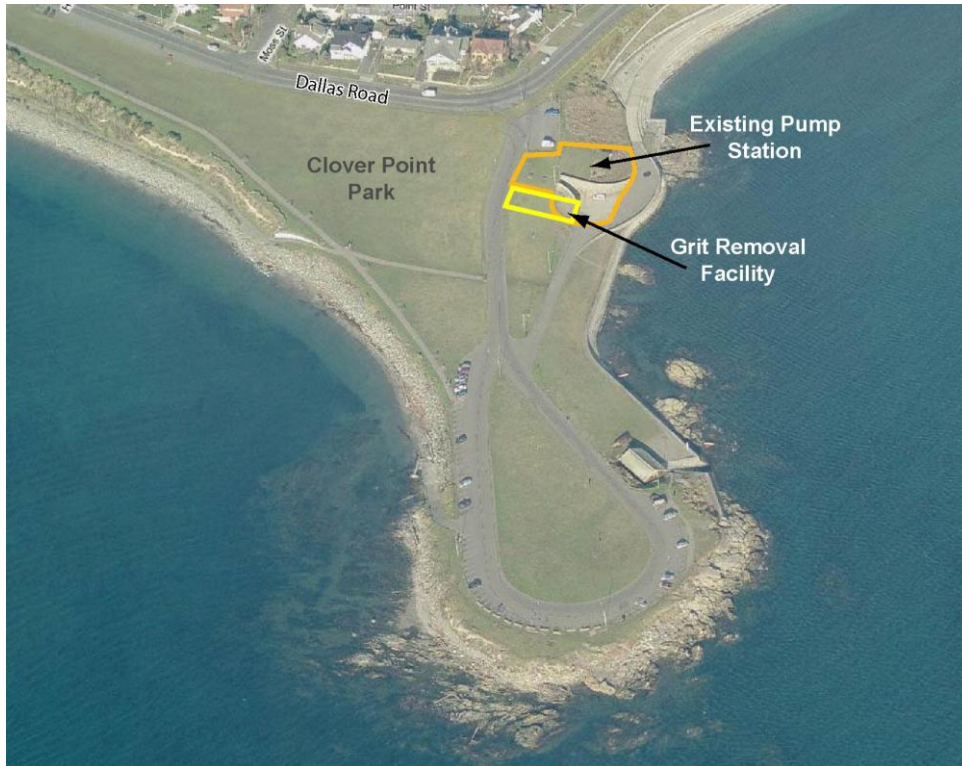
Figure 5-2. Oblique view of Clover Point Pump Station looking north
