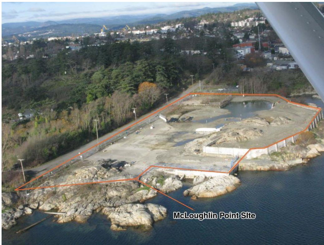
Figure 5-4. McLoughlin Point site from south
