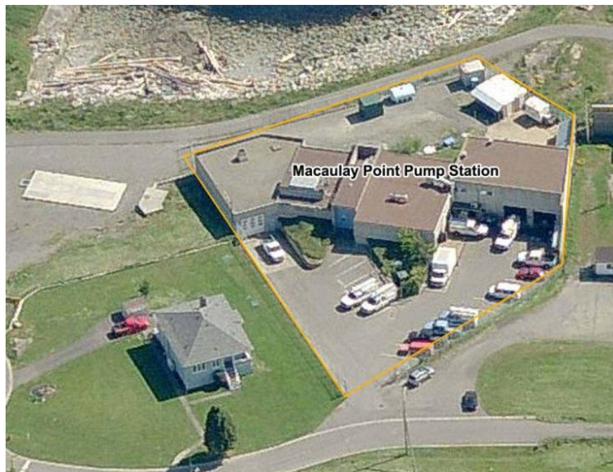
Figure 5-38. Macaulay Point Pump Station oblique view looking south
