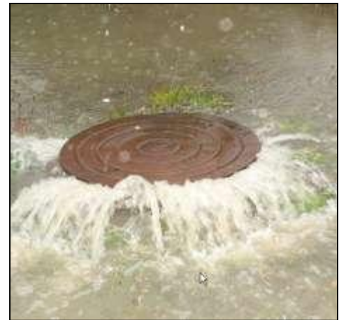
A sewer overflow from a surcharging manhole.
