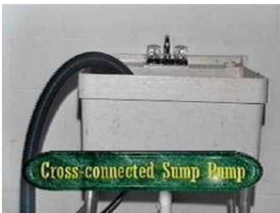
Figures 7.5 and 7.6: Examples of Sump Pump Cross Connections
