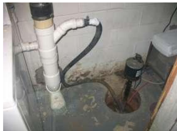
Figures 7.5 and 7.6: Examples of Sump Pump Cross Connections
