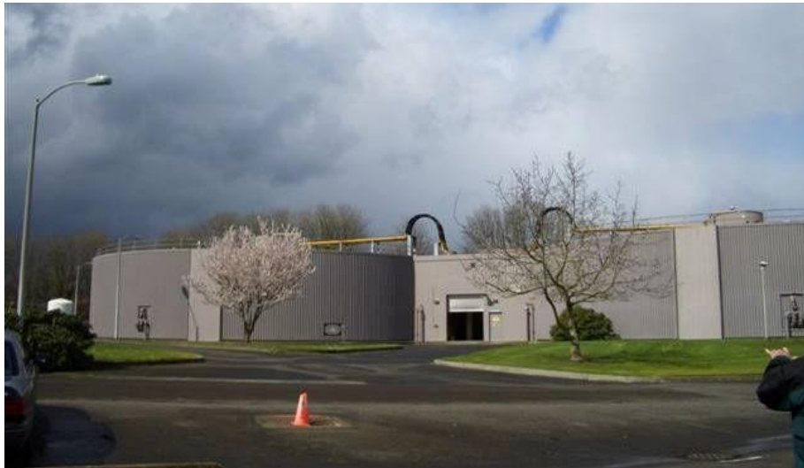
Figure 5.2 – Mesophilic Anaerobic Digesters: Columbia Boulevard WWTP, Portland, Oregon
