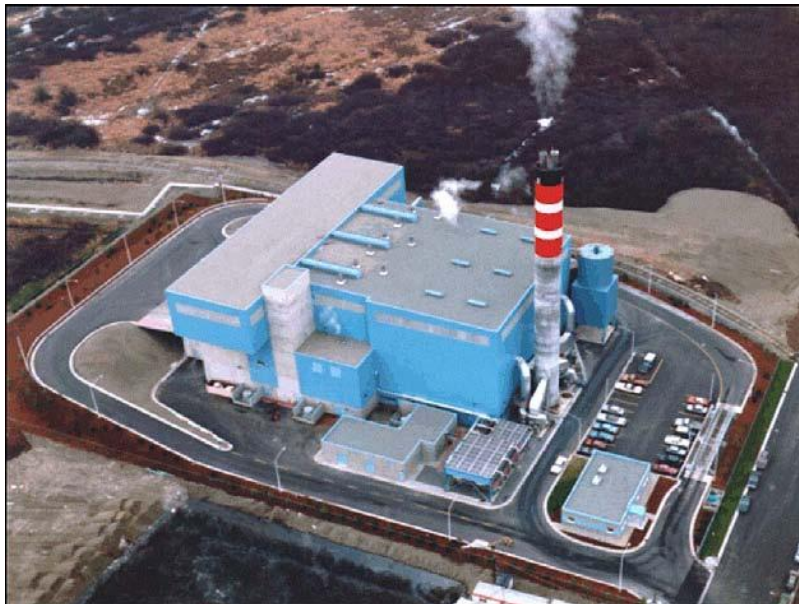
Figure 3.17 – Burnaby Mass Burn WTE Facility
