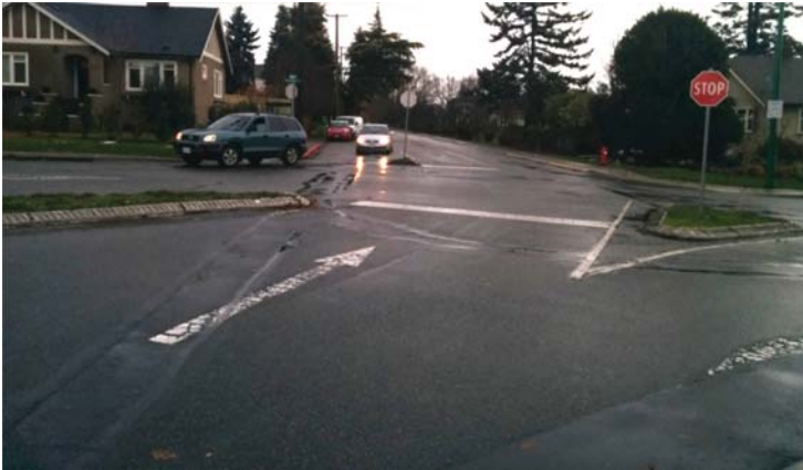
▲ Looking east through the intersection of Cadboro Bay Rd., Thompson Ave., and Nottingham Rd.
