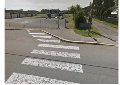
Figure 7- Crosswalk on Henry Ave does not align with the fence entrance to the school.
