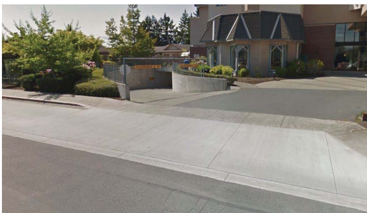
Figure 10- Shoal Centre underground parking lot entrance/exit. The angle of the entrance/exit makes it difficult for drivers to see pedestrians.
