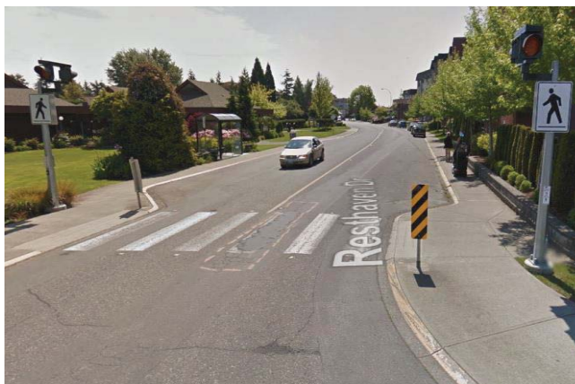
Figure 9- Enhanced crosswalk at Resthaven Dr. and Mills Rd. with extended curbs.
