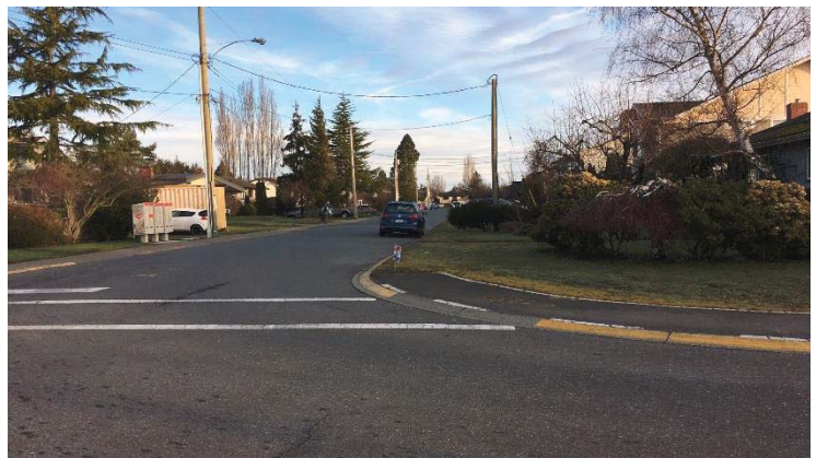
Figure 6- The abrupt ending to the Henry Ave. bike path at Siddall Rd. This path does not have a let down, nor does it indicate where cyclists should go.
