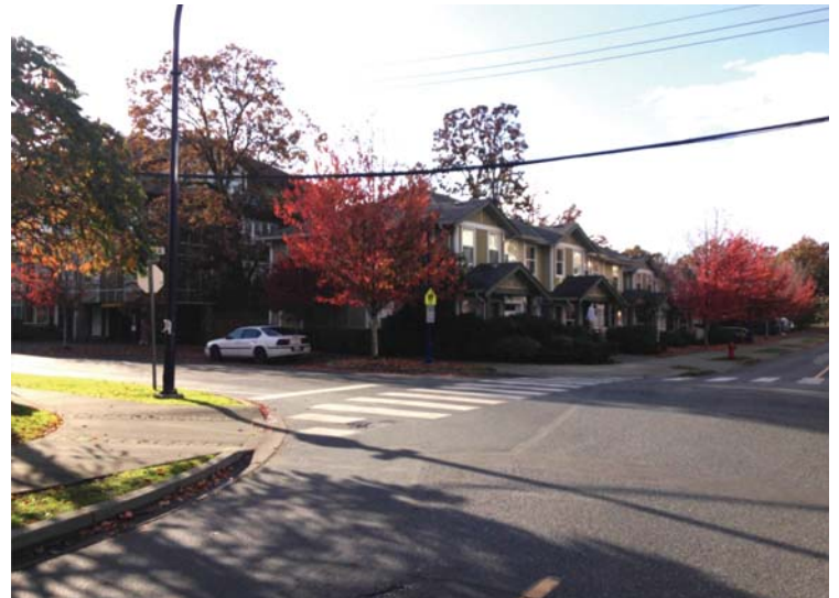
▲ Wide curb returns at the intersection of Jacklin Rd. and Brock Ave.
