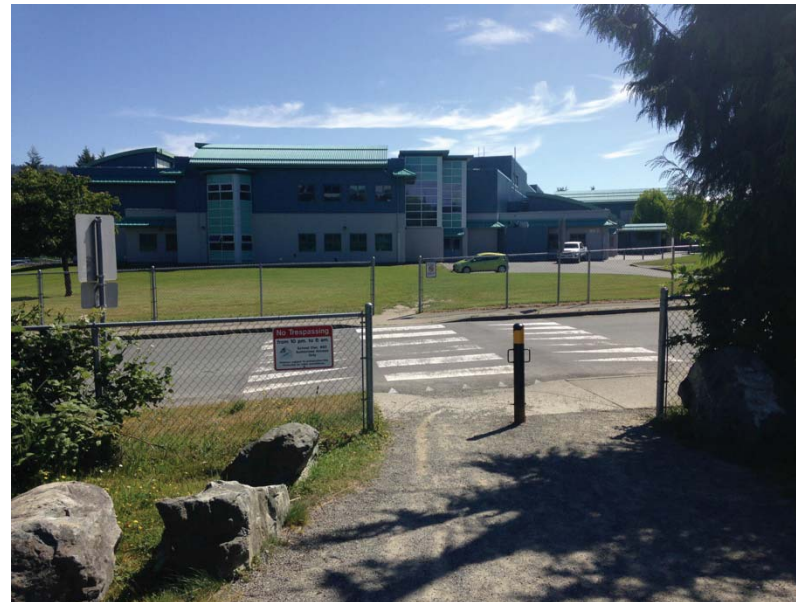
▲ A raised crosswalk provides the only traffic calming on Journey School Ln.
