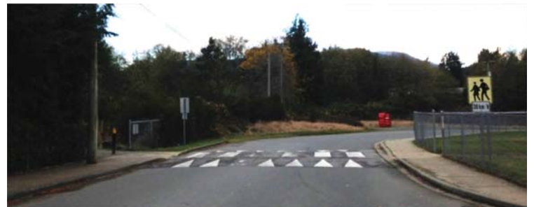
▲ Looking north towards the raised crosswalk on Journey School Ln.
