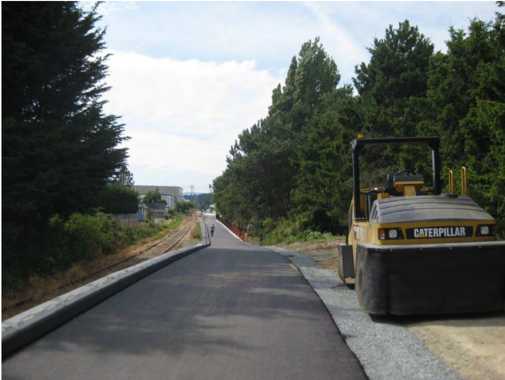
Paving a section of the E&N Rail Trail.
