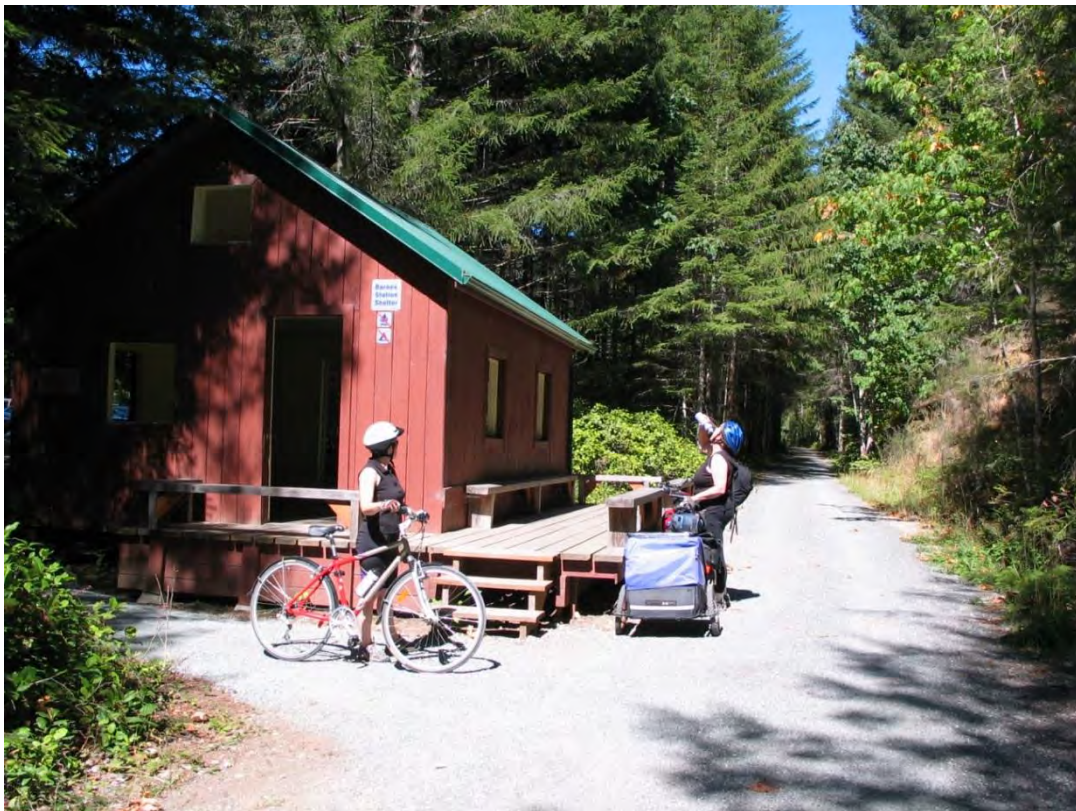
Barnes Station rest-stop at Sooke Potholes Regional Park along the Galloping Goose Regional Trail.
