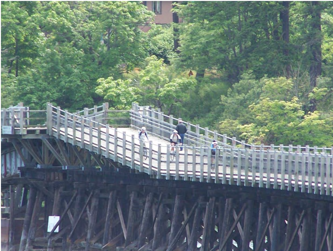
Travelling on the Selkirk Trestle, Galloping Goose Regional Trail. Photo by John Luton.
