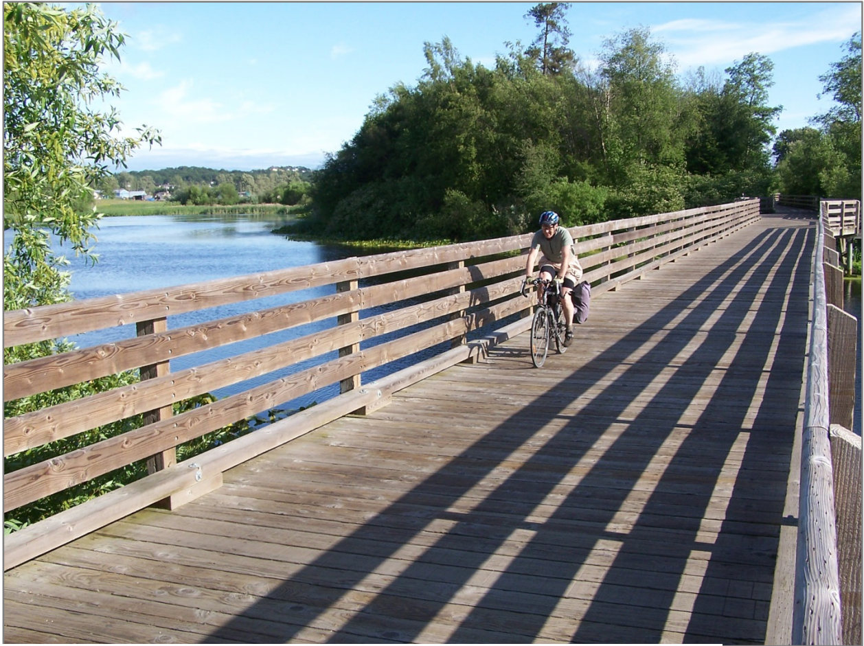
Saanich's Blenkinsop Trestle, Lochside Regional Trail Photo: John Luton
