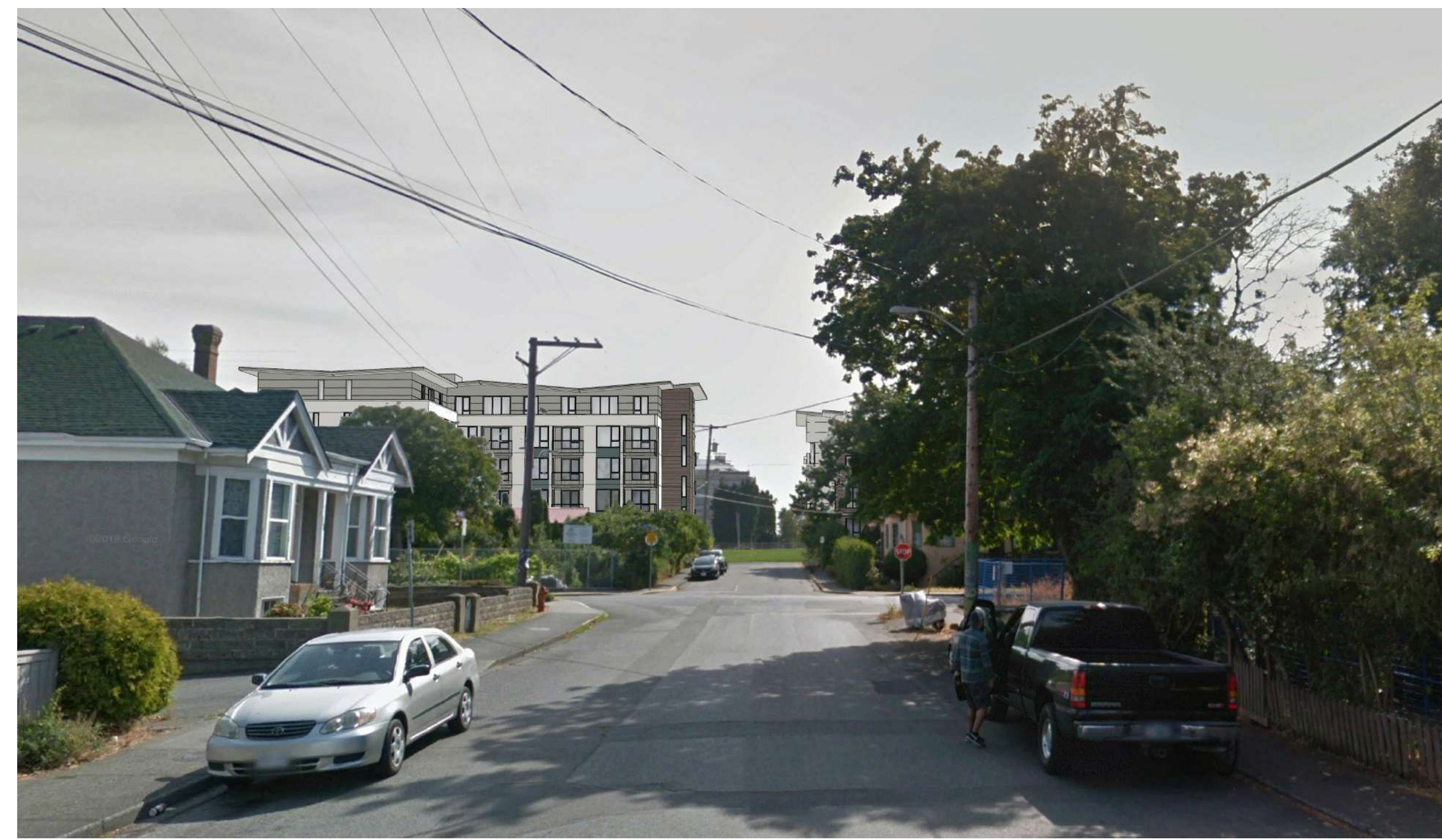
AFTER LOOKING EAST - FROM NORTH PARK ST.
