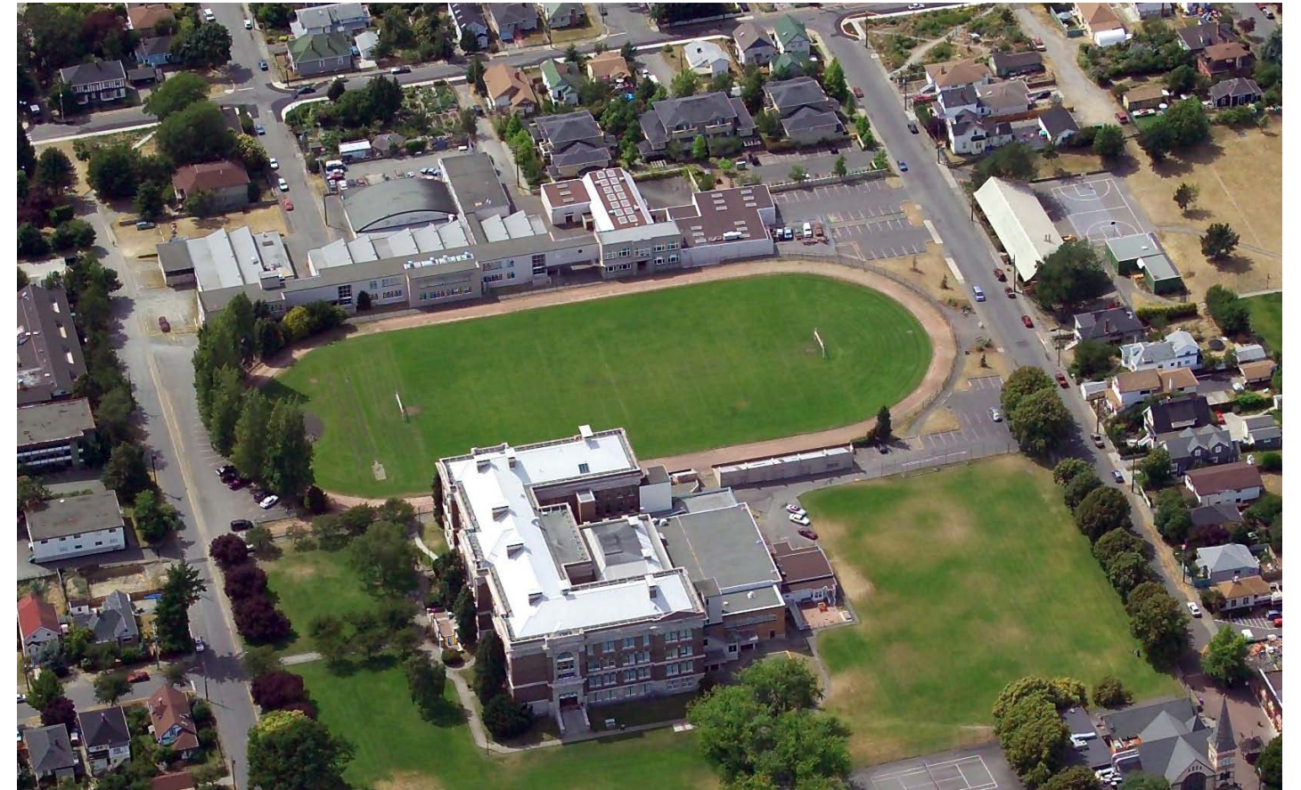
Aerial View (prior to demolition)
