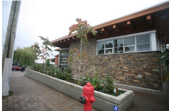
Figure 1 Planter irrigated by roof water collected in underground detention tanks.
