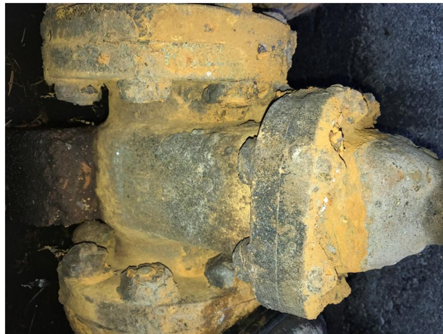
Photograph #10 – Side View: 150 mm Low Level Outlet Control Valve, flanges, nuts & bolts
